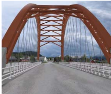
Fig. 5: Steien bridge from the driver's view
