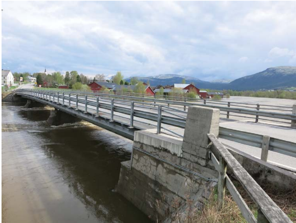
Fig. 1 The existing Steien bridge
