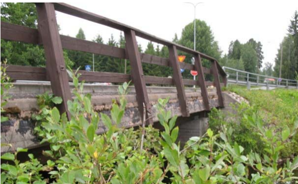
Fig. 13. Kruununmylly Bridge in 2013.
