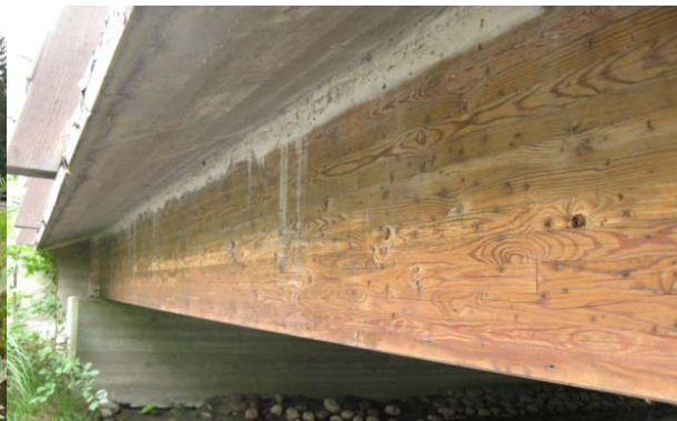
Fig. 14. Outer surface of the glulam beam.
