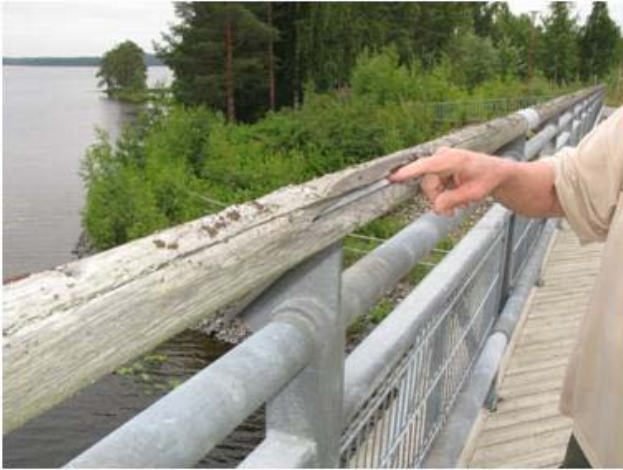
Fig. 16. Worn top guide of the railing. On the background wildy growing bushes are seen.
