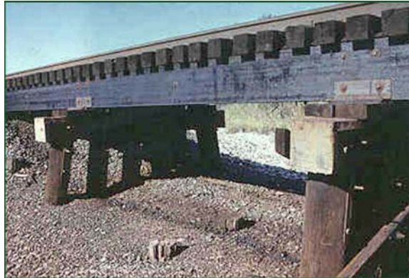
Rehabilitated bridge using glued-laminated stringers.
