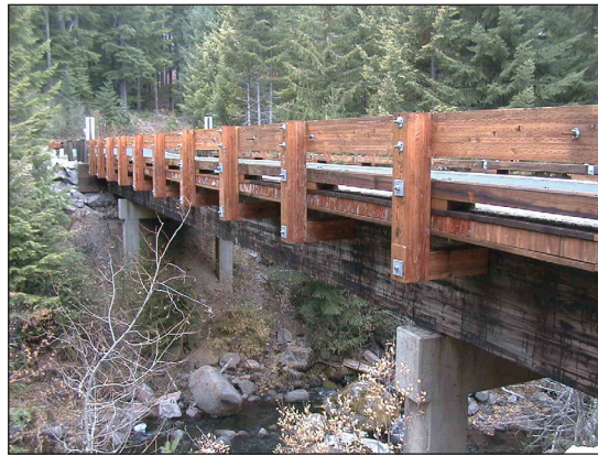
Modern timber bridge on a county highway.
