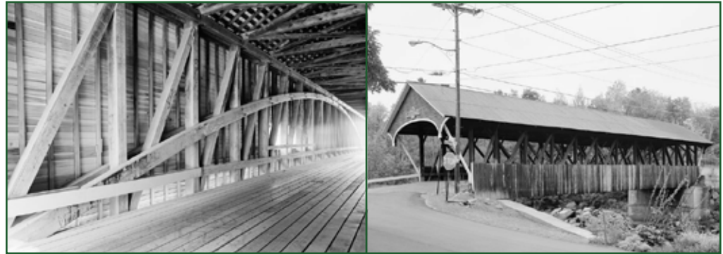
Figure 1. Arch truss and long truss covered bridges
