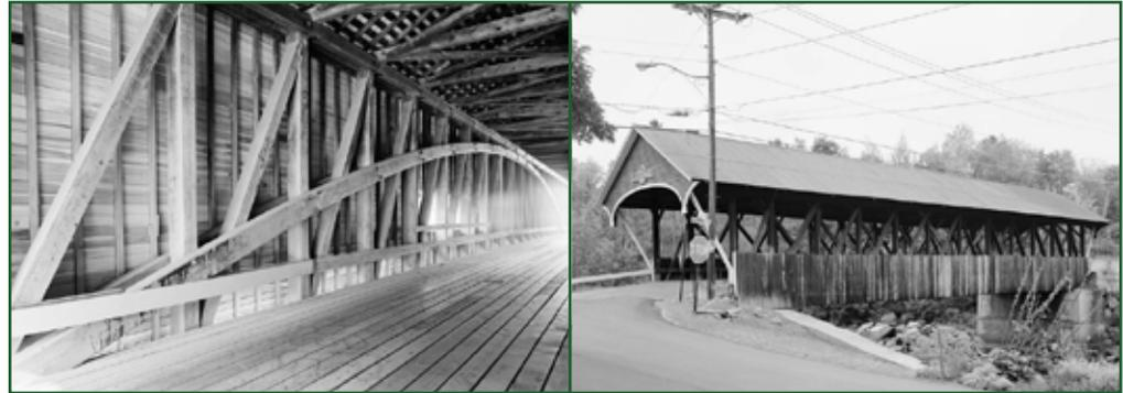
Figure 1. Arch truss and long truss covered bridges
