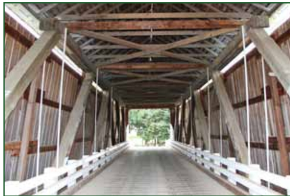
Gallon House Covered Bridge located at Silverton, Oregon, is a Howe Truss design.
