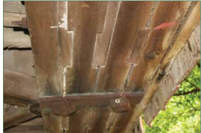
Figure 3—Bottom chord connection detail.
