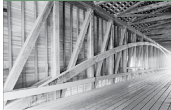
Figure 1—Burr Arch covered bridge.
