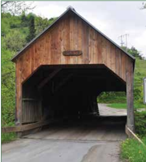
Figure 2— Phase I Queen Post Truss in Flint, Vermont.
