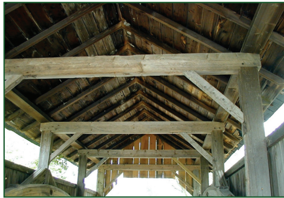
In covered bridges, naturally durable wood species are an attractive option for replacement components that are protected from moisture
