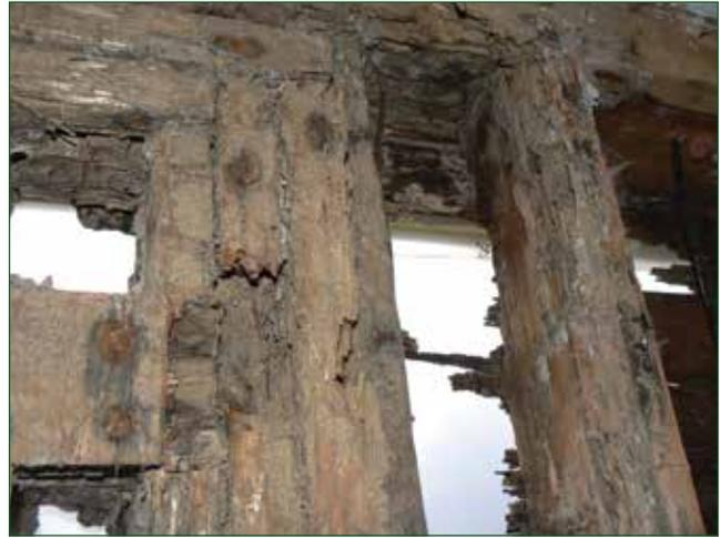
**Termite damage to an existing structural bridge member.**
