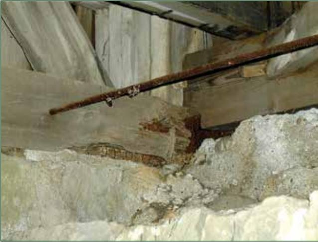
**Cubicle brown-rot decay and termite damage to the support members masonry contact under covered bridge.**
