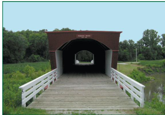
Roseman Bridge, Madison County, Iowa.
