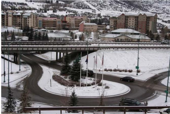
Figure 6.4 Teardrop Roundabout on the I-70 exit ramp to Avon, CO (Isebrands)
