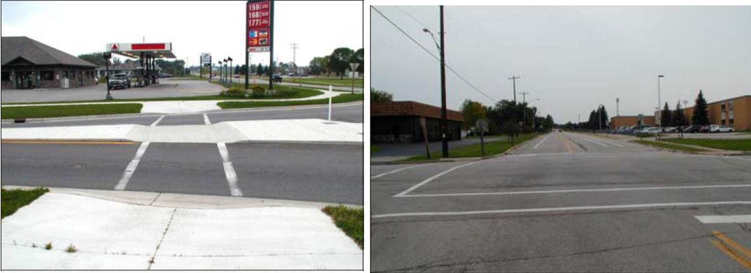
Figure 6.2 Pedestrian crossing accommodations at the Lineville/Cardinal Roundabout compared (left) to a regular intersection (right) (Brown County, WI)
