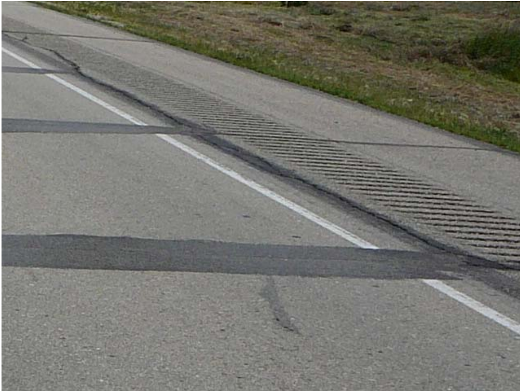
Figure 4.7. Rolled rumble strips
