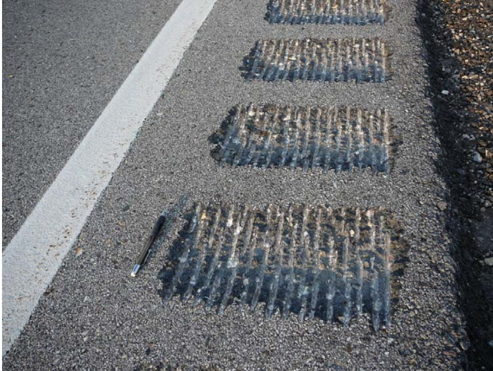
Figure 4.8. Milled rumble strips
