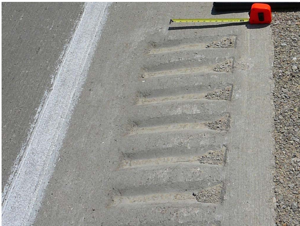
Figure 4.9. Formed rumble strips
