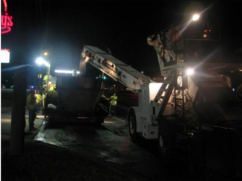
**Figure 4.5. Surface milling in Florida using stationary and equipment-mounted lighting**
