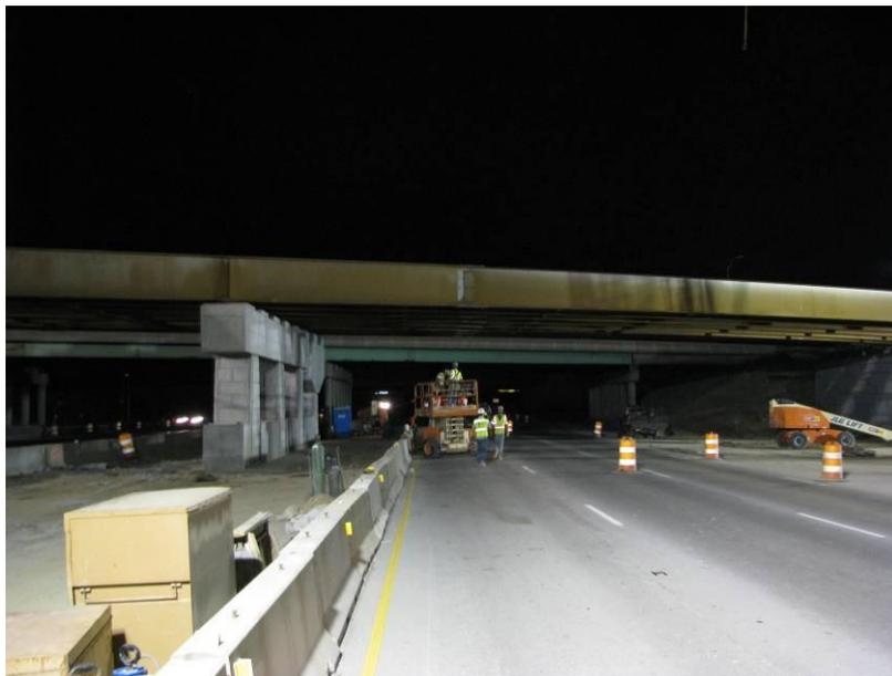
***Figure 4.7. Construction workers performing bridge deck tie placement in Indiana***
