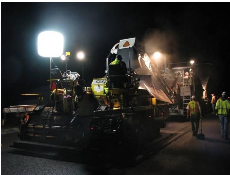
**Figure 4.4. Mainline paving on SB I-55 using equipment-mounted balloon lighting**
