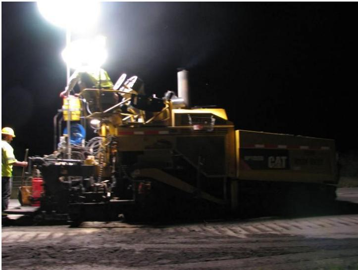
**Figure 4.3. Milling and paving on SR 10 and I-66 using equipment-mounted balloon lighting**
