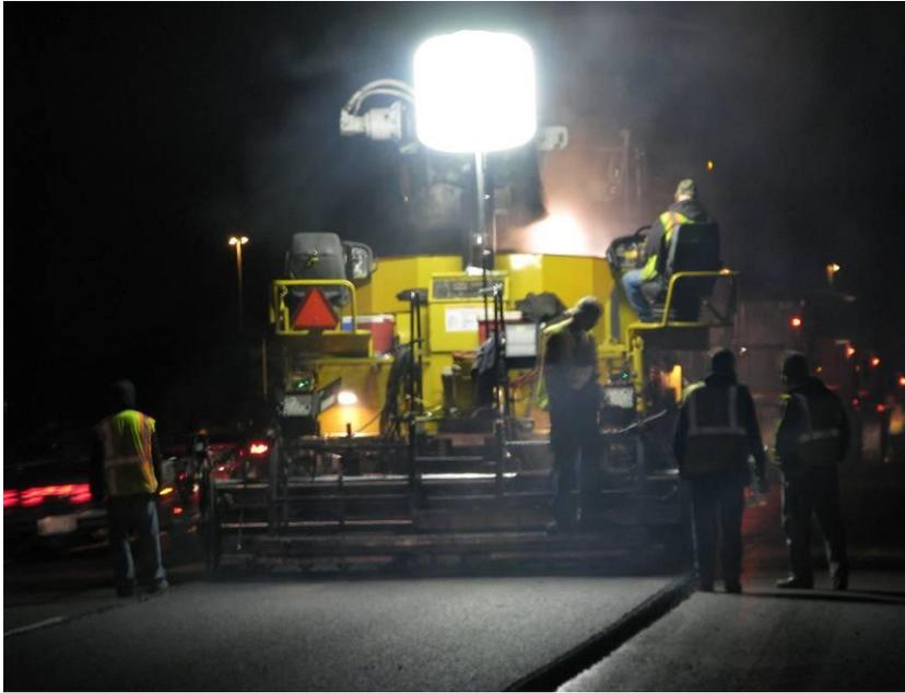
**Figure 4.8. Workers on I-290 performing surface milling and paving in Illinois**
