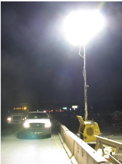
***Figure 4.2. Portable stationary lighting in use on I-465 bridge deck replacement in Indiana***
