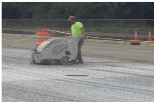
**Figure 7. A typical early entry saw-cutting process**
