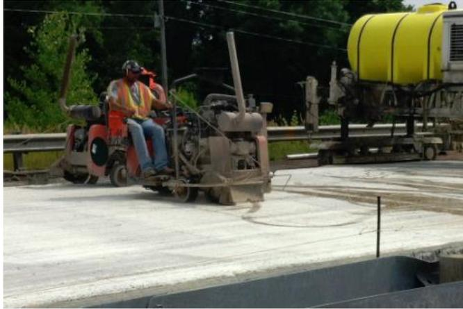
**Figure 8. A typical conventional saw-cutting process**
