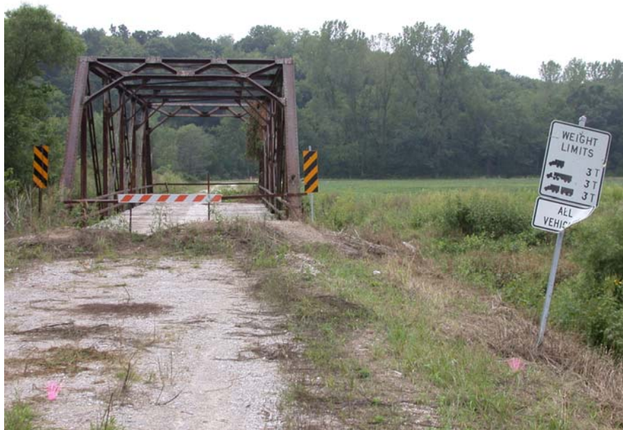
Figure 1.1. Wapello County truss bridge prior to replacement.
