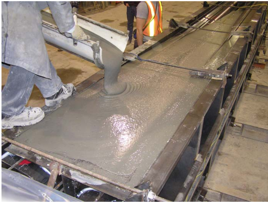
Figure 3.4. Placement of concrete during construction of Wapello County UHPC bridge beams.
