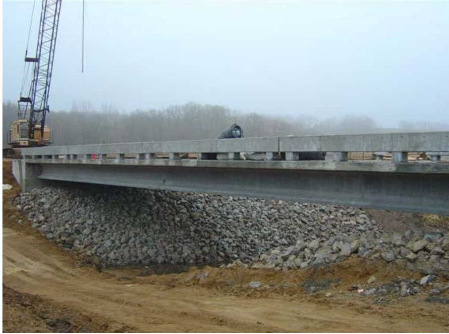
Figure 3.5. Elevation of Wapello County UHPC bridge.
