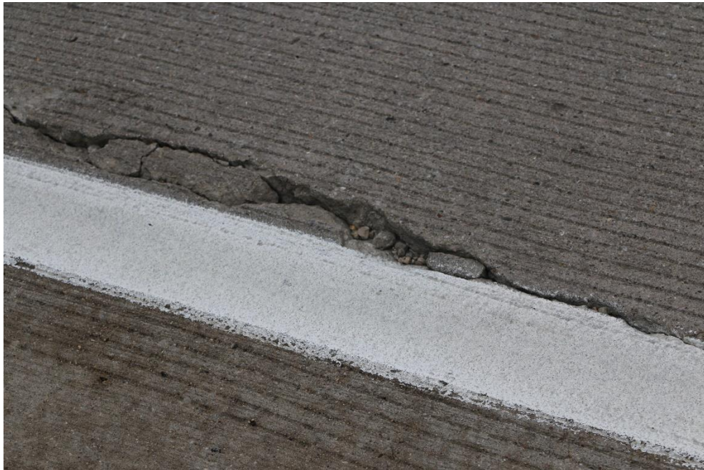
Figure 77. Longitudinal cracks at Site 5
