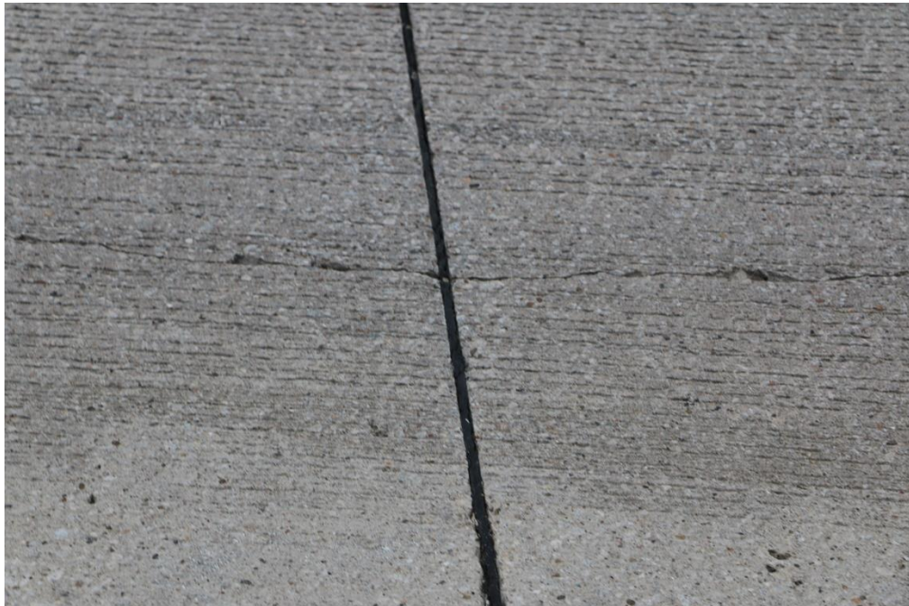
Figure 67. Transverse (top) and longitudinal (bottom) cracks at Site 3
