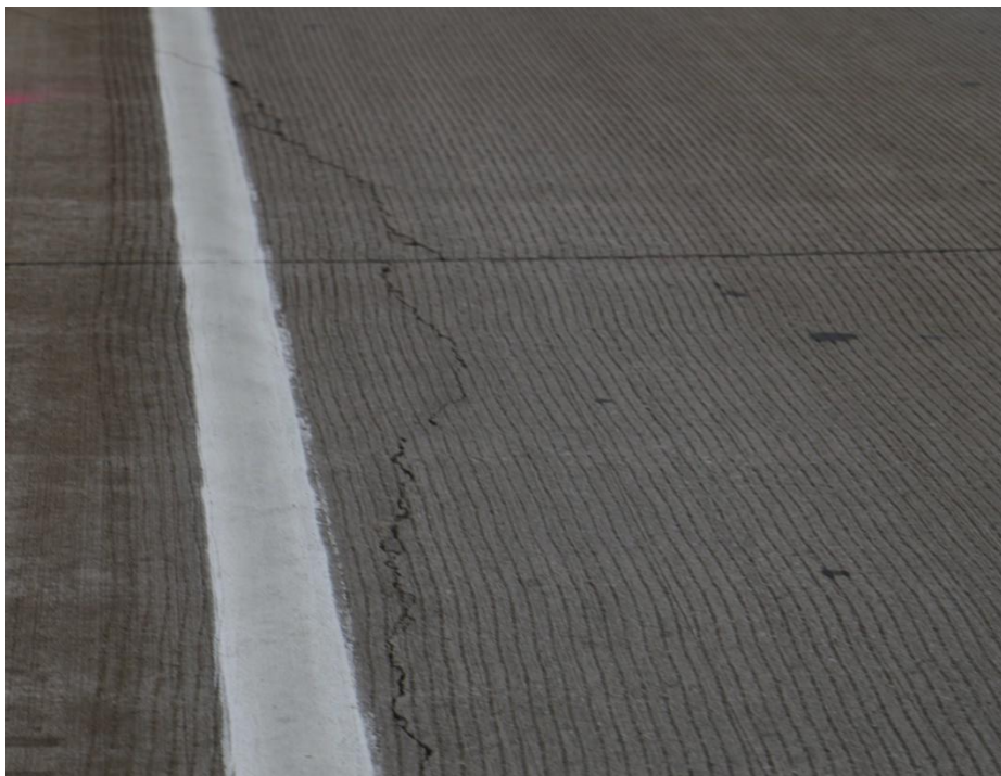
Figure 76. Slabs with cracks observed at Site 5
