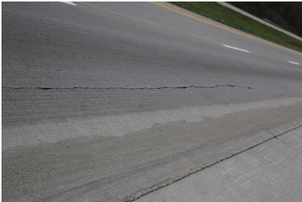
Figure 66. Slabs with cracks observed at Site 3
