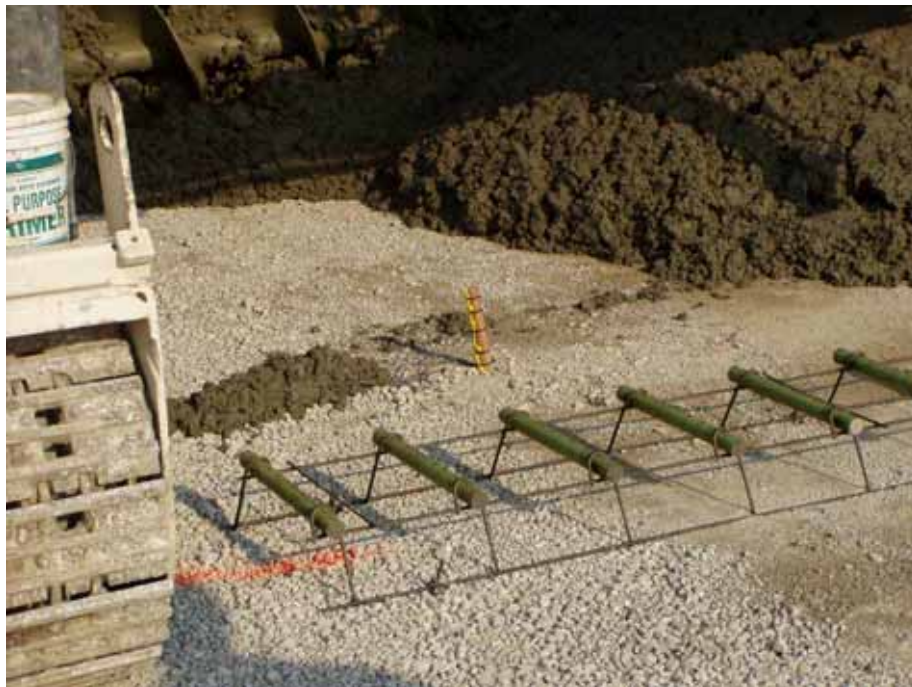
Figure G.8. Temperature instrumentation
