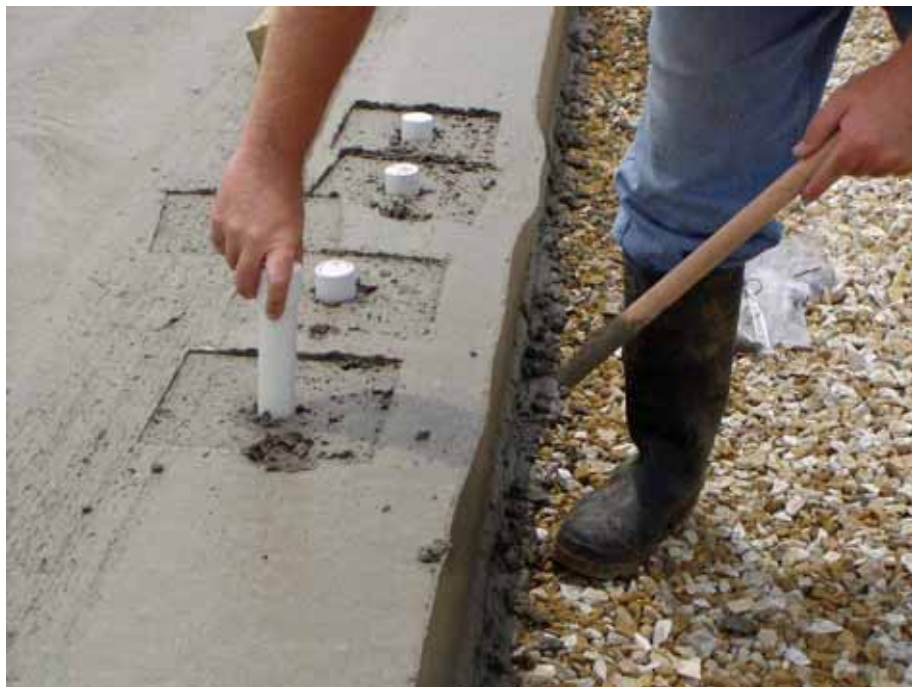
Figure D.10. Relative humidity instrumentation installation following AVA sampling
