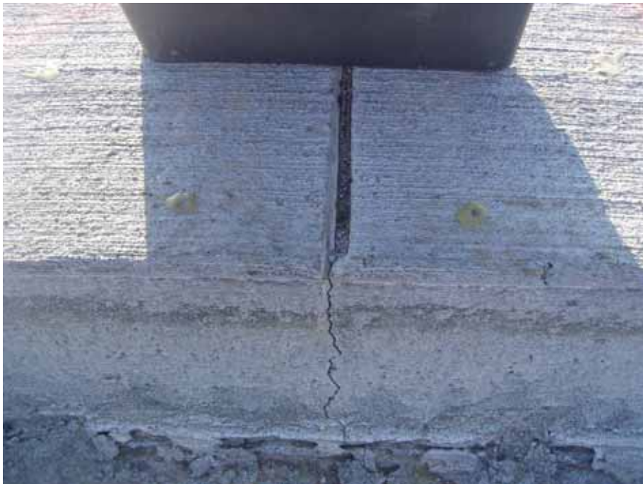
Figure D.16. Transverse joint DEMEC location in morning (visible crack)
