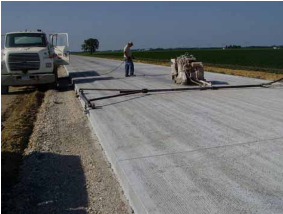
Figure. D.4. Longitudinal sawcut operations
