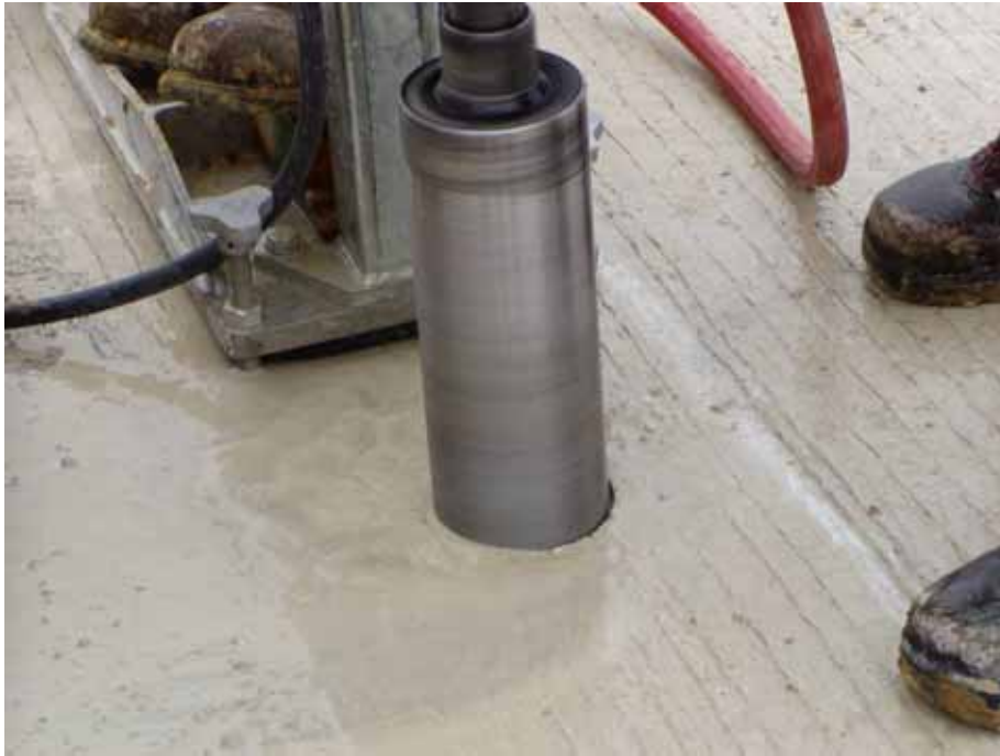
Figure A.21. Pavement coring
