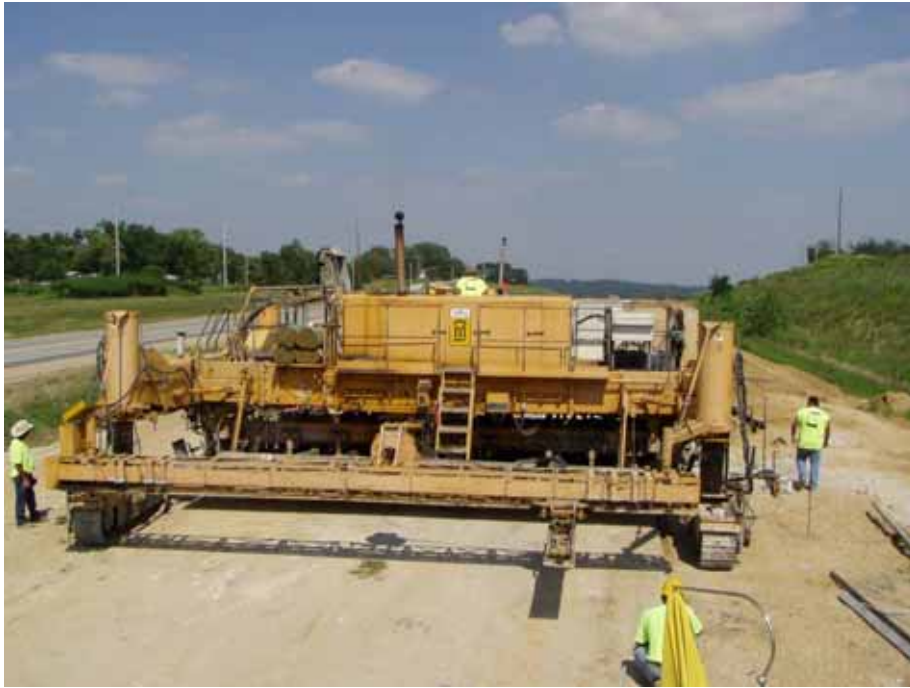
Figure G.1. Slipform paver
