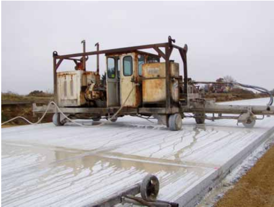
Figure A.9. Transverse sawcut operations
