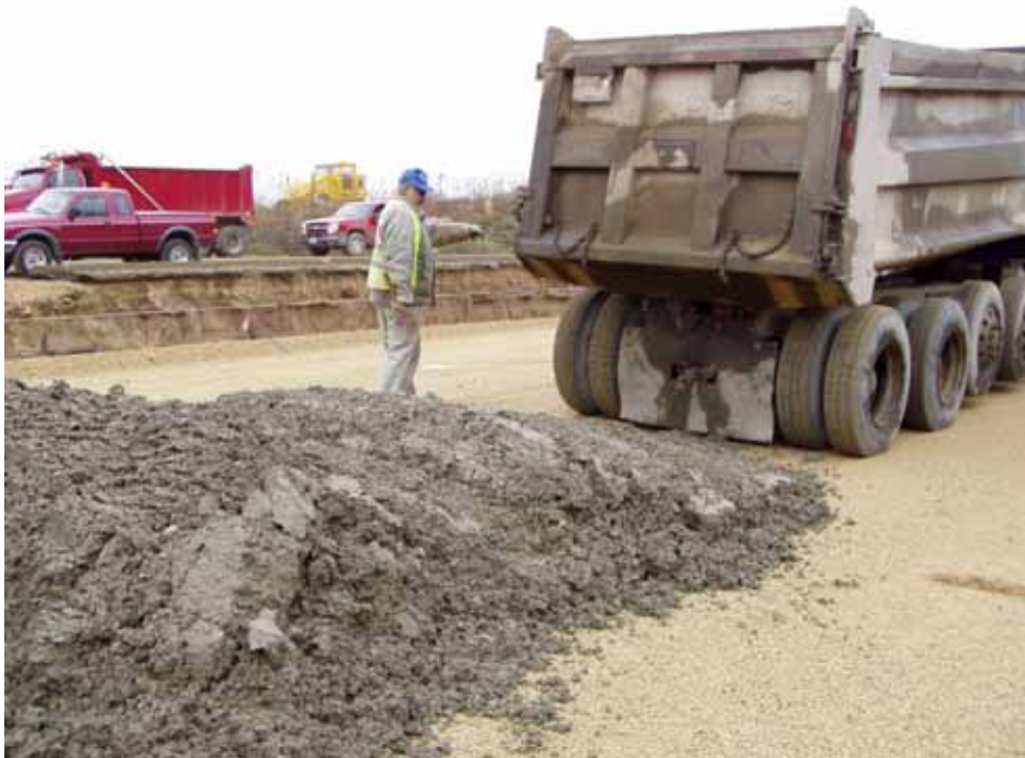
Figure A.2. Concrete delivery operations
