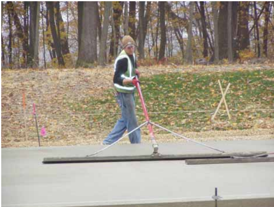
Figure A.6. Straightedge operations
