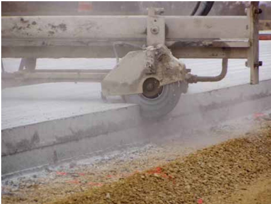
Figure A.10. Transverse sawcut operations
