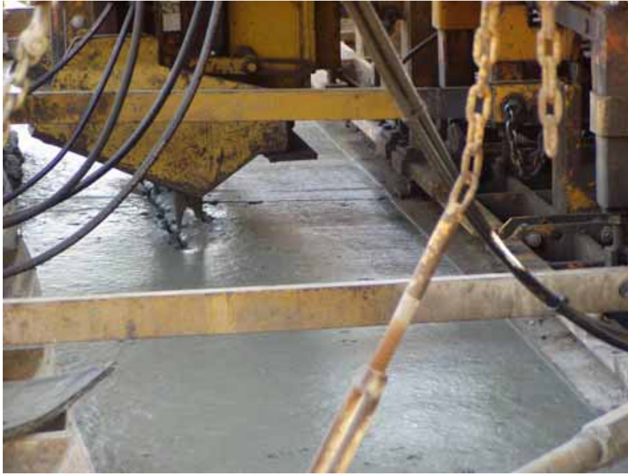
Figure G.3. Tie bar insertion operations
