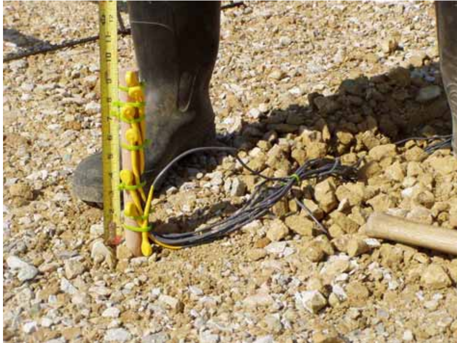
Figure D.7. Temperature instrumentation installation
