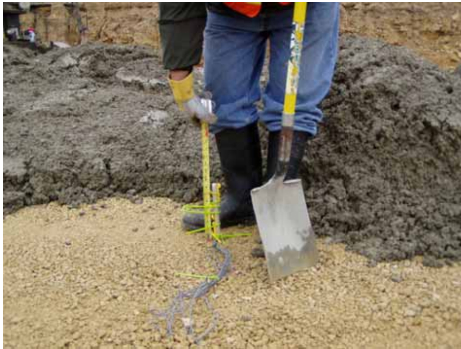
Figure A.15. Temperature instrumentation installation
