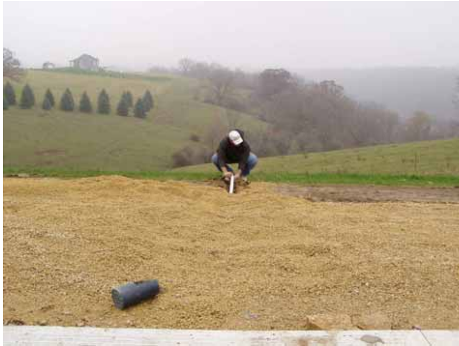
Figure A.17. Temperature instrumentation installation
