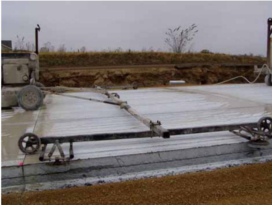
Figure A.11. Longitudinal sawcut operations
