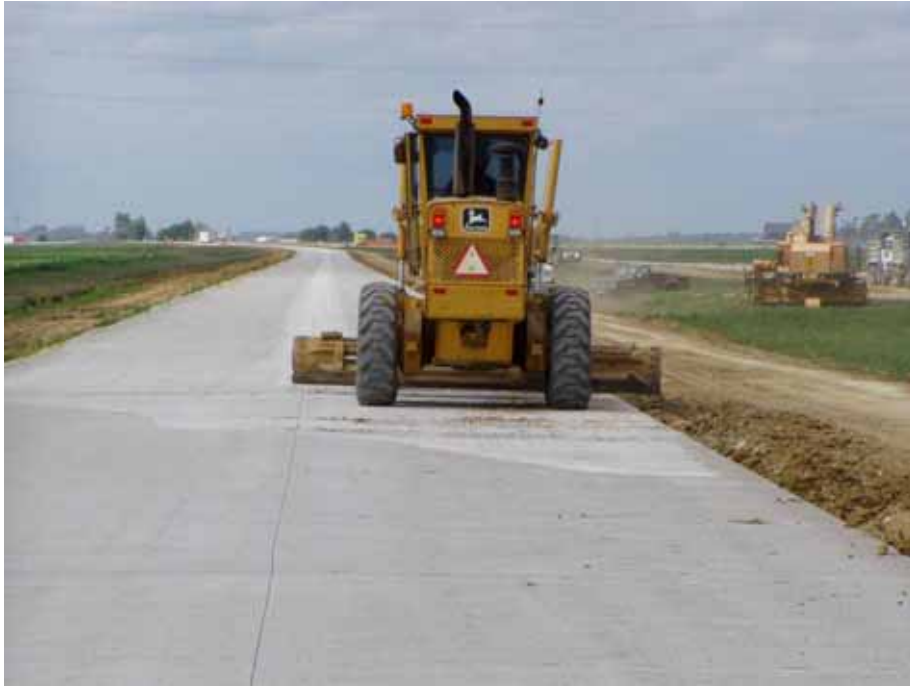
Figure D.5. Motor grader operations prior to acceptance profile measurements
