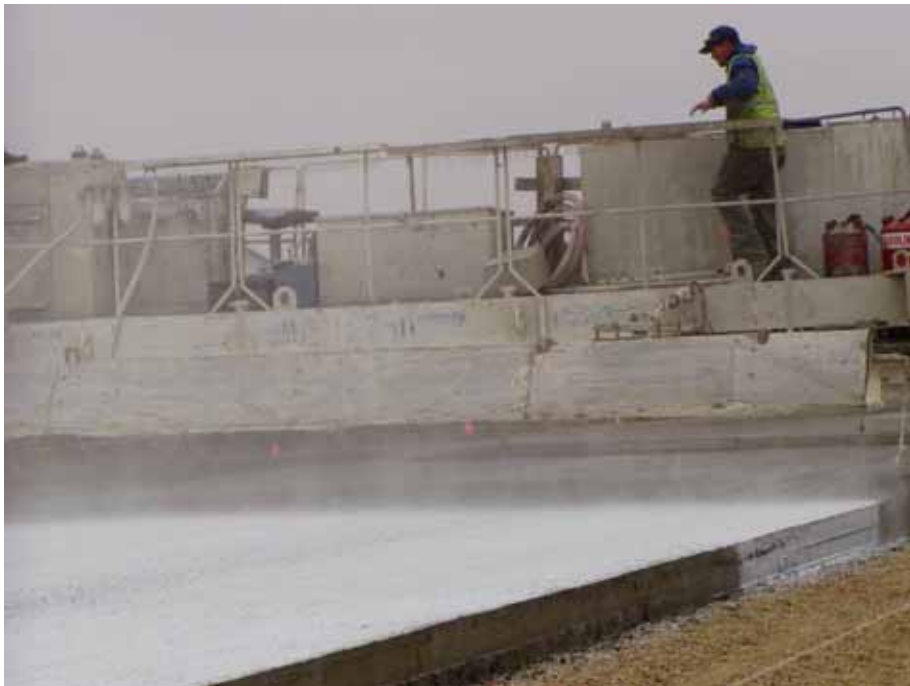
Figure A.8. Curing operations
