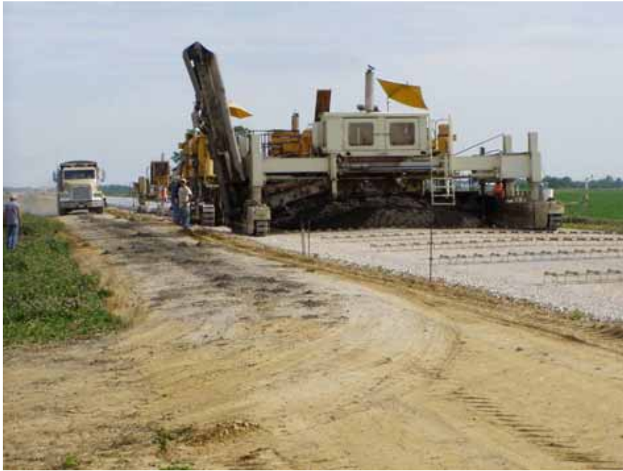
Figure D.1. Concrete delivery and paving operation
