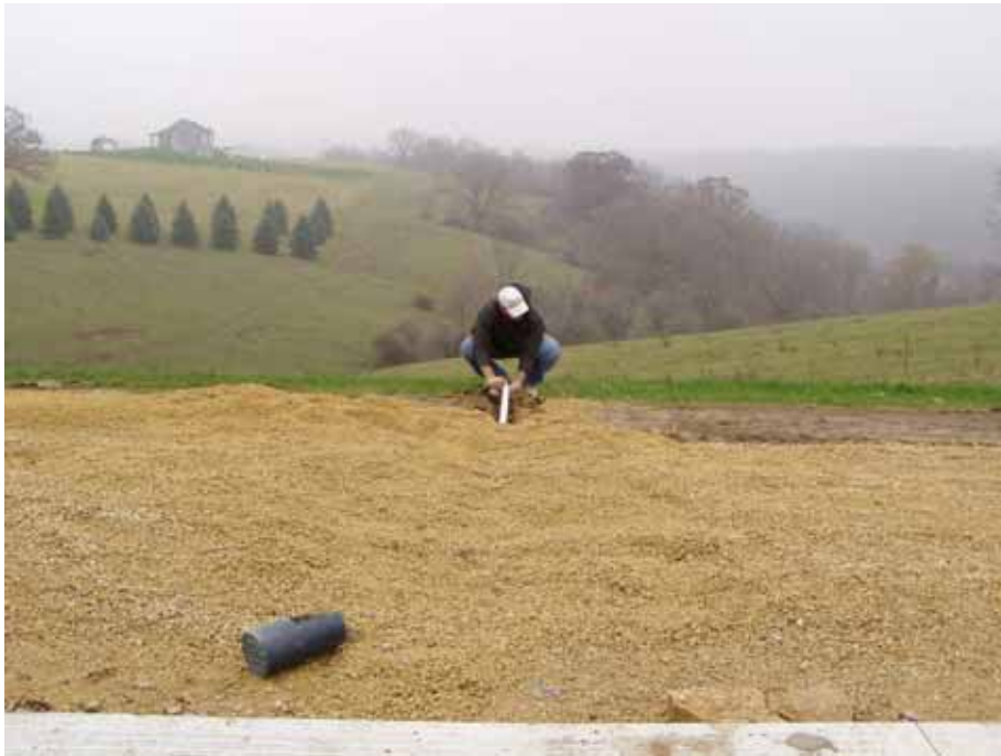
Figure 19. Typical temperature instrumentation leadwire protection for future access
