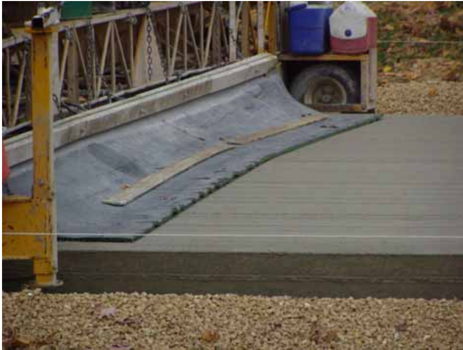
Figure A.7. Texturing operations
