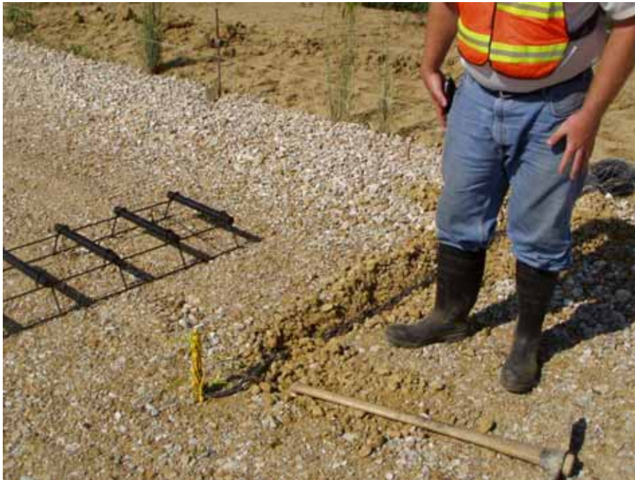
Figure D.6. Temperature instrumentation installation
