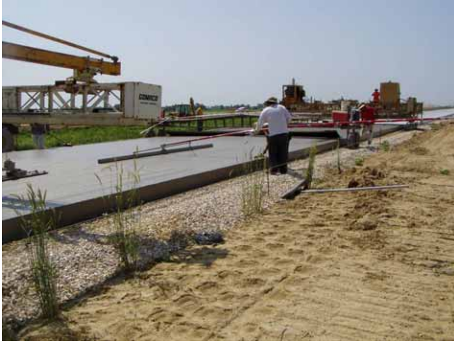
Figure. D.3. Finishing operations
