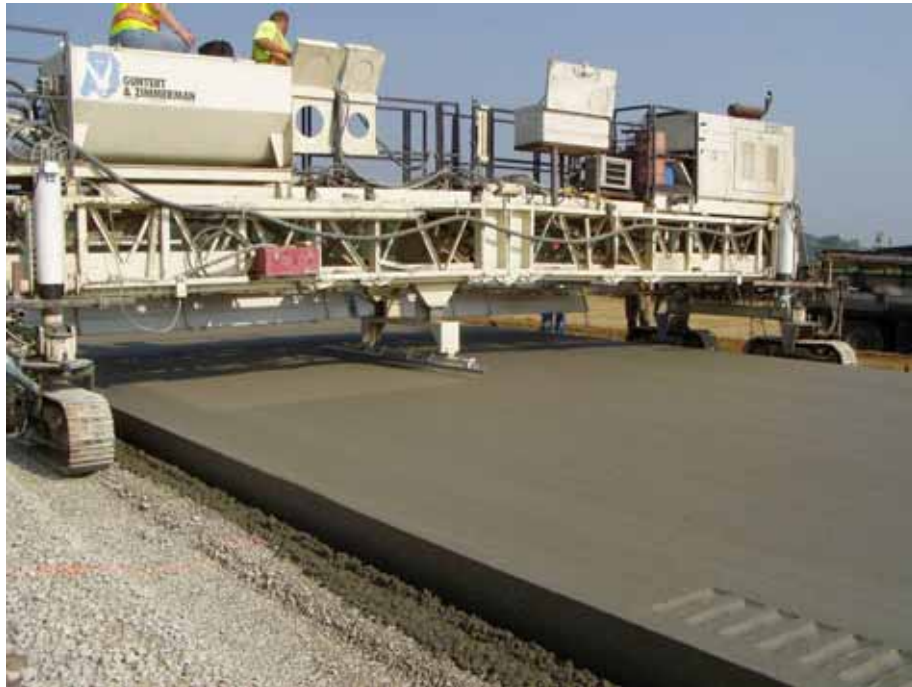
Figure G.5. Texturing and curing operations
