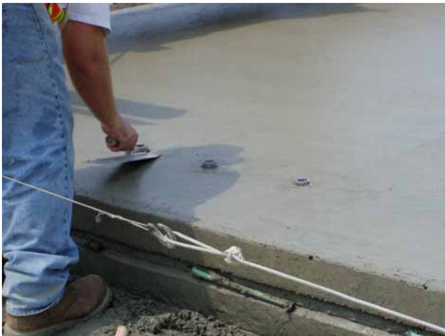
Figure G.10. Hygrochron instrumentation casing insertion
