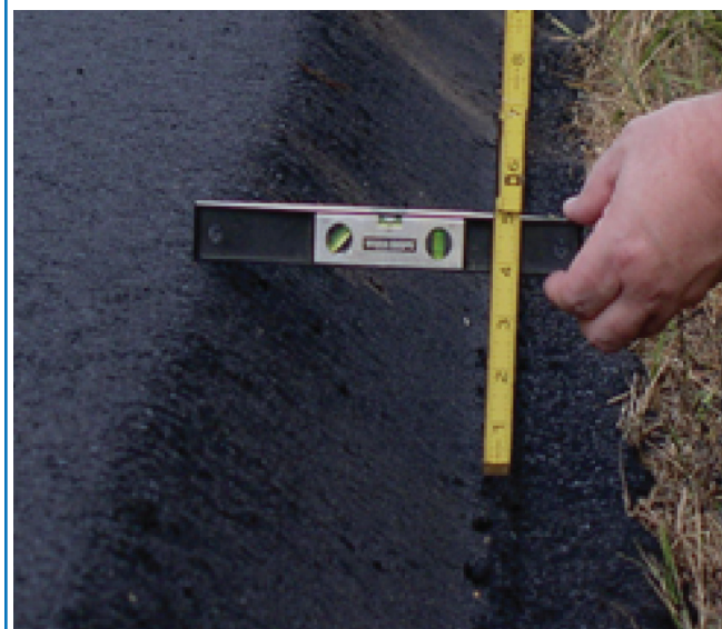
Pavement edge after resurfacing with Safety Edge
