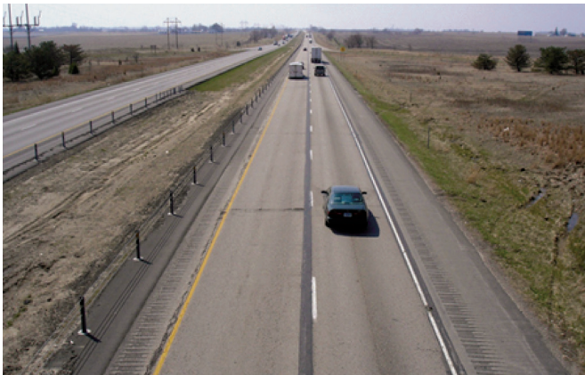
Figure 5.1. High-tension cable median barriers on Interstate 35 between Ames and Ankeny, Iowa
