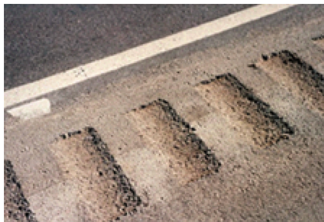
Figure 3.3. Milled-in shoulder rumble strips (Morena 2003)
