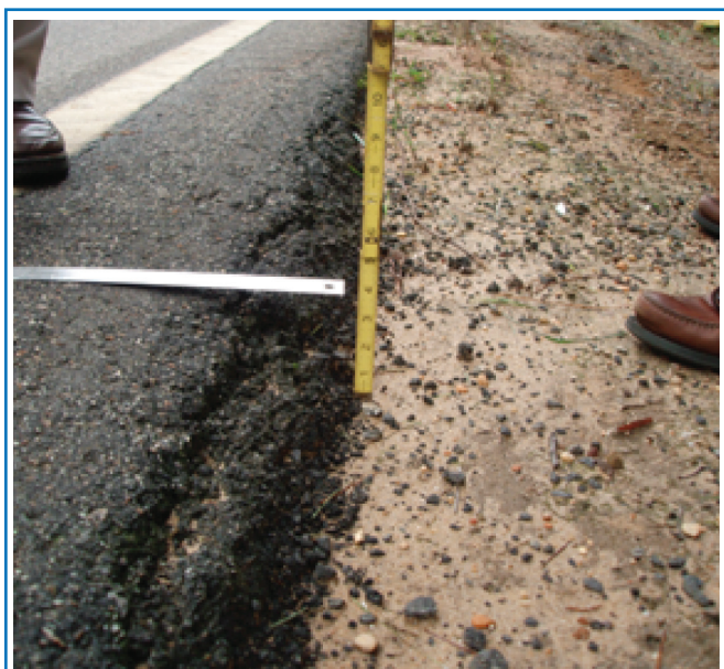
Pavement edge after resurfacing without Safety Edge
