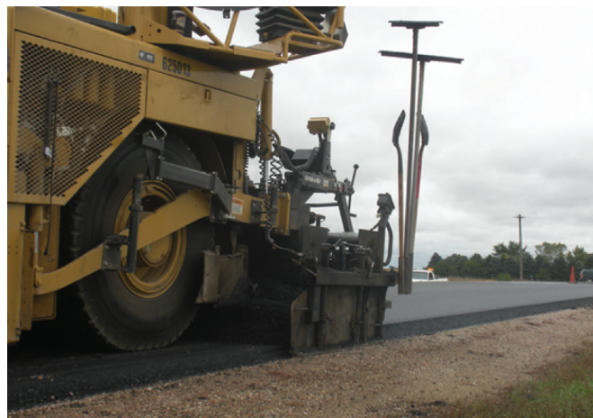
Figure 2.3. Application of the Safety Edge during resurfacing
