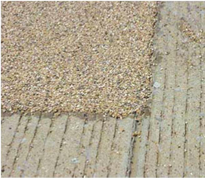
Figure 6.11: A high-friction surface treatment (Julian and Moler 2008)
