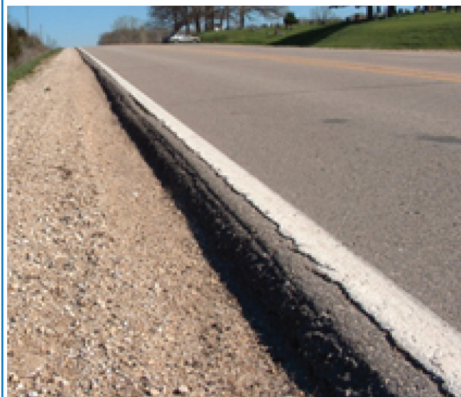
Typical rounded edge on asphalt
