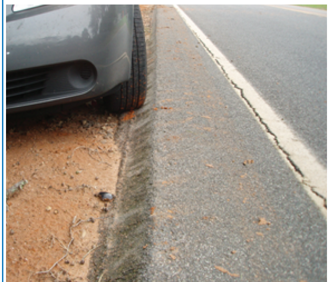
Pavement edge after resurfacing with Safety Edge
