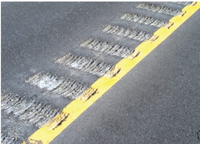
Figure 4.6. 18 inch CLRS in Iowa (Iowa DOT)
