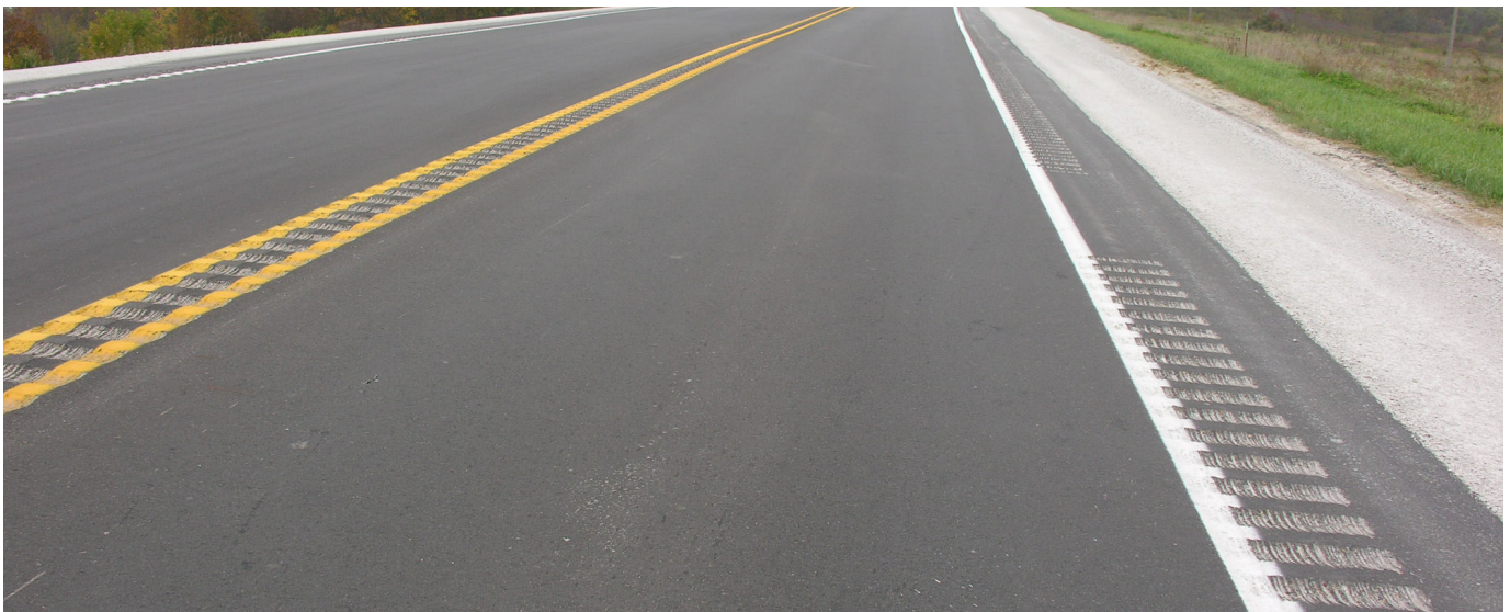
Figure 3.13 Gapped milled-in shoulder rumble stripes on US Highway 34 near Creston, Iowa (Roche 2011)
