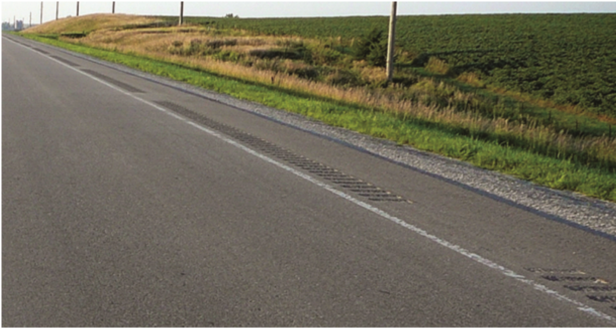
Figure 3.9. Gapped milled-in rumble strips on a state highway with 4 foot paved shoulders
