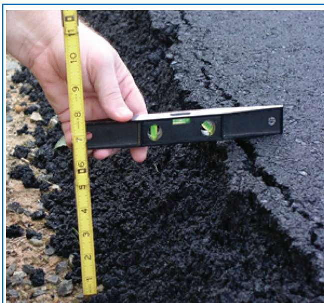
Pavement edge after resurfacing without Safety Edge
