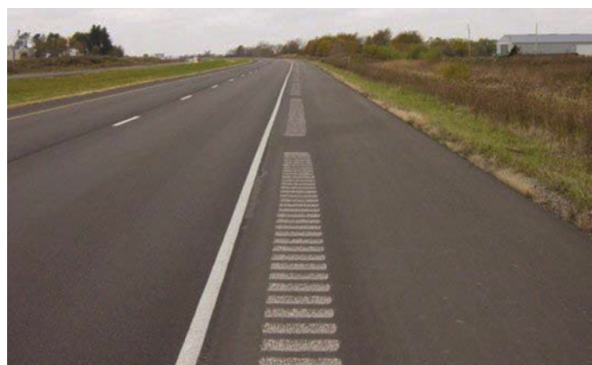
Figure 3.8. Gapped shoulder rumble strip pattern provides bicyclists with crossover spaces (Iowa DOT)
