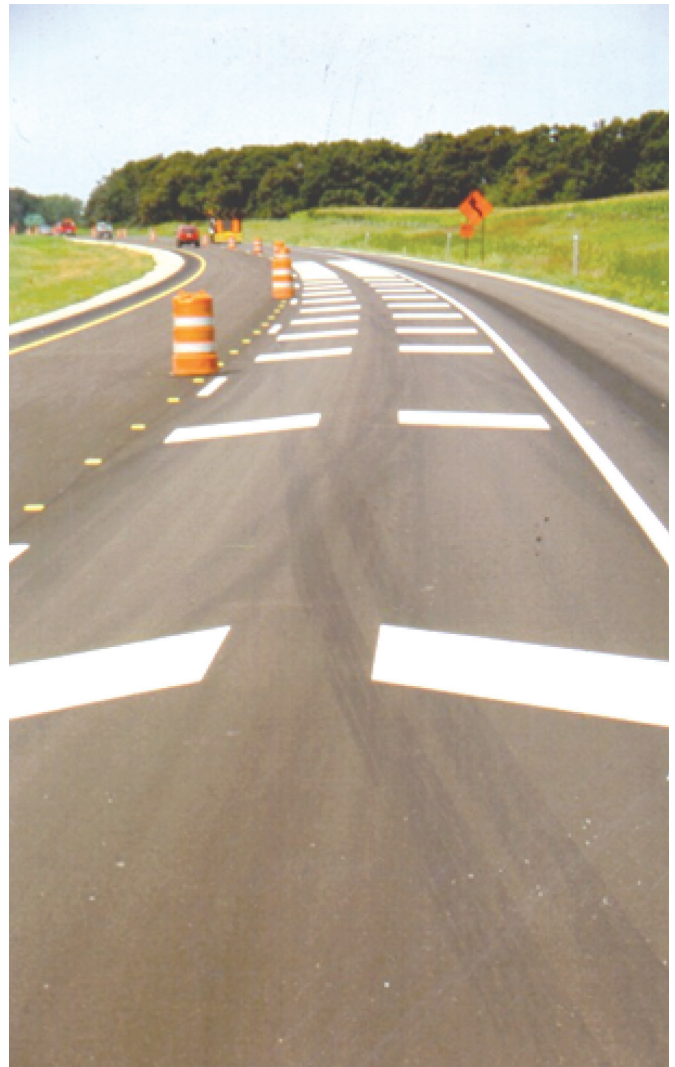
Figure 6.17. Mn/DOT "Tiger Tails" broken chevron pattern (Briese 2003)
