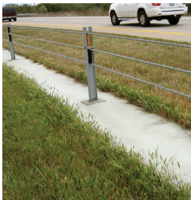
Figure 5.9. Mow strip for cable guardrails (WeedEnd®)
