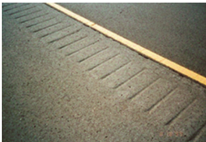
Figure 3.4. Rolled-in shoulder rumble strips (Morena 2003)
