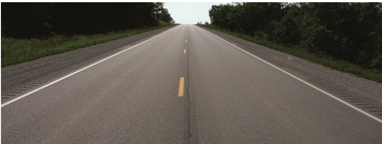
Figure 3.10. Continuous milled-in shoulder rumble strips on Iowa two-lane roadway with 2 foot paved shoulders
