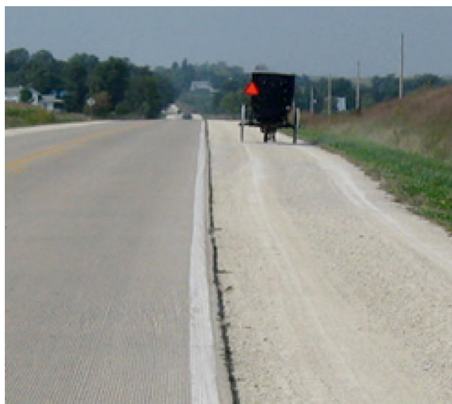
Figure 1.4. Horse and buggy traveling along an unpaved shoulder with edge drop-off (Hawkins, InTrans)
