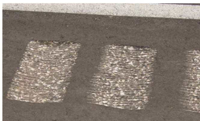
Figure 3.7. Milled shoulder rumble strips (Iowa DOT)
