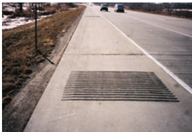
Figure 3.5. Formed-in shoulder rumble strips (Morena 2003)
