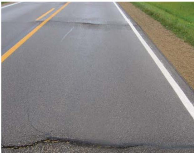
*This PCC pavement overlaid with HMA without rubblization of the existing pavement slabs exhibited high levels of reflective cracking.*
