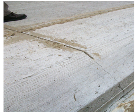
Safety Edge application (top), pavement with significantly more vertical toe (lower left), saw-cut transverse joint and expected Safety Edge crack (lower right)
