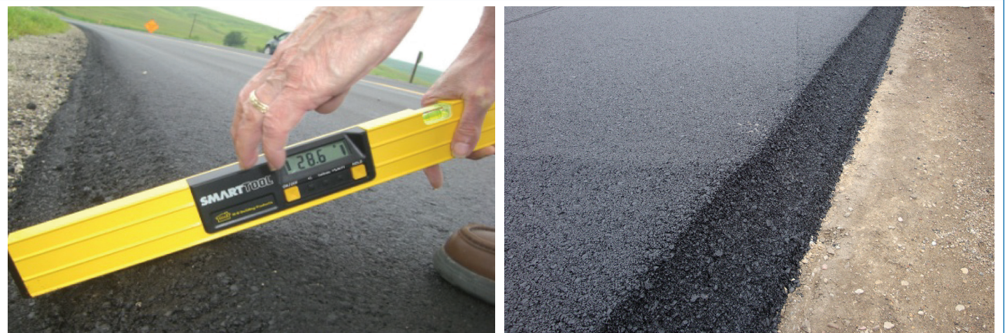
Safety Edge slope measurement (left) and warm-mix asphalt Safety Edge application (right)
