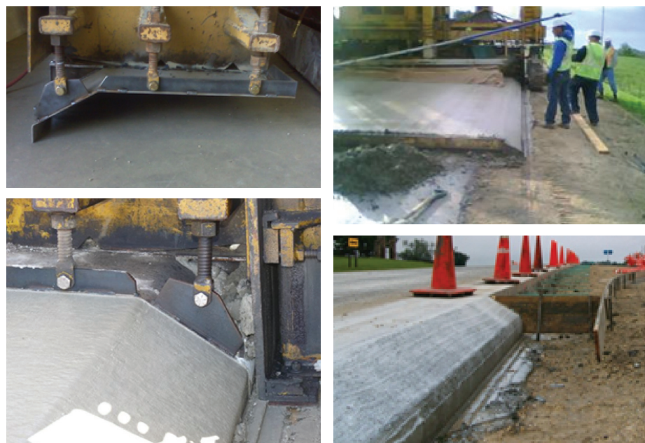
Angled plate and assembly welded to the paver pan (upper left), Safety Edge extrusion (lower left), start of project paving (upper right), and "box-out" and re-bar for intersection (lower right)
