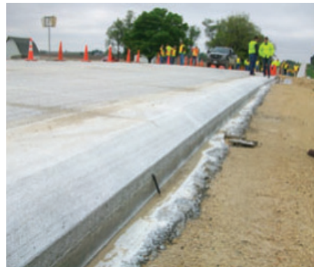
Safety Edge application (top), pavement with significantly more vertical toe (lower left), saw-cut transverse joint and expected Safety Edge crack (lower right)
