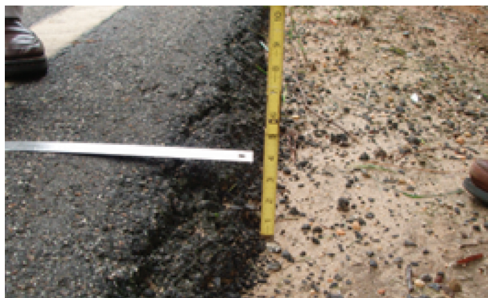
Pavement edge six years after resurfacing without the Safety Edge (left) and with the Safety Edge (right) (Roche, 2009)
