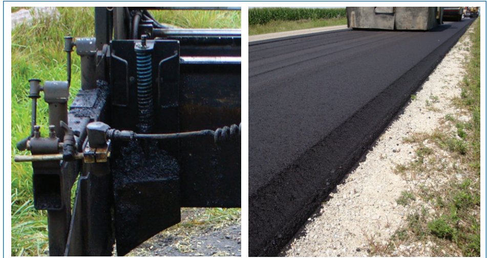
Advant-Edger installed and in use (left) and Safety Edge applied (right)
