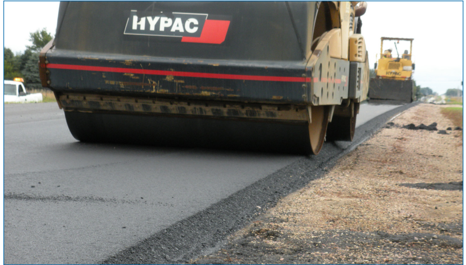
Quality assurance during paving includes slope measurement, as well as monitoring for rollover
