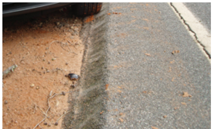
Pavement edge six years after resurfacing without the Safety Edge (left) and with the Safety Edge (right) (Roche, 2009)
