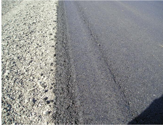
Figure 7.8. Finished Safety Edge Slope on CR H24 in Union County
