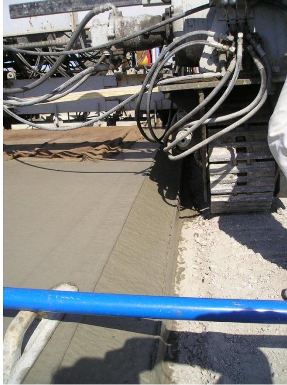
Figure 6.6. PCC paver modification for the Keokuk County Safety Edge
