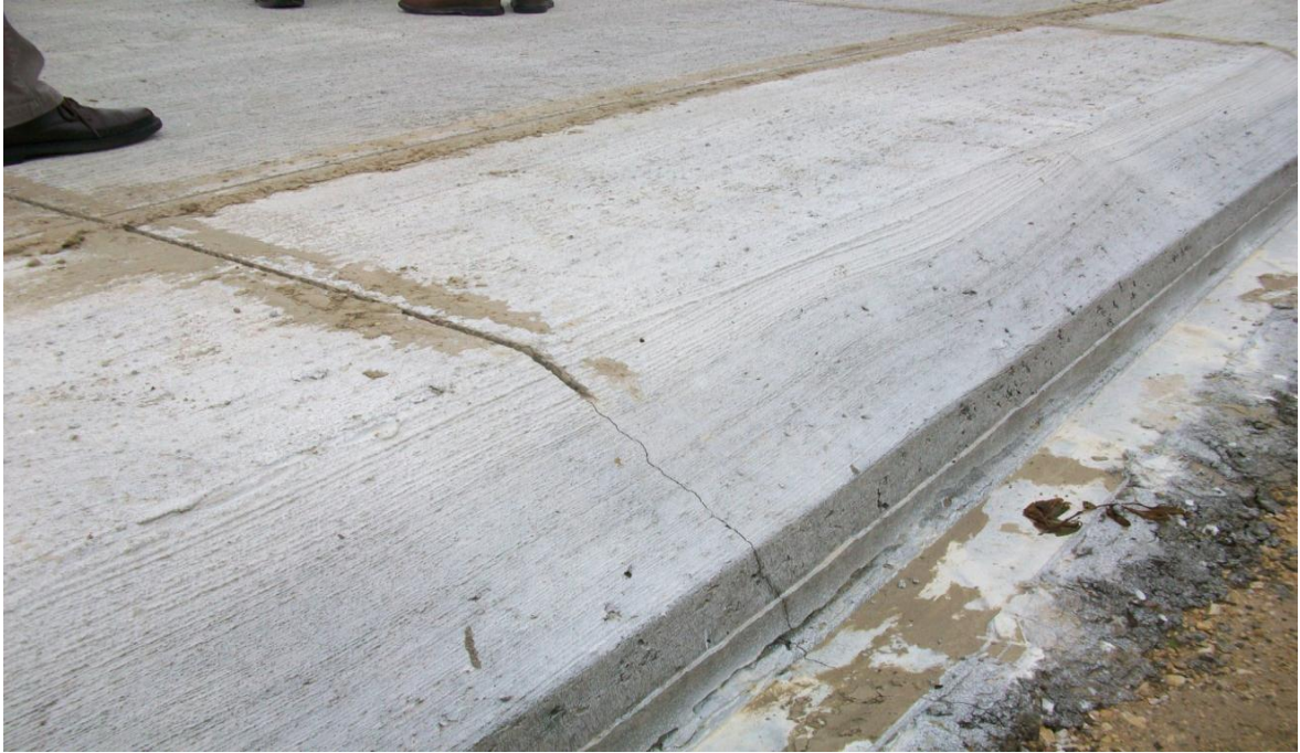
Figure 6.10. Saw cut transverse joint with the Safety Edge
