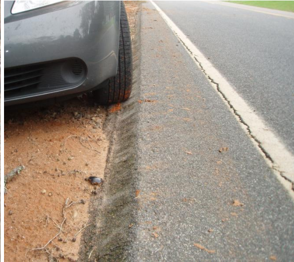
Pavement edge after resurfacing with Safety Edge
