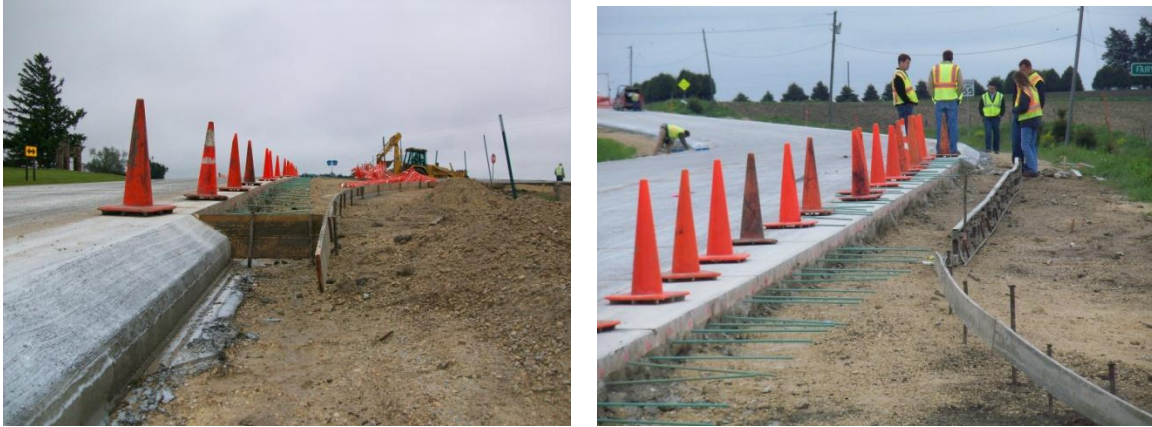
Figure 6.7. Safety Edge modifications at a paved road intersection
