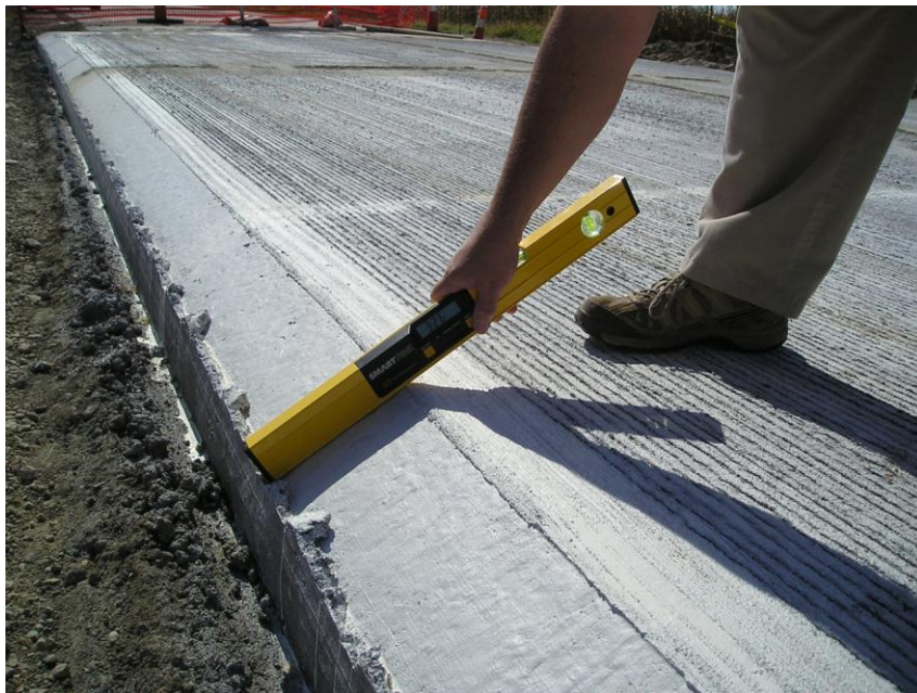
Figure 7.4. Safety Edge on Keokuk CR V63
