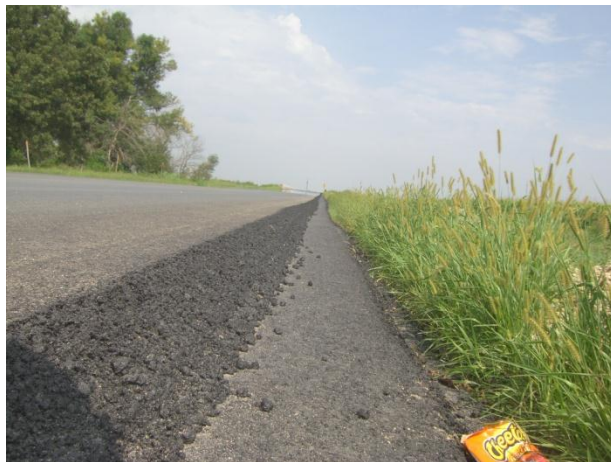
Excess width in base for second and third lifts
