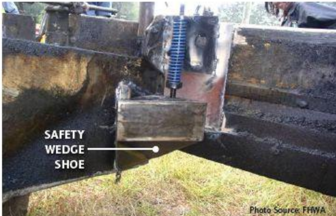
Figure 2.1. Trans Tech safety wedge shoe (FHWA, 2009a)
