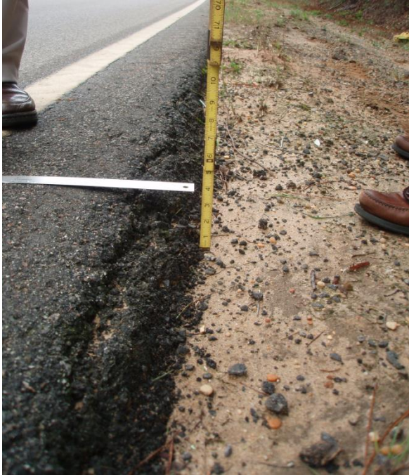
Pavement edge after resurfacing without Safety Edge
