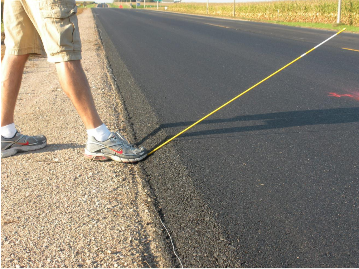
Figure 1.4. Pavement edge shape resulting from application of the Safety Edge
