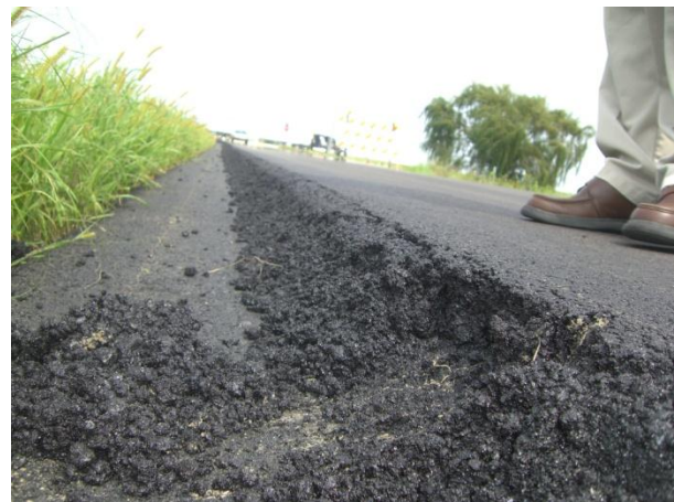
Excess base and insufficient second width for third lift
