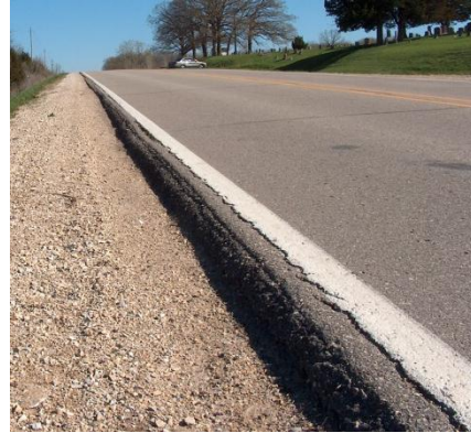
Typical rounded edge with hot-mix asphalt pavement
