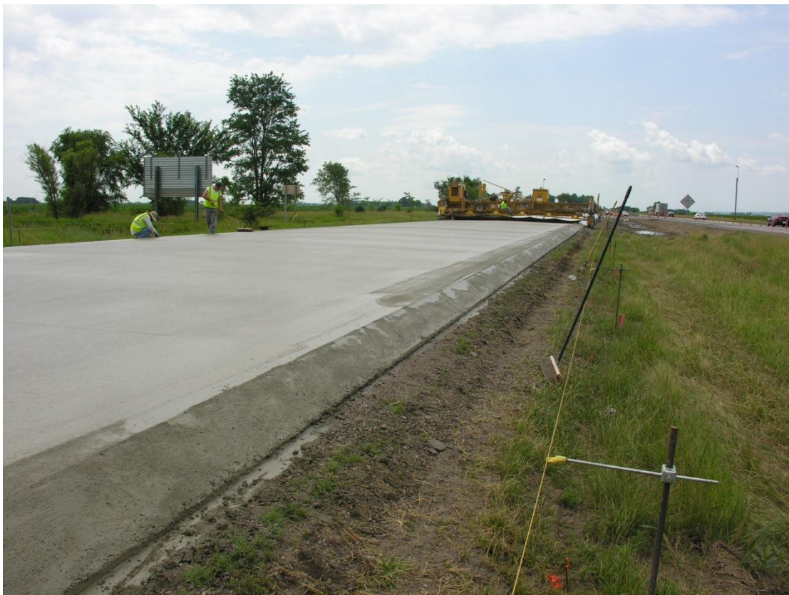
Figure 7.1. Sloped edge on I-29 in Woodbury County
