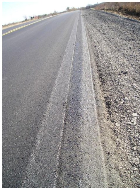
Figure 8.2. Improved safety edge resulting from modified shoes
