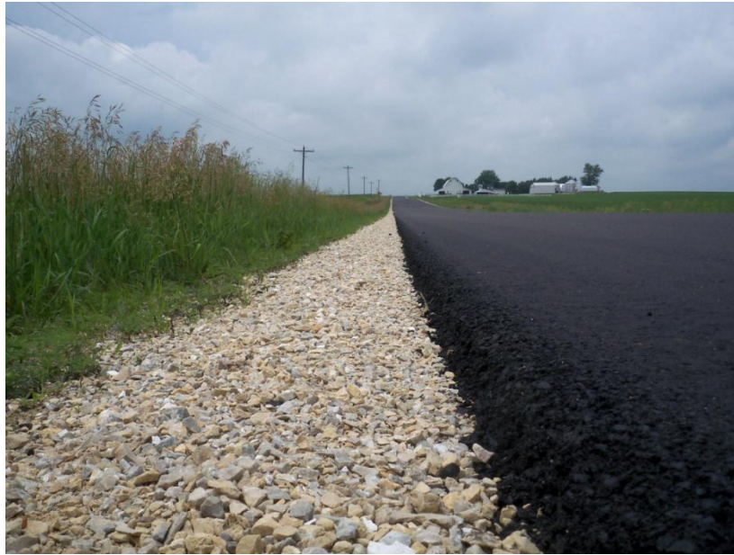
Figure 7.11. Typical Safety Edge on CR D34 in Delaware County
