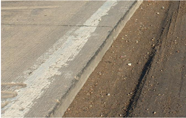
Typical vertical edge with Portland cement concrete pavement
