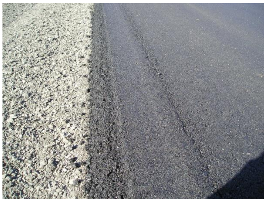
Figure 8.2. Improved safety edge resulting from modified shoes
