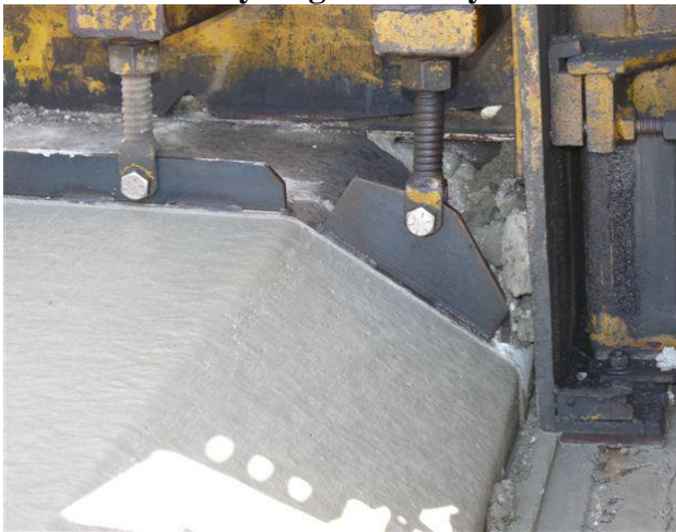
Extrusion of the Safety Edge
