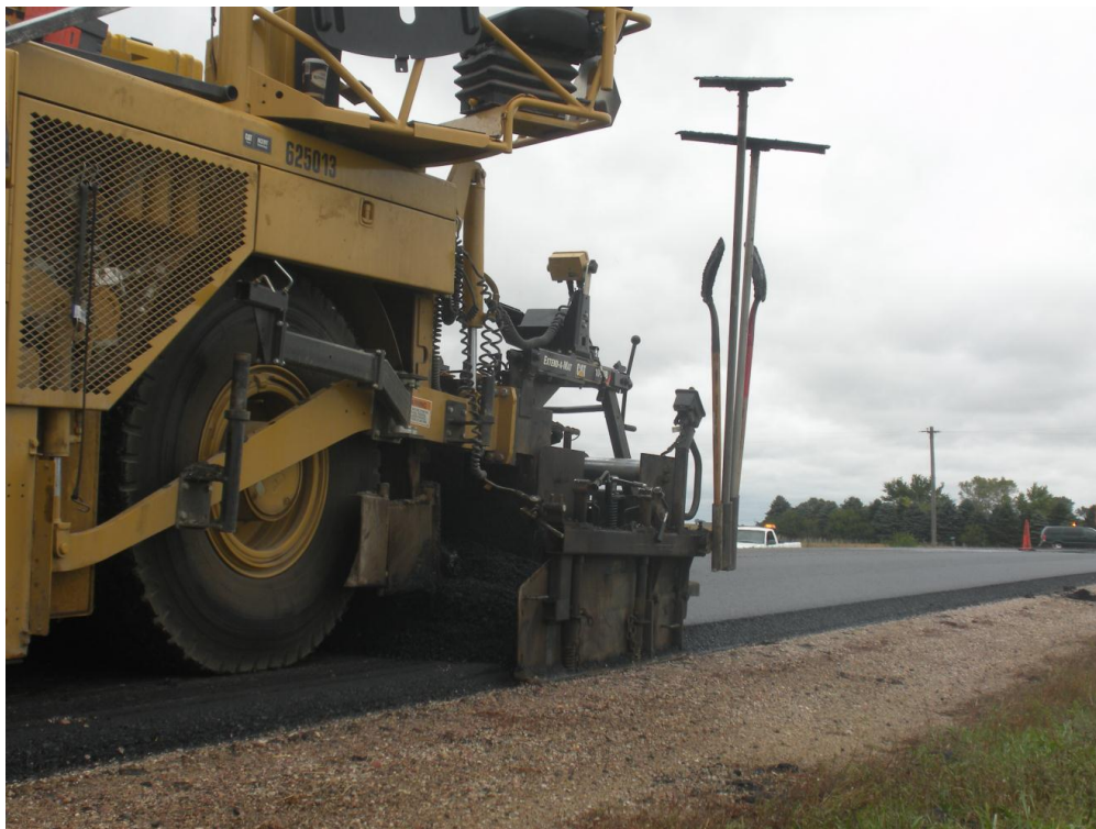
Figure 1.3. Application of the Safety Edge during paving
