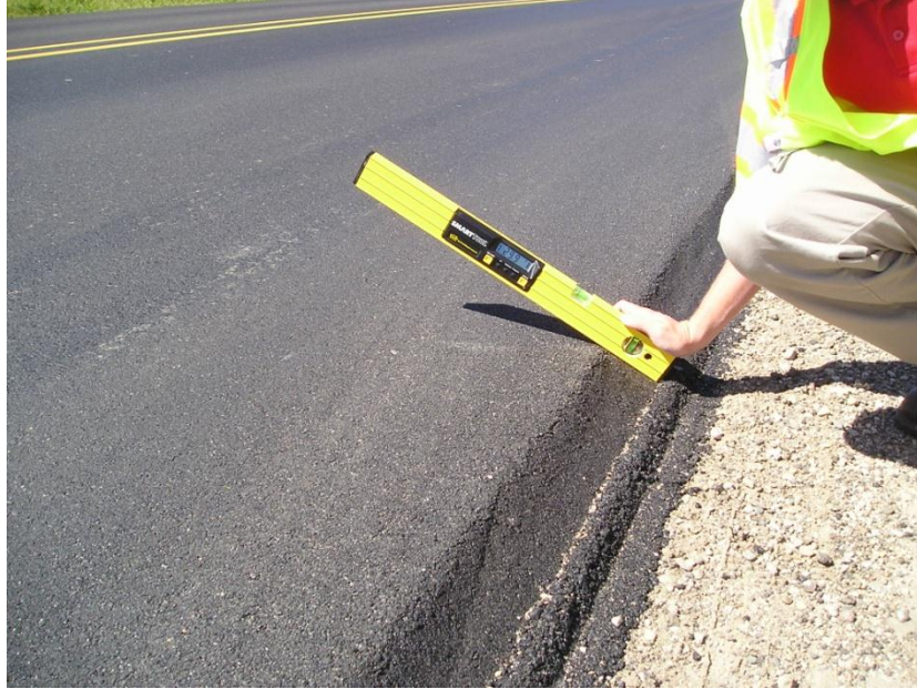
Figure 5.1. Measurement of Safety Edge slope with SmartTool
