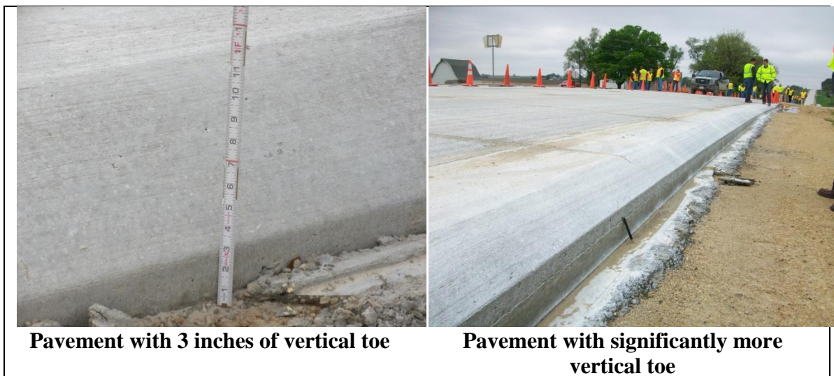
Figure 6.8. Placement with various dimensions of vertical toe
