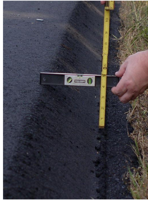
Pavement edge after resurfacing with Safety Edge
