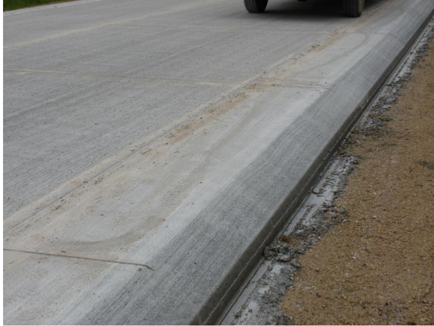
Figure 7.3. Finished PCC Safety Edge for CR E34 in Jones/Linn Counties
