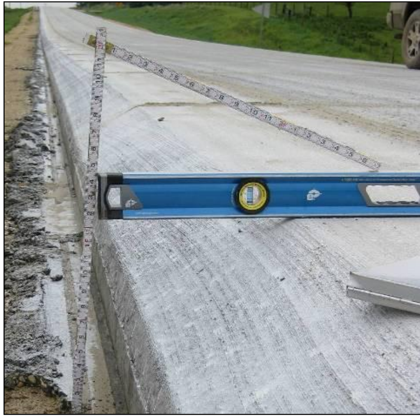
Figure 6.9. Edge of PCC Safety Edge showing ridge and bow (FHWA, 2011)
