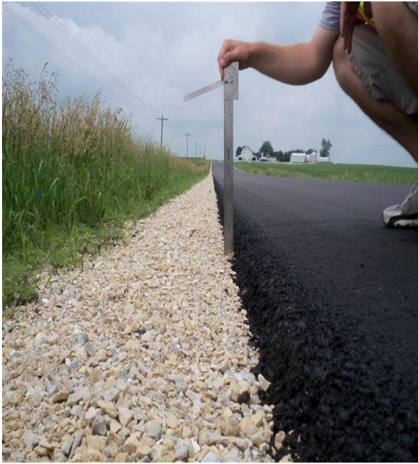
Pavement edge after resurfacing without Safety Edge
