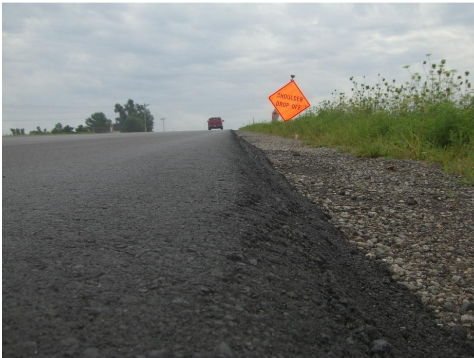
Figure 7.10. Completed Safety Edge on CR Y26 in Cedar County
