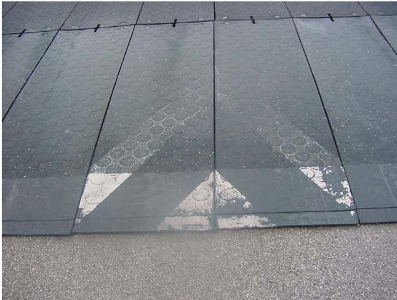
**Figure 24. Pavement Markings After Approximately Six Months**
