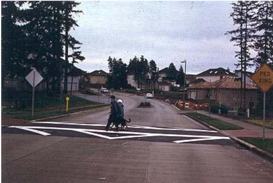
**Figure 2. Typical Speed Table
