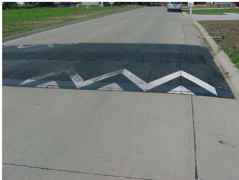
**Figure 23. Pavement Markings on Speed Hump/Table**
