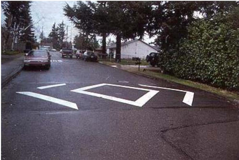
**Figure 1. Typical Speed Hump
