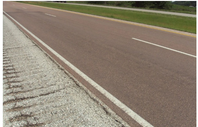
Moisture-related distresses on HMA over JPCP-type composite pavement system where no drainage outlets located in the field
