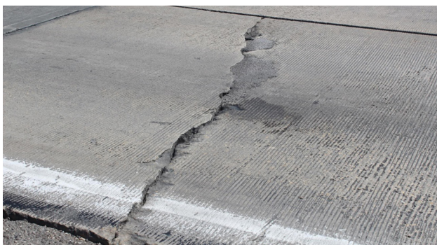
Moisture-related distresses on JPCP where no drainage outlets located at site
