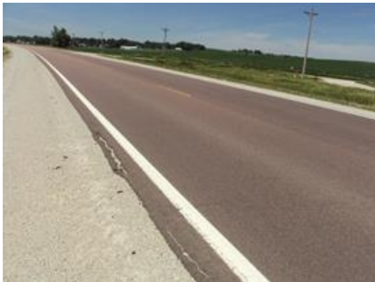
Transverse cracking
