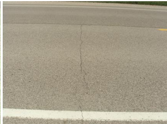
Transverse cracking
