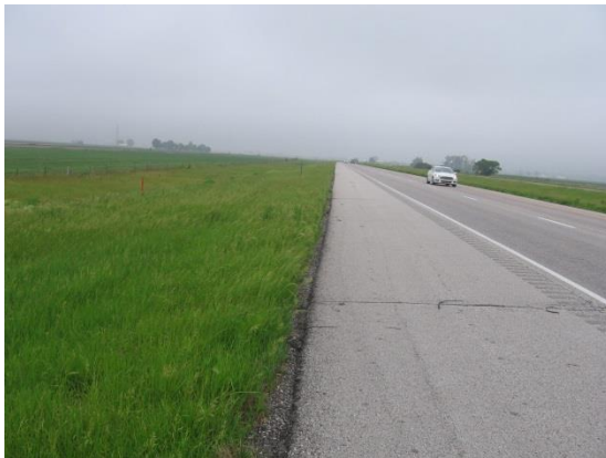
No drainage outlet
