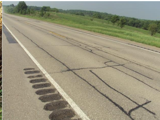
Longitudinal and transverse cracking patching
