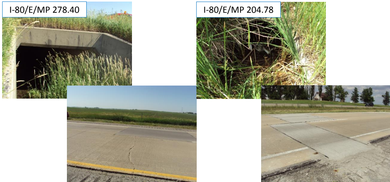
Figure 17. Cracking/patching observed near culvert-only/culvert with drainage outlet locations in newly constructed JPCP sites
