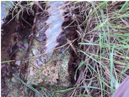
Tufa blockage/damaged outlet pipe
