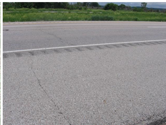
Transverse cracking
