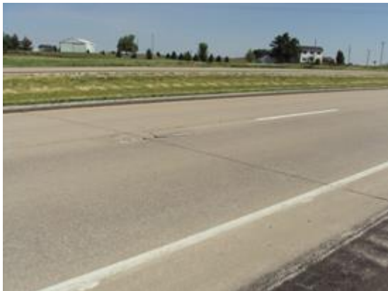
Corner crack
