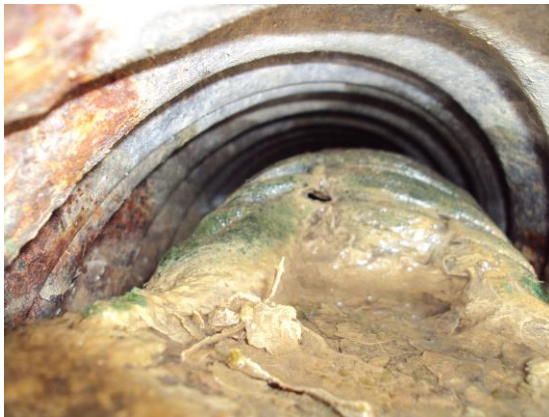
Tufa blockage extends back into the pipe
