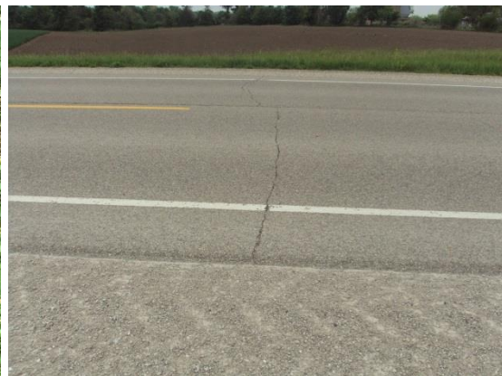
Transverse cracking
