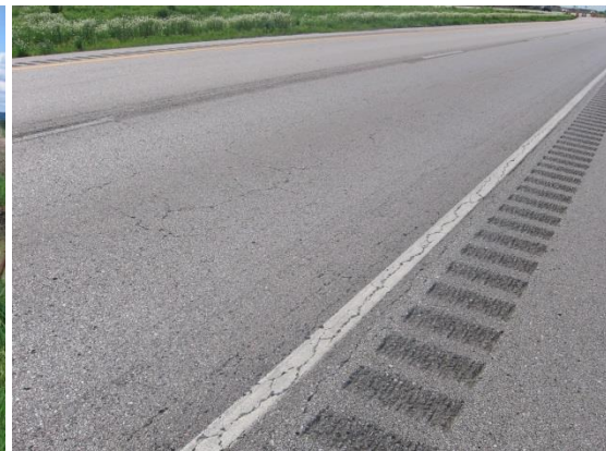
Alligator cracking/corner erosion damage
