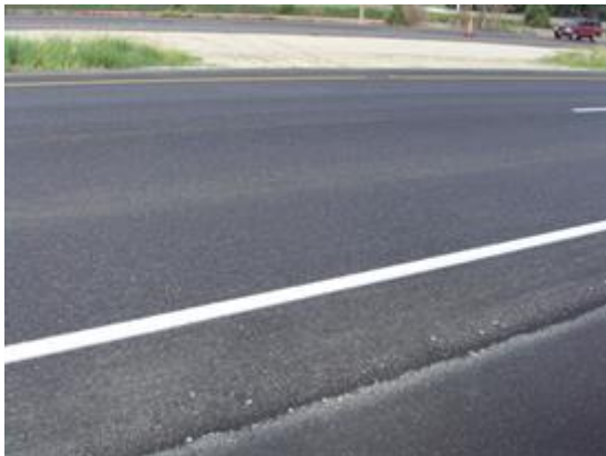
New HMA overlay
