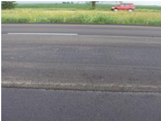
New HMA overlay
