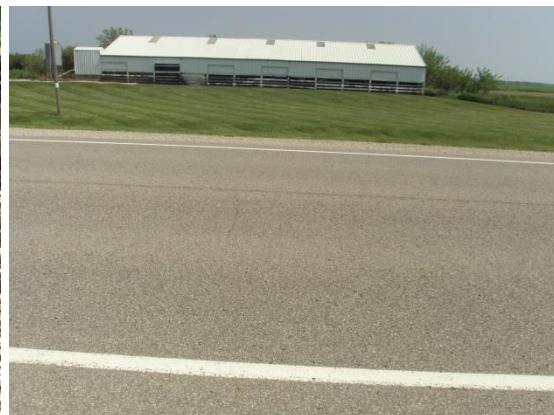
Transverse cracking
