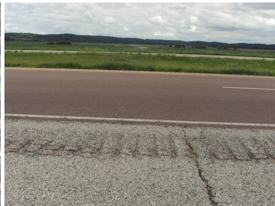
Rutting/transverse cracking
