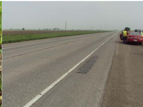
Transverse cracking
