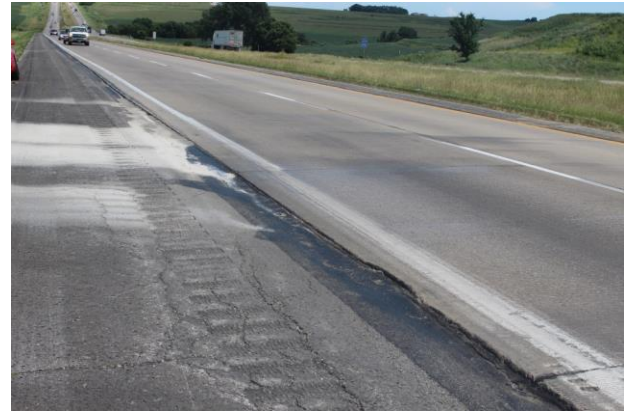
Figure 18. Moisture-related damage observed on JPCP sites where no drainage outlet was found
