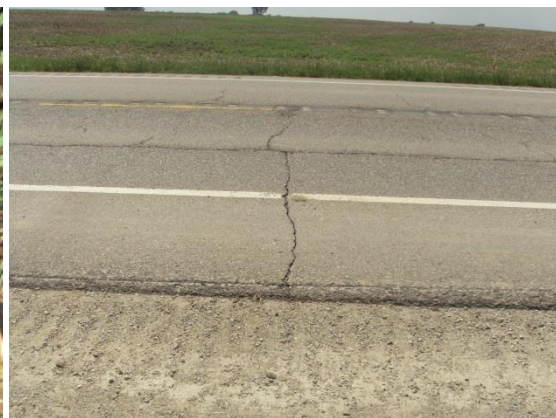
Longitudinal and transverse cracking
