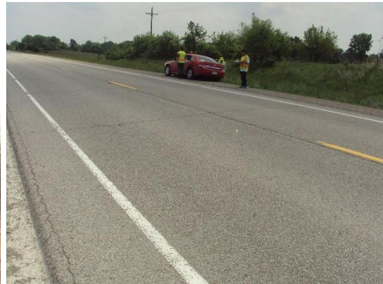
Reflection cracking
