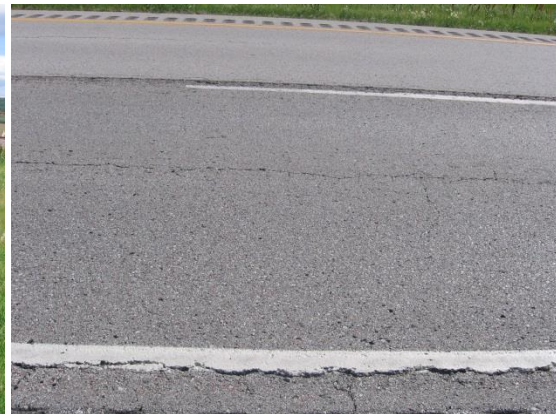
Alligator and transverse cracking
