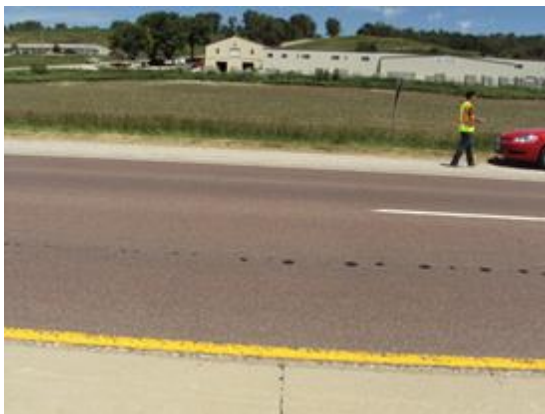
Transverse cracking
