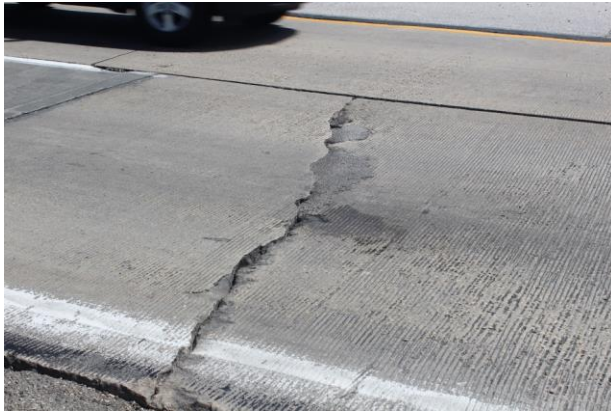
Figure 18. Moisture-related damage observed on JPCP sites where no drainage outlet was found
