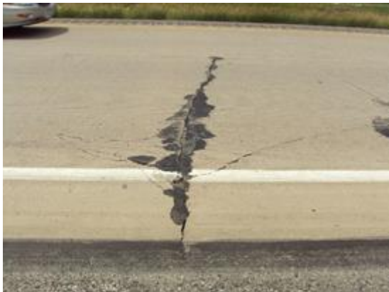
Longitudinal and transverse cracking
