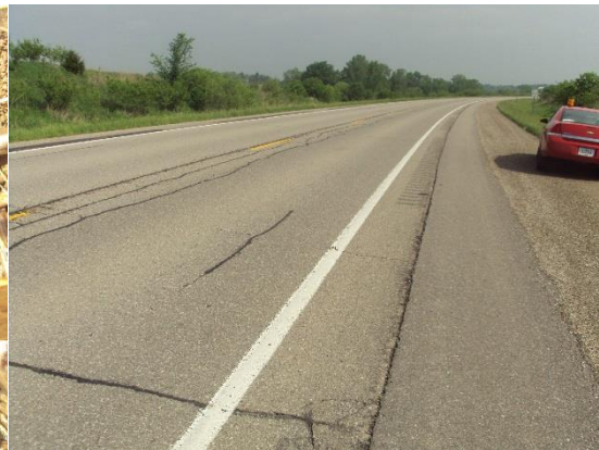
Longitudinal and transverse cracking patching
