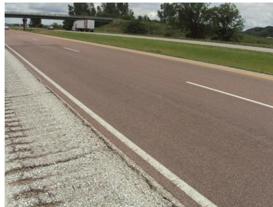
Figure 25. Moisture-related damage observed on HMA over JPCP sites where no drainage outlet was found
