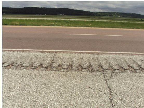
Transverse cracking
