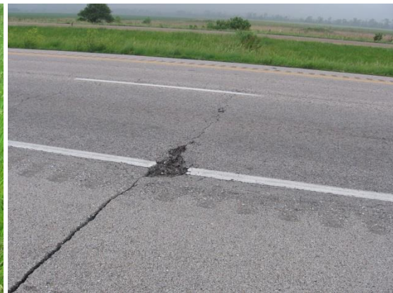
Transverse and alligator cracking
