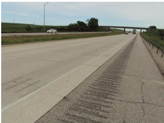
Transverse cracking due to culvert
