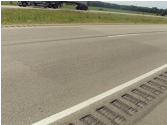
Pavement surface grinding
