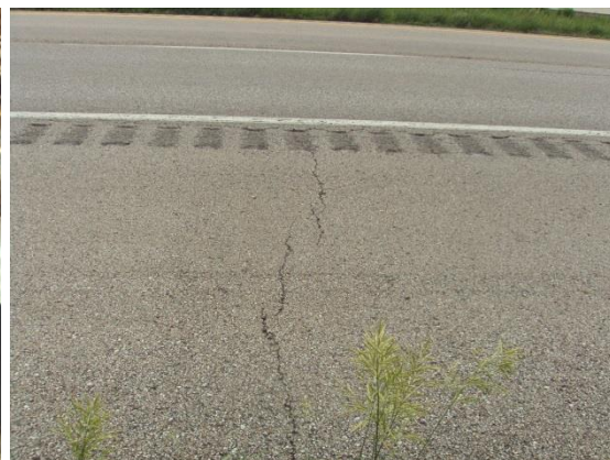
Transverse cracking
