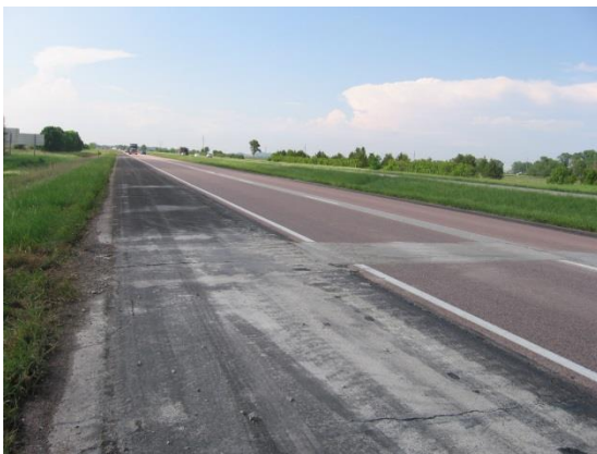
Reflection cracking/concrete patching
