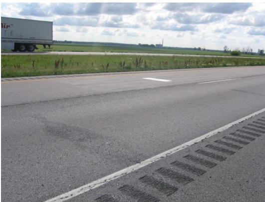
Figure 25. Moisture-related damage observed on HMA over JPCP sites where no drainage outlet was found
