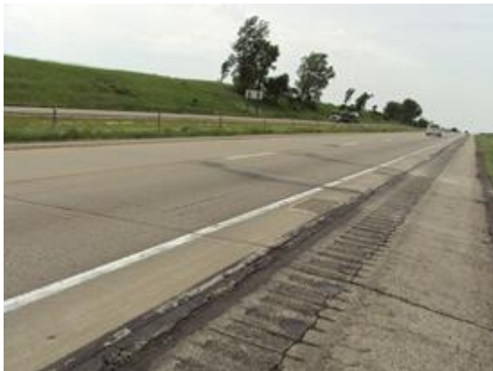
Transverse cracking
