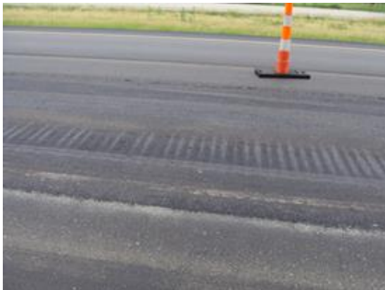
New HMA overlay
