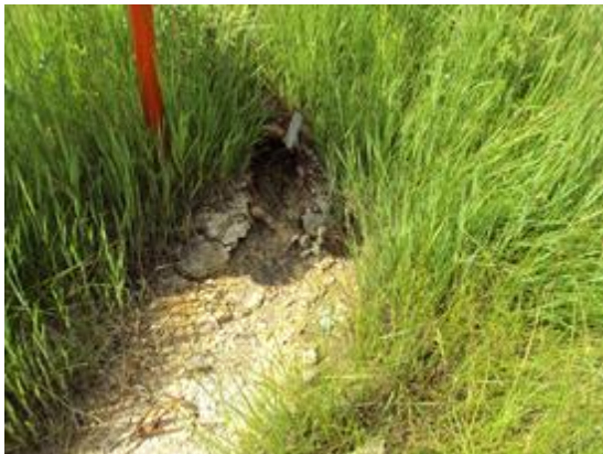
Pipe damaged during tufa removal
