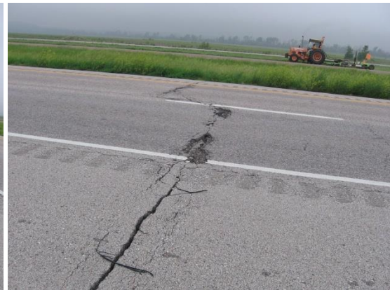
Transverse and alligator cracking
