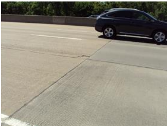
Small corner crack
