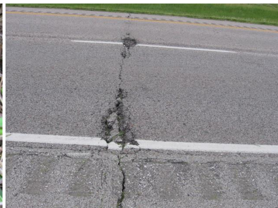
Transverse and alligator cracking
