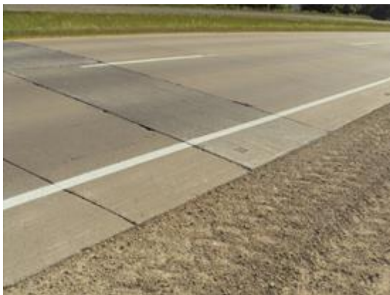
Pavement patching due to culvert
