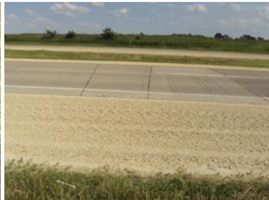
Pavement patching due to culvert
