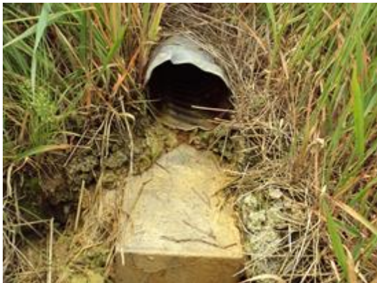
Good drainage pad installation
