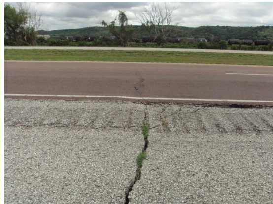
Transverse cracking/rutting
