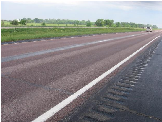
Reflection cracking
