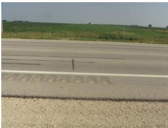
Longitudinal and transverse cracking patching
