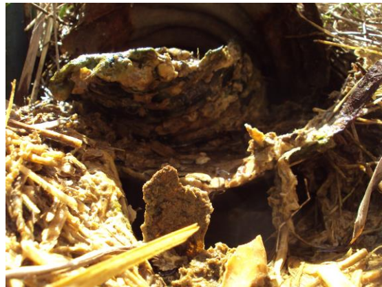
Damaged and tufa formation at outlet
