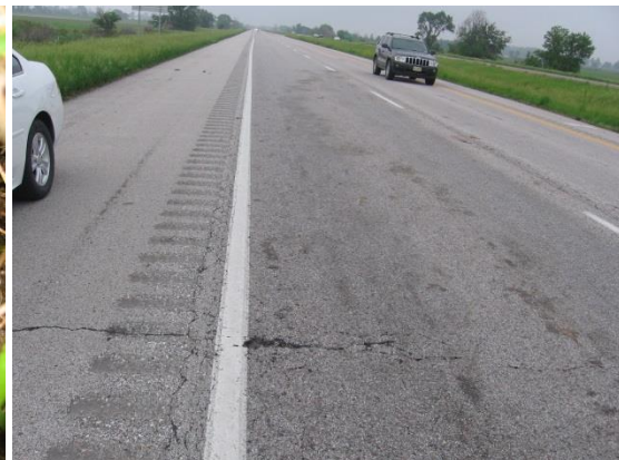
Longitudinal and transverse cracking/rutting
