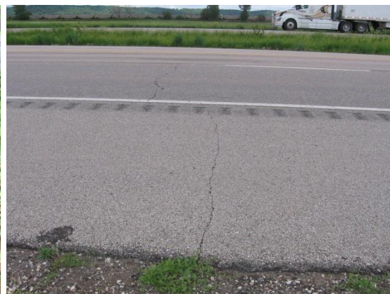
Transverse cracking
