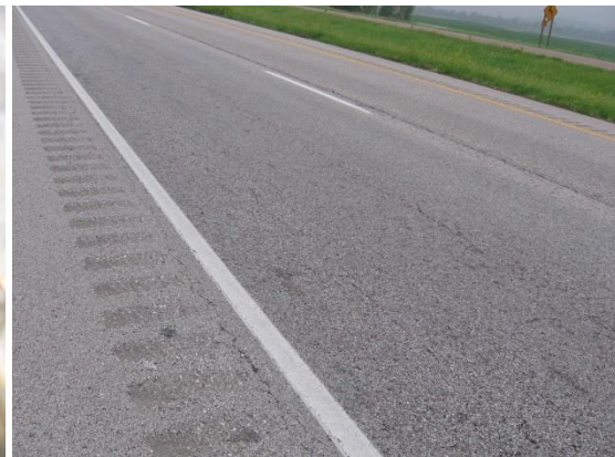
Alligator cracking
