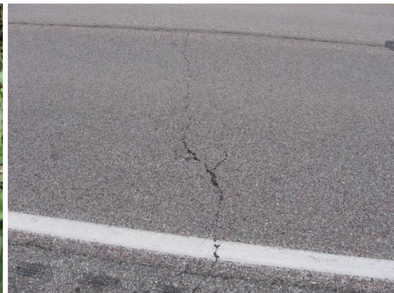
Transverse cracking
