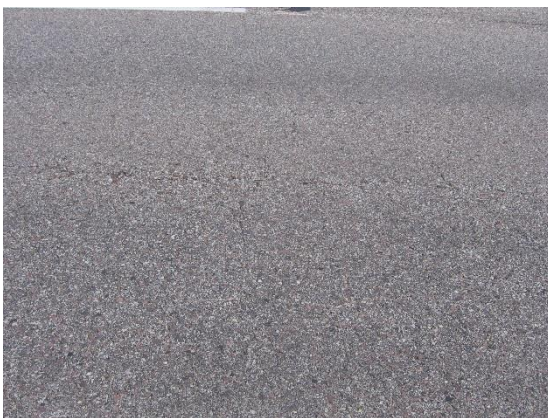
Alligator cracking
