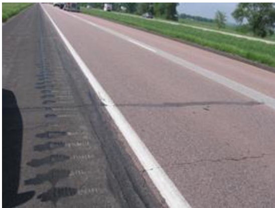
Reflection and transverse cracking
