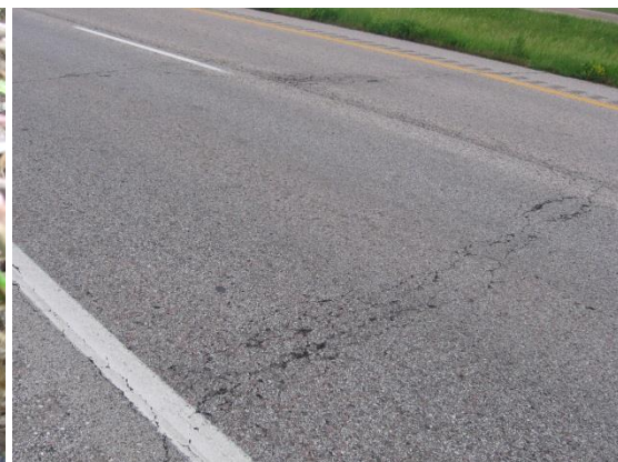
Transverse and alligator cracking/rutting
