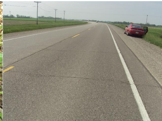
Reflection cracking
