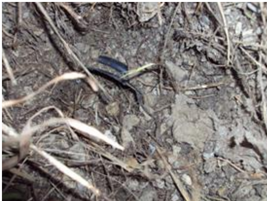
Soil blockage/damaged outlet pipe
