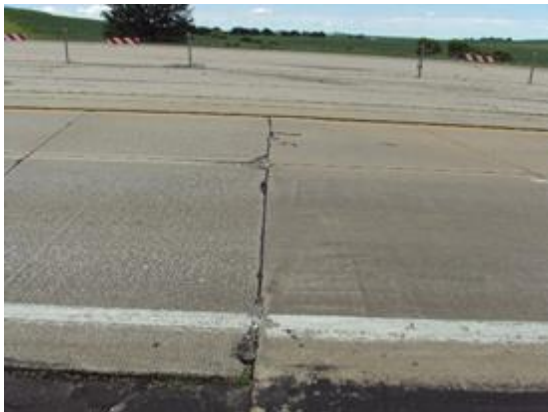
Corner cracking
