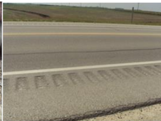
Longitudinal cracking patching
