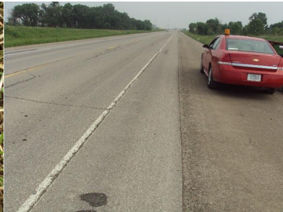
Longitudinal and reflection cracking
