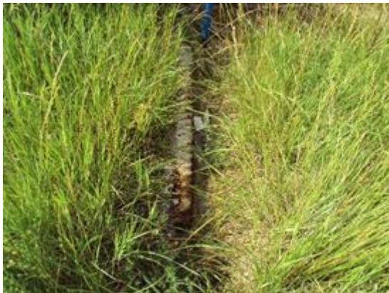
Tufa blockage and damage
