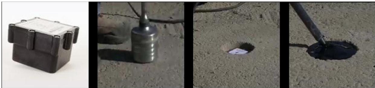
**Figure 60. Wireless VDS sensor installation (Bajwa et al. 2011)**
