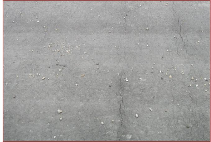
*Transverse cracking on Span 1 (with plywood) two months post construction*
