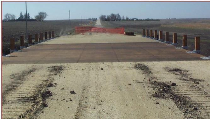
*Bridge after plywood and guardrail posts installed*
