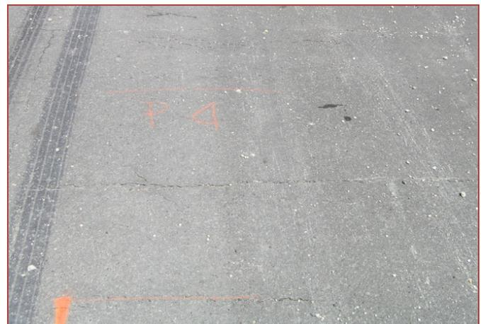
*Transverse cracking on Span 1 (with plywood) one year post construction; visible cracking evident at the transverse plywood joints as well as at the panel joints*
