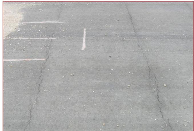
*Transverse cracking on Span 2 (no plywood) two months post construction*
