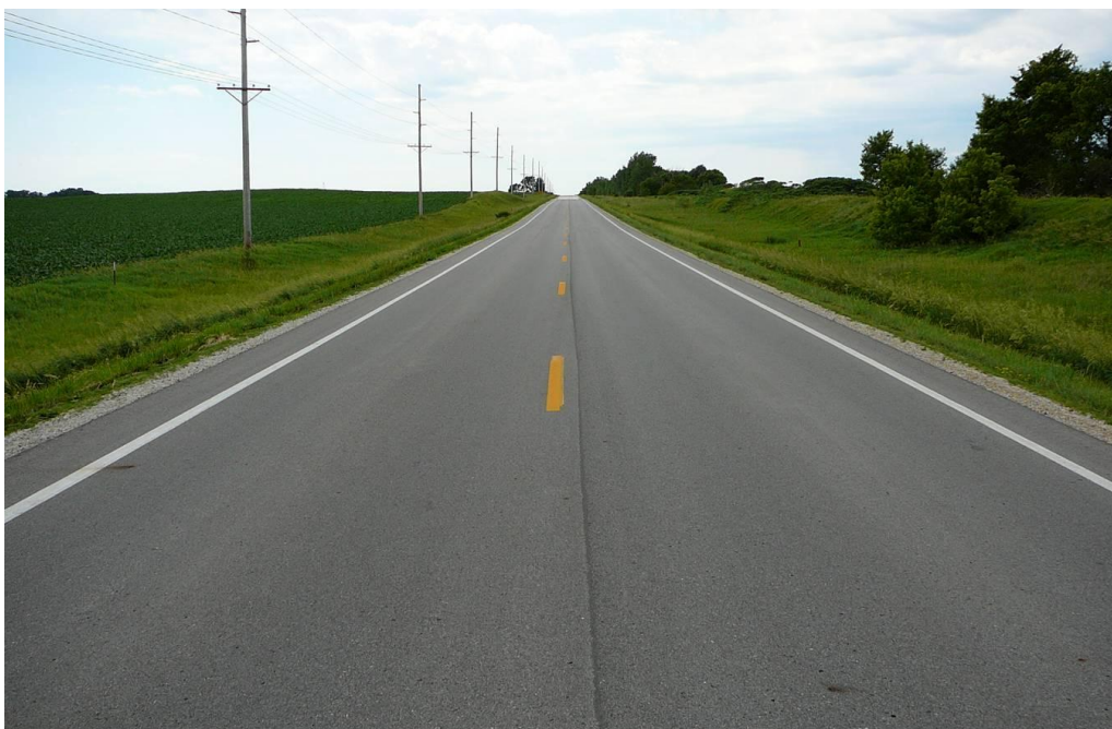
Figure 4.5. Two-lane highway with partially paved shoulders
