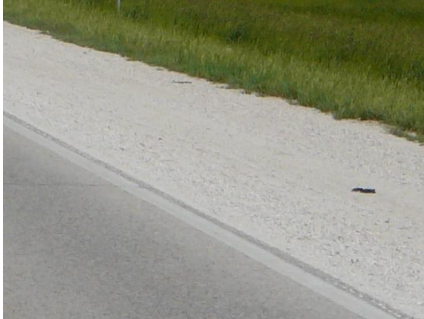
Figure 4.1. Typical gravel unpaved shoulder type
