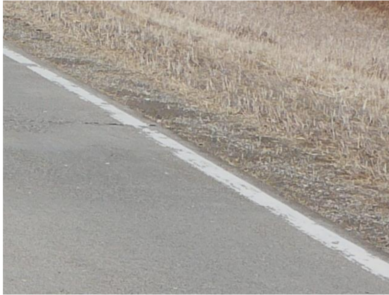
Figure 4.3. Typical mixed unpaved shoulder type
