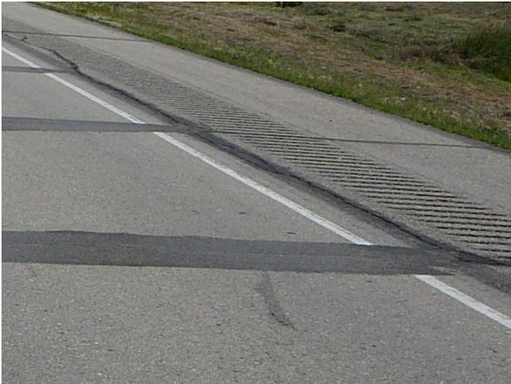
Figure 4.7. Rolled rumble strips
