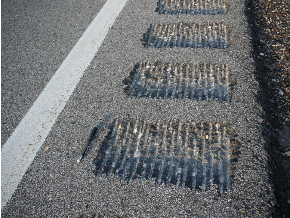
Figure 4.8. Milled rumble strips
