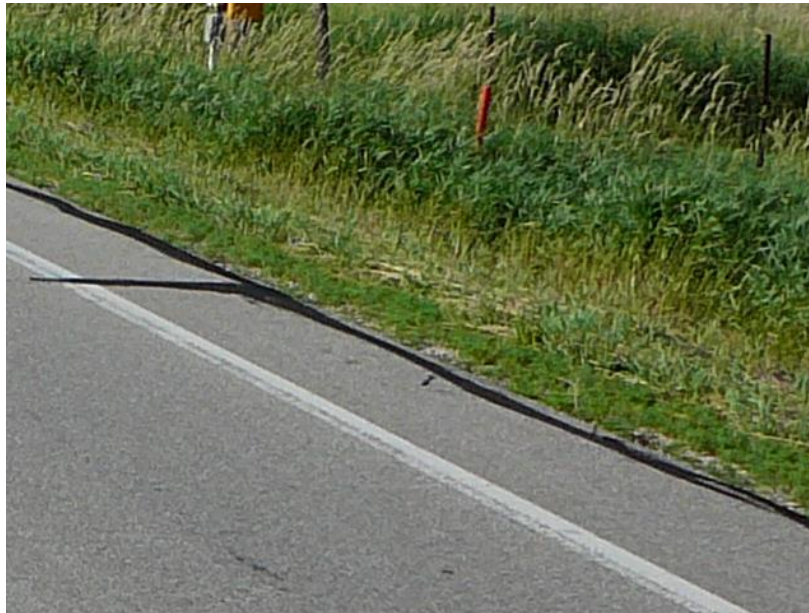
Figure 4.2. Typical earth unpaved shoulder type
