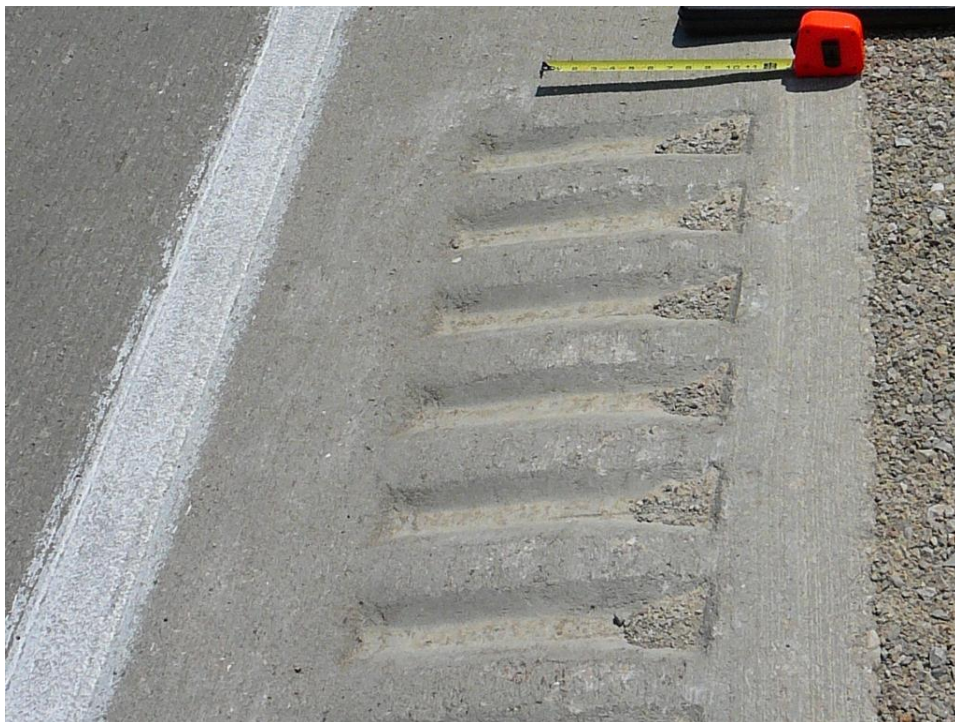
Figure 4.9. Formed rumble strips
