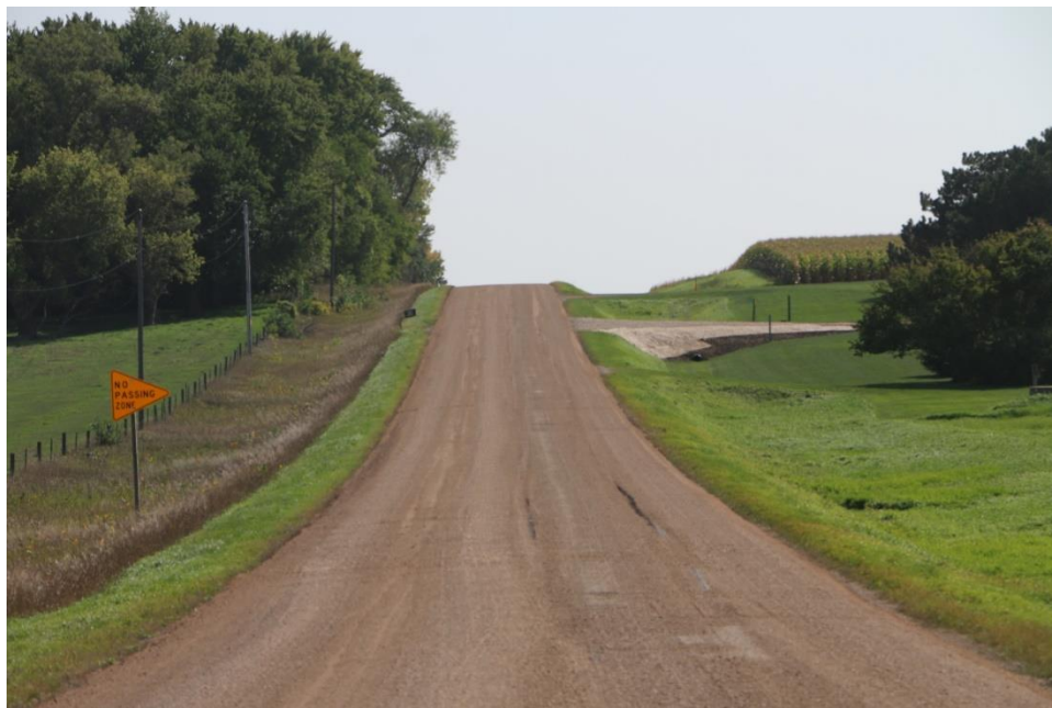
Figure 127. Appearance at a slope area of Otta seal two days post construction
