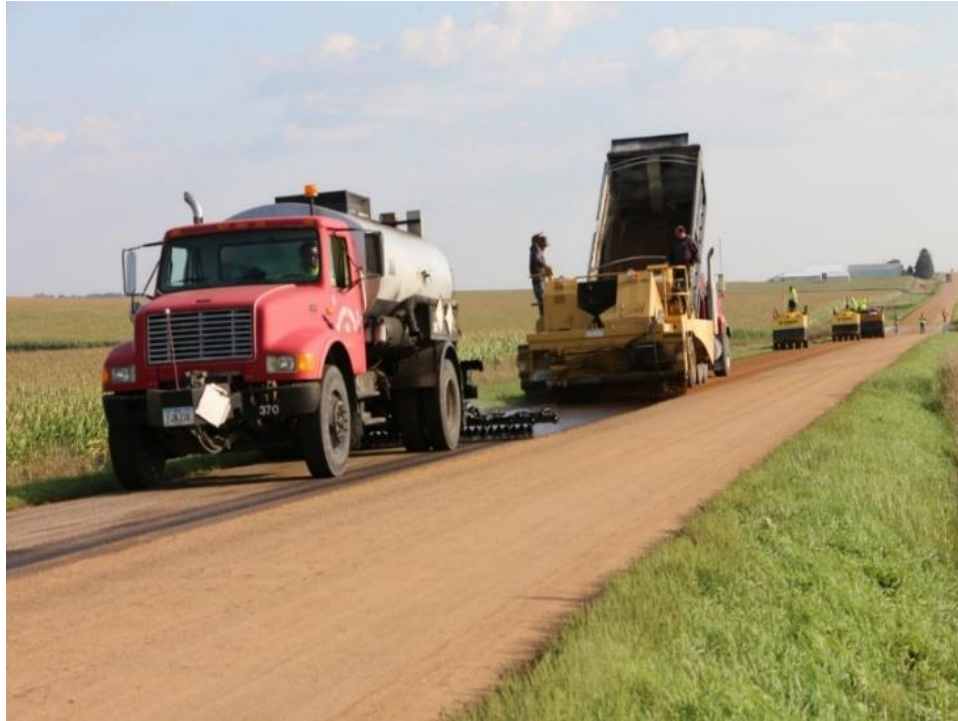
Figure 48. The entire Otta seal construction process
