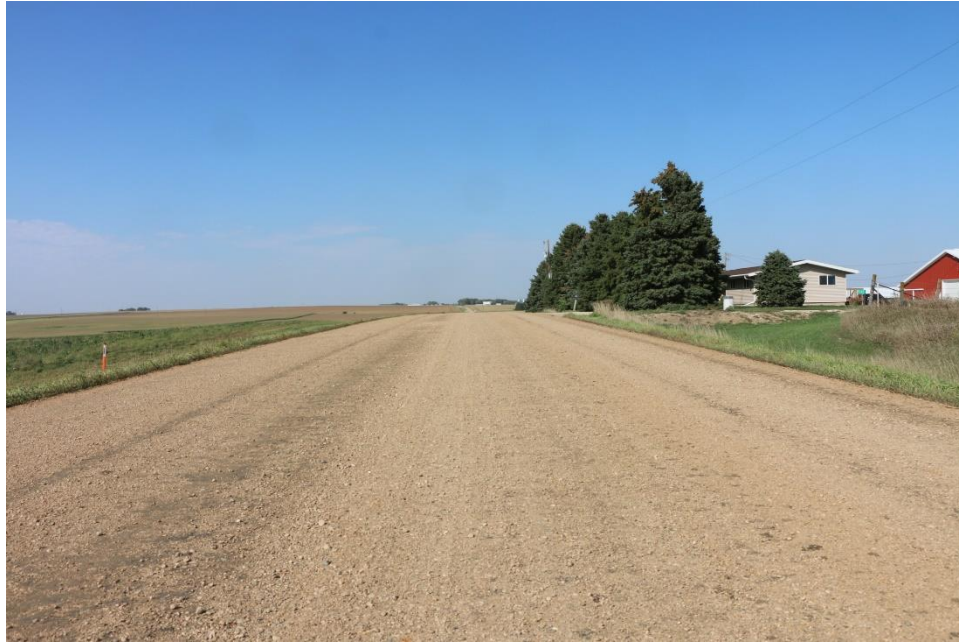
Figure 130. Appearance of Otta seal two days post construction showing dark areas near lane center
