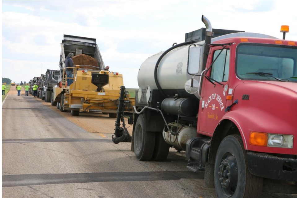
Figure 110. Binder, aggregate, and other construction equipment
