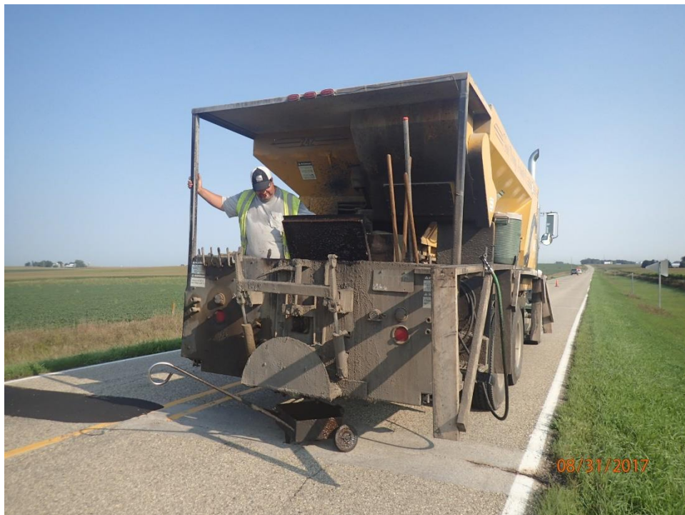
Figure 95. During the process of applying slurry seal
