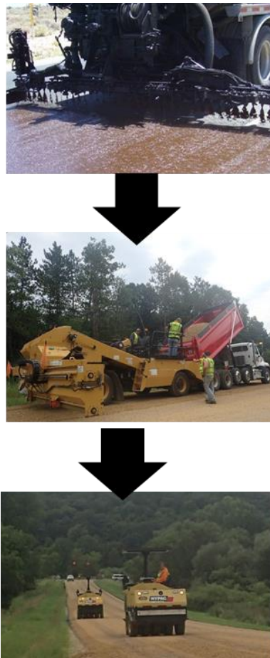
Figure 3. Surface treatment operation sequence
