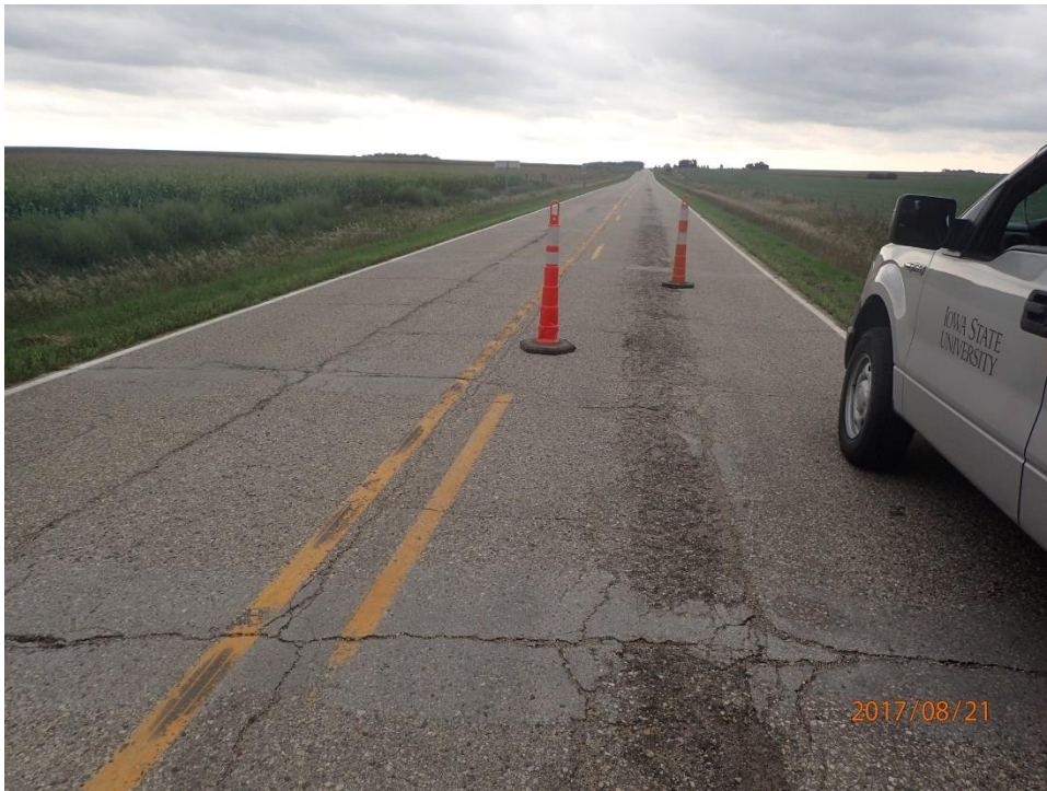
Figure 89. Longitudinal and transverse cracking present before implementing Otta seal in Cherokee, Iowa
