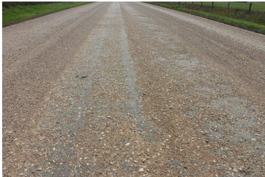
Figure 68. First layer appearance in whole sections: one week after application
