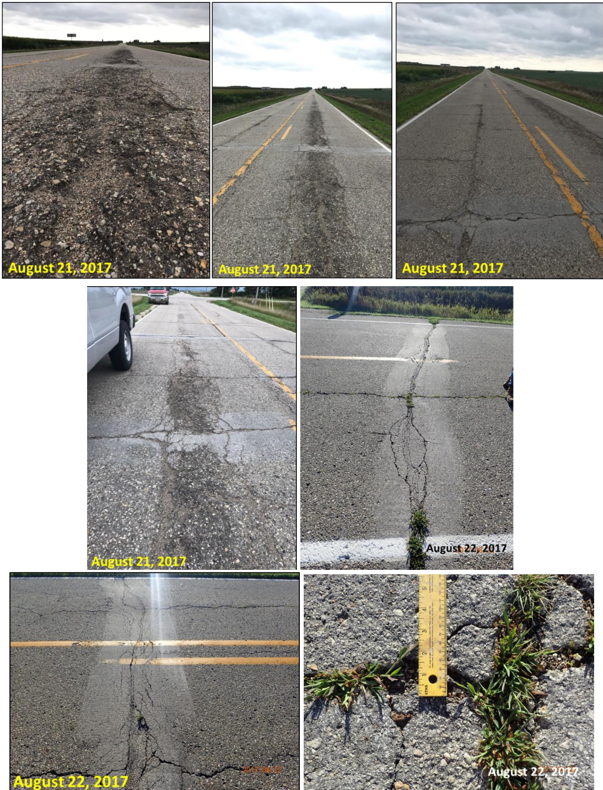
Figure 36. Various types of distresses observed on CR L-40 Otta seal project site prior to any surface treatment, August 21–22, 2017
