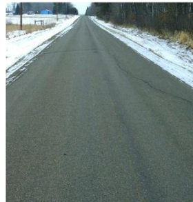
Otta Seal constructed 2001, Cass County CR171
