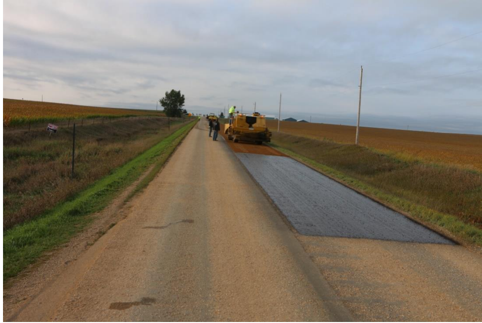
Figure 124. Aggregate application during second layer construction
