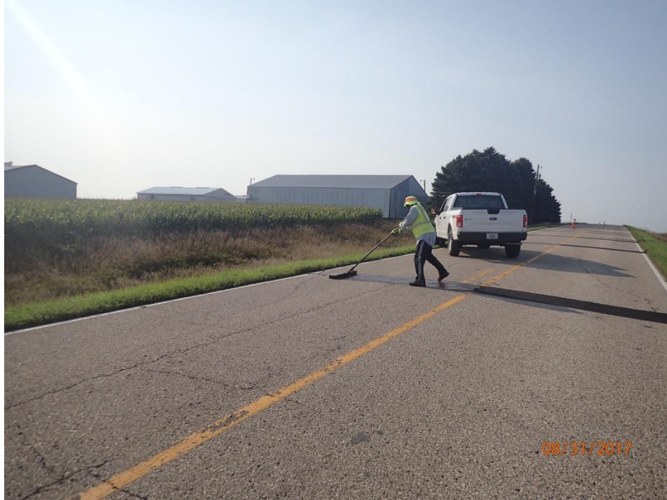
Figure 96. Applying slurry seal
