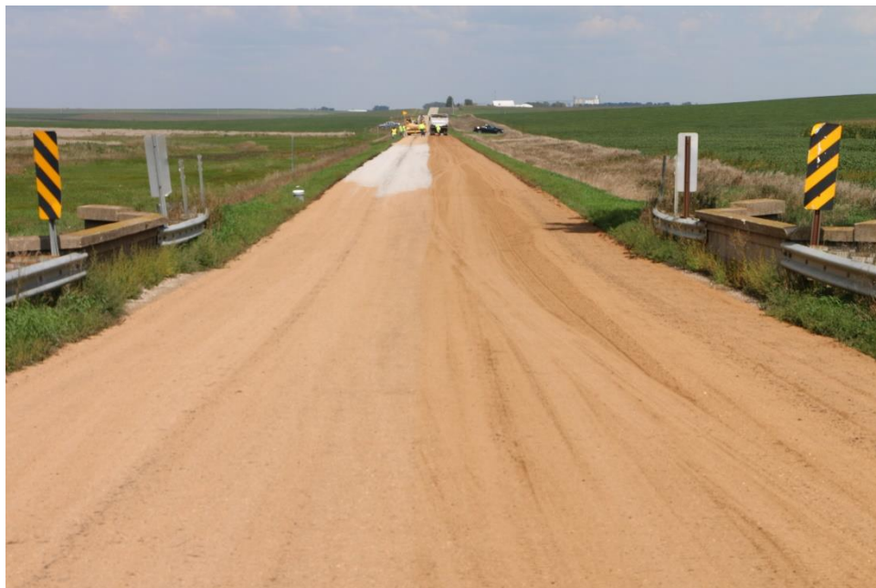
Figure 109. Otta seal first layer construction
