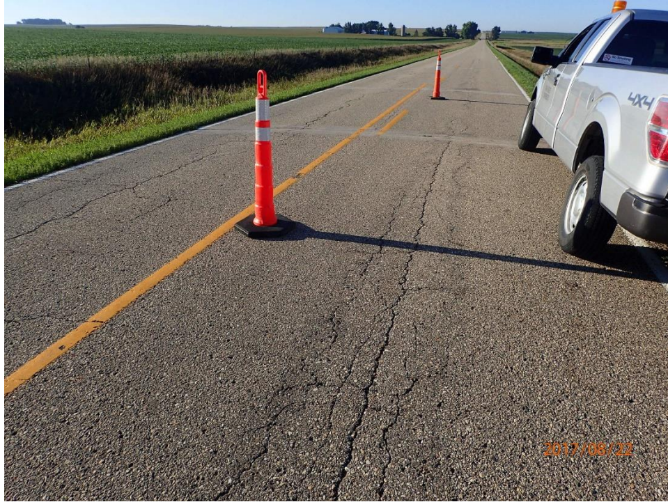
Figure 92. Existing longitudinal cracking
