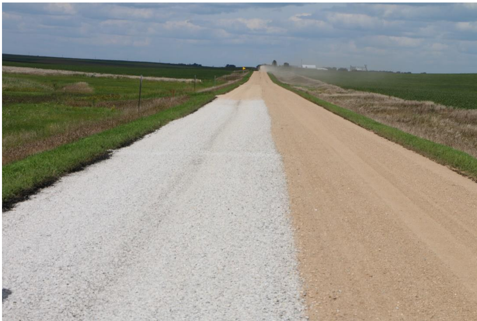
Figure 117. Appearance of Otta seal first layer after comparing test sections
