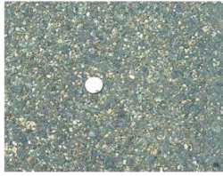
Otta Seal constructed 2001, Cass County CR171
