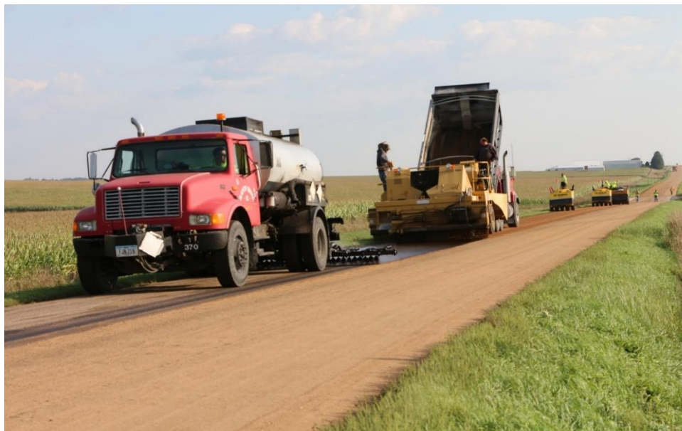
Figure 105. The complete processes of Otta seal construction
