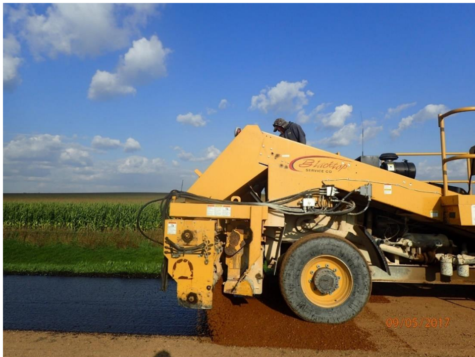
Figure 103. Aggregate application during the first layer construction
