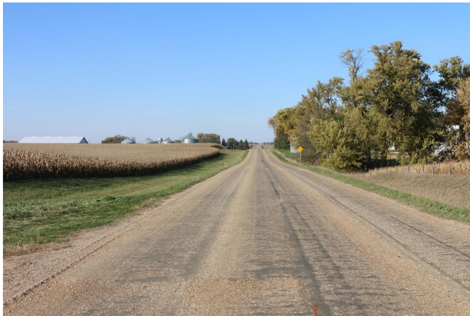
Figure 137. Appearance of Otta seal two weeks post construction, showing surface changed to darker color
