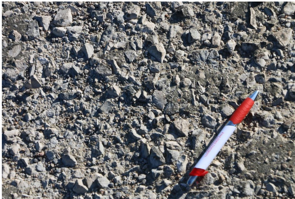
Figure 139. Appearance of Otta seal surface two weeks post construction of test section using limestone
