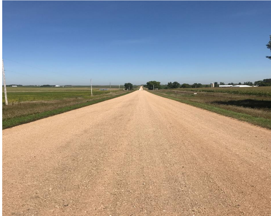
Figure 67. First layer appearance: three days after application
