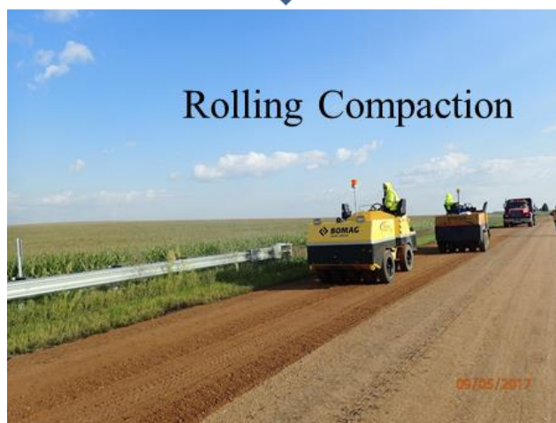
Figure 47. Three key steps during Otta seal construction
