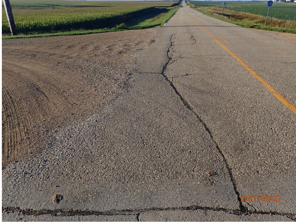
Figure 94. Existing cracking at intersection area
