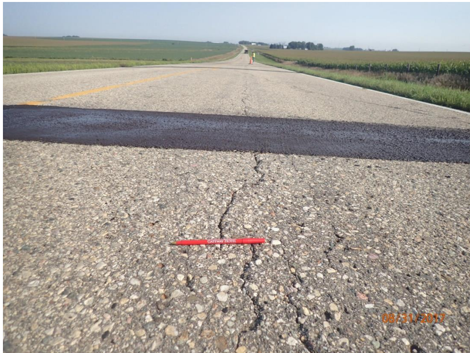
Figure 99. Slurry seal in curing
