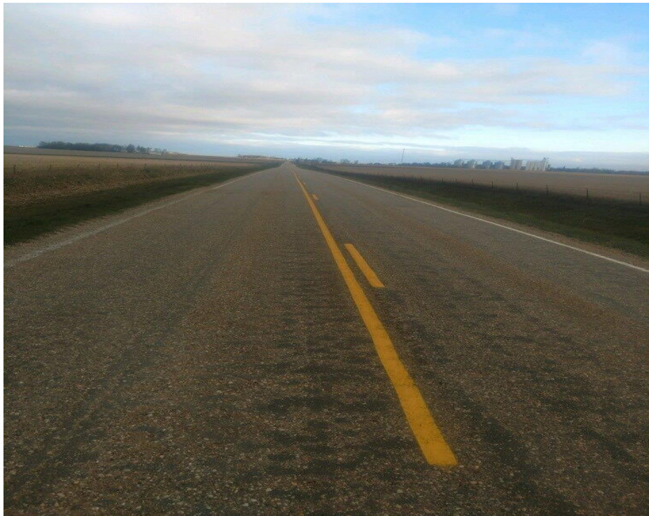
Figure 143. Appearance of Otta seal surface two months post construction, showing that surface continued to change to darker color
