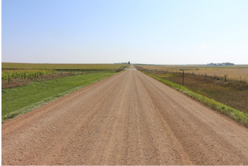
Figure 69. Second layer appearance in whole sections: two days after application
