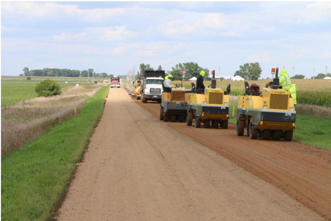
Figure 113. Compaction after applying binder and aggregates
