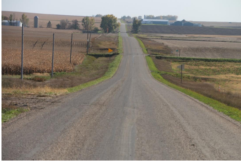
Figure 138. Appearance of Otta seal two weeks post construction, with lane center a lighter color than other areas
