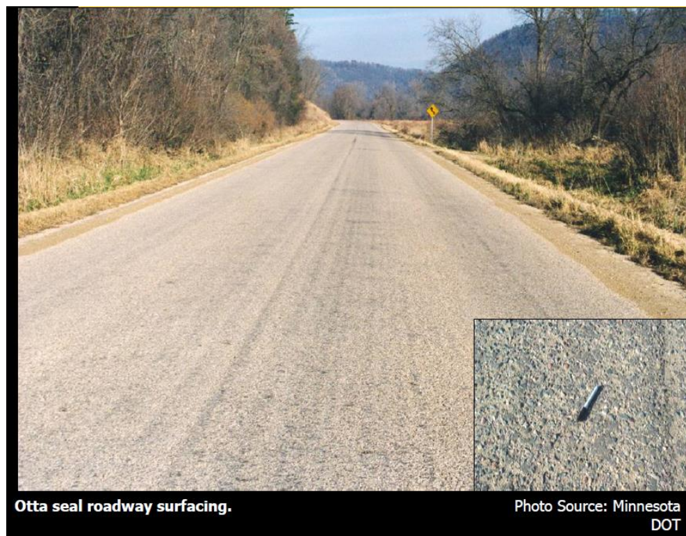
Figure 8. Otta seal surfacing
