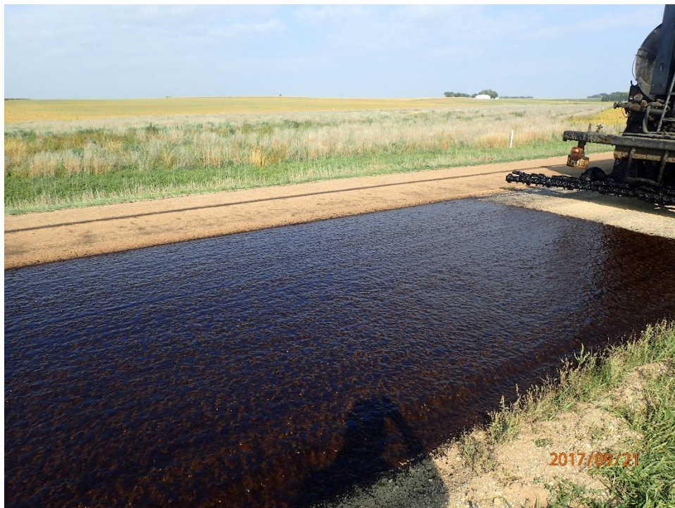
Figure 123. Binder spraying during second layer construction
