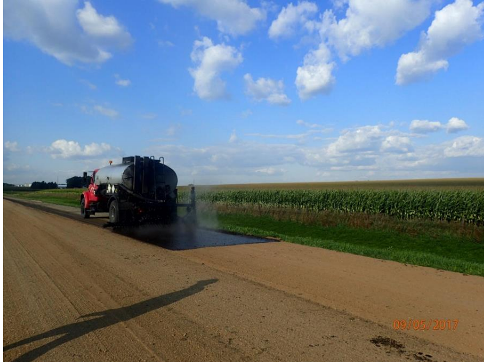
Figure 102. Binder application during the first layer construction
