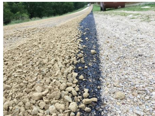
Figure 22. Aggregate used for Otta seal on CR 116, Winona County, Minnesota
