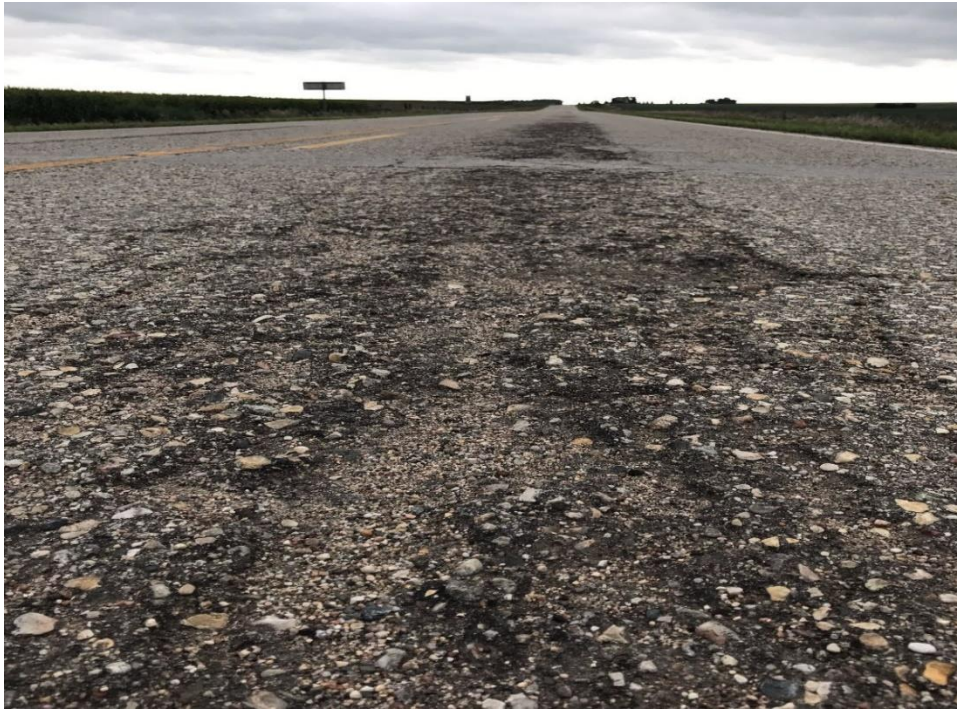
Figure 88. Condition of the road surface before implementing Otta seal in Cherokee, Iowa
