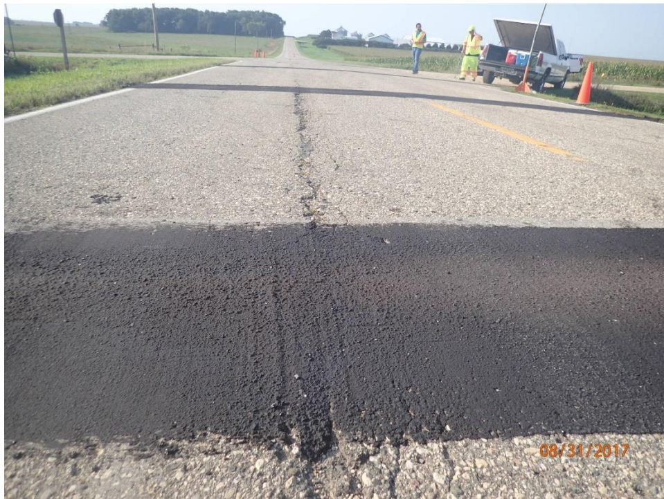
Figure 101. Slurry sealed cracking area
