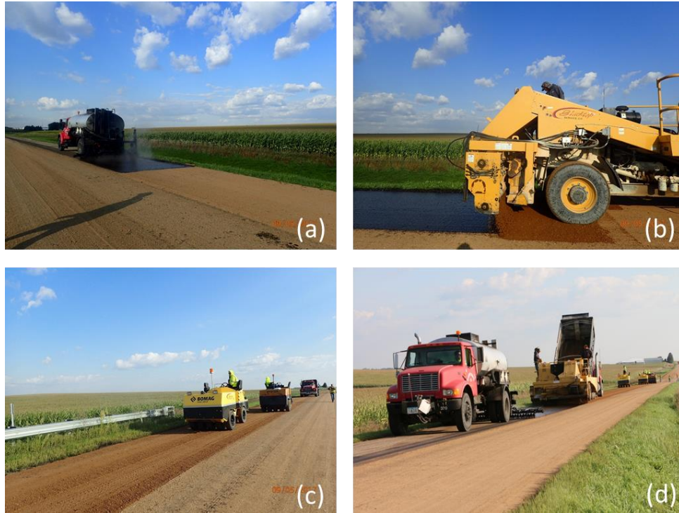
Figure 55. Construction of the second Otta seal layer: (a) binder spraying, (b) aggregate application, (c) rolling compaction, and (d) the complete process
