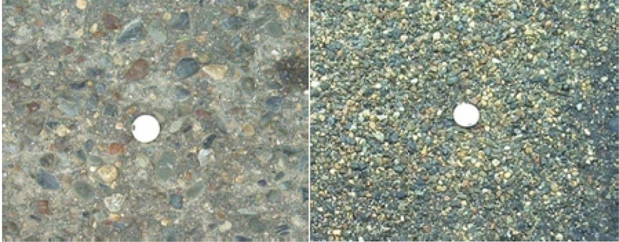
Figure 1. Otta seal roadway surfacing
