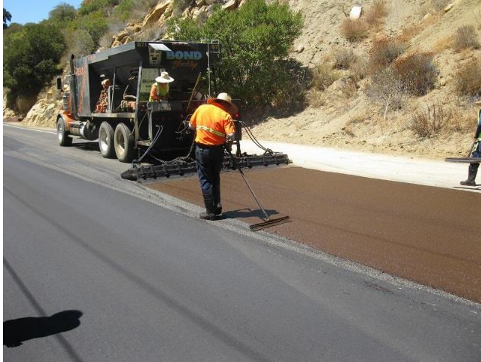
Figure 5. Microsurfacing application
