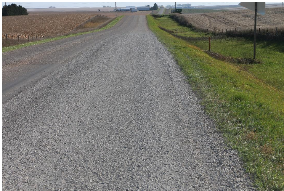
Figure 135. Appearance of Otta seal two weeks post construction showing one test section
