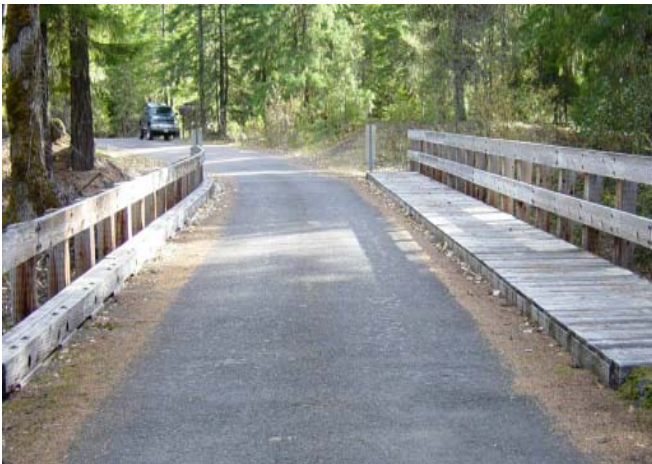
Figure 10. Lost Creek Bridge wearing surface in 2002.
