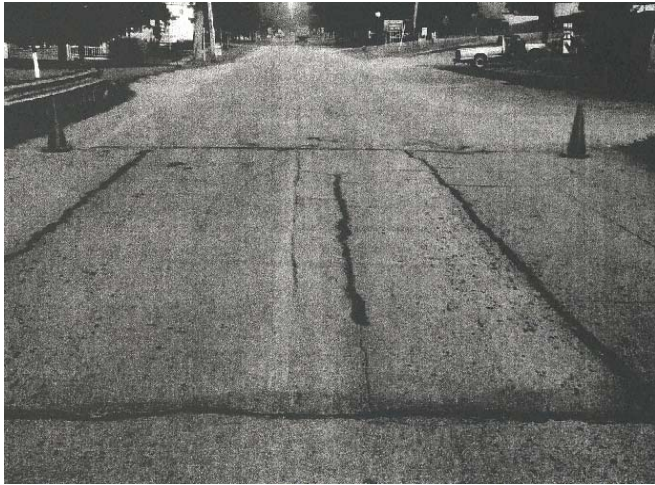
Figure 26. East Main Street Bridge wearing surface in 2000.
