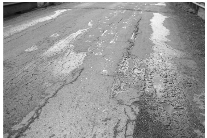
Figure 20. Bolivar Bridge wearing surface in 2003.
