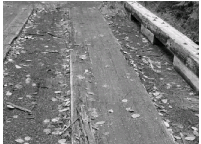
a. Longitudinal planks on wheel lines.
