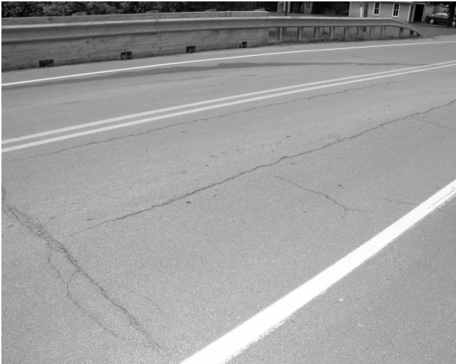
Figure 13. East Main St. Bridge wearing surface in 2003.
