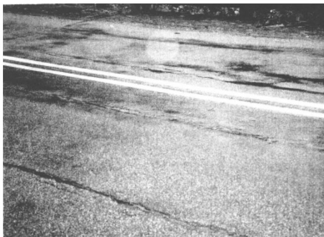
Figure 16. Angelica Creek Bridge wearing surface in 1998.
