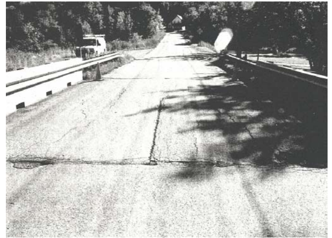
Figure 27. Bolivar Bridge wearing surface in 2000.
