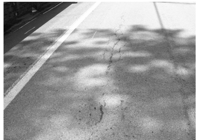
Figure 22. Scio Bridge wearing surface in 2003.
