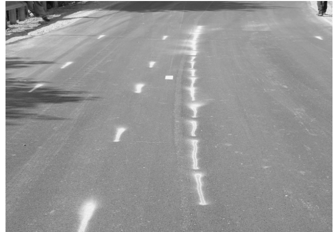
Figure 17. Angelica Creek wearing surface in 2003.
