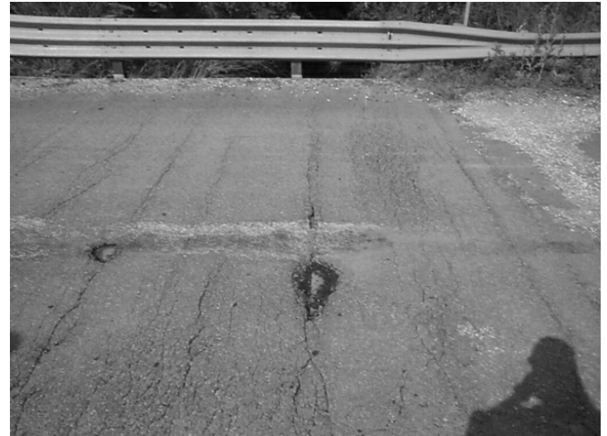
Figure 11. Chambers Co. Bridge wearing surface in 2003.
