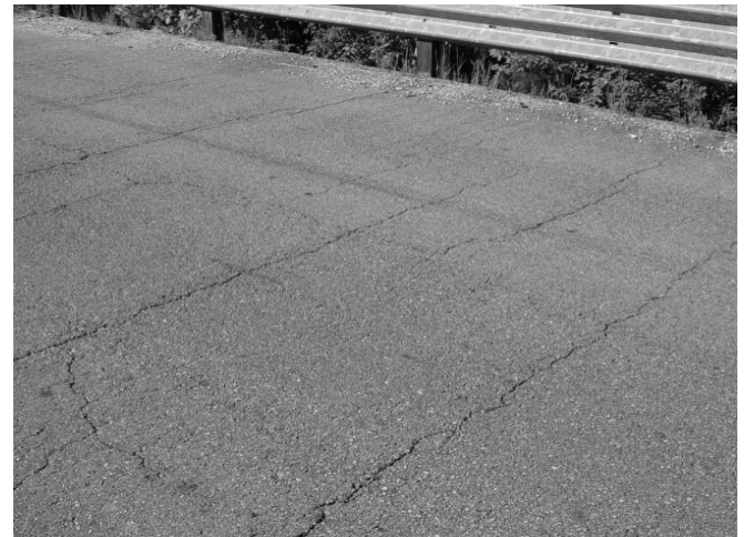
Figure 6. Russellville Bridge wearing surface in 2003.
