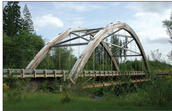
Figure 1. Three-pinned glulam arch timber bridge located in Mason County, Washington.
