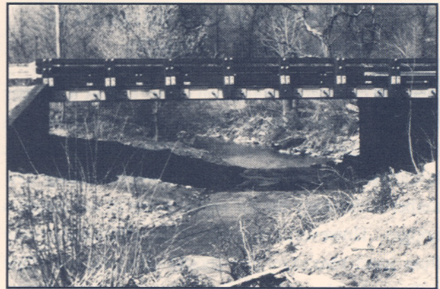
Leon A. Shook Memorial Bridge
