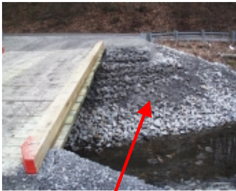
Gabion Basket Abutments
