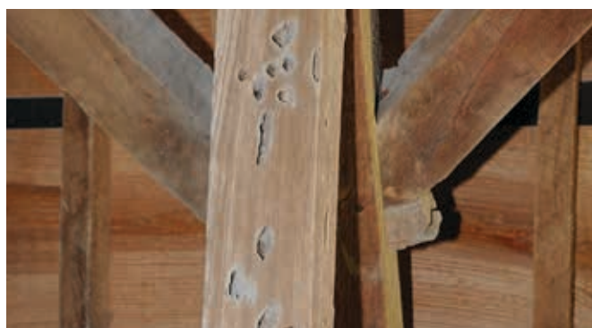
Figure 10.2—Example of insect damage.
