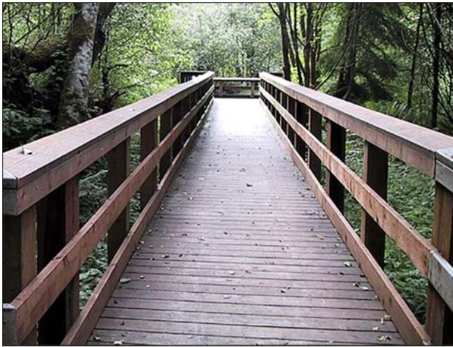
Figure 7—This CDDC-treated boardwalk is being evaluated for leaching and environmental accumulation of copper.
