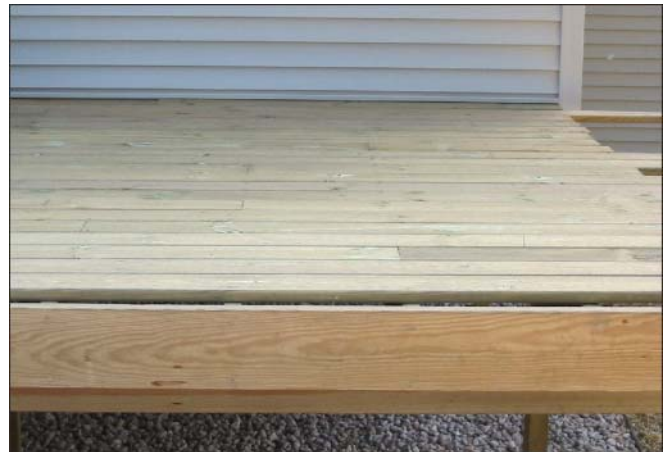
Figure 5—Supports treated with CCA and decking treated with copper azole (CBA-A).
