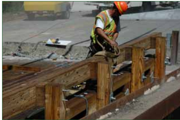
Assembling a crash-tested guide railing on a glued laminated longitudinal deck.
