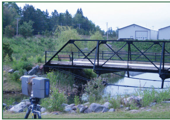
3D laser scanning technologies are used to document as-built conditions of historic structures, such as this 1905 bridge built by A.Y. Bayne & Co. It is currently located on the grounds of Minnesota’s St. Louis County Richard H. Hansen Public Works and Transportation Complex.
