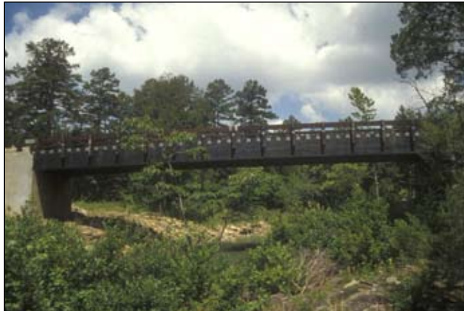
Big Shoal Creek glulam bridge located in Arkansas' Ozark National Forest.
