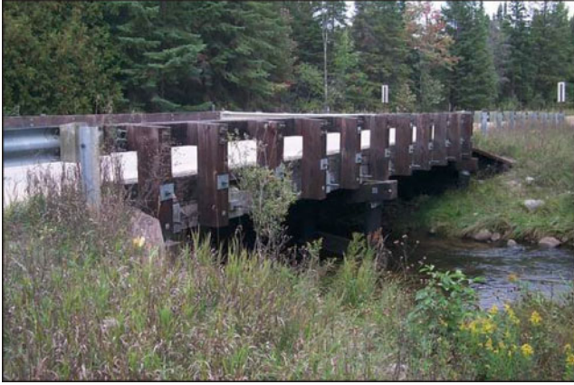
Figure 8—Old Vanderbilt bridge in Otsego County.
