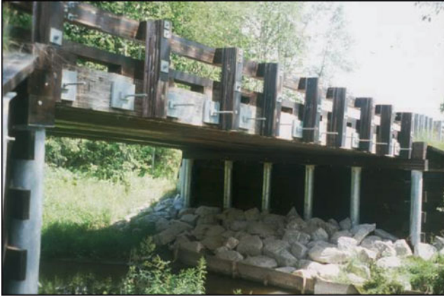
Figure 7—Barlow bridge in Alcona County.
