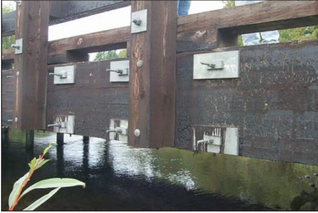
Figure 5—Cameron bridge in Crawford County.
