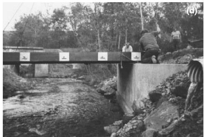
Figure 11—Completed deck placed on abutments: (a) bar tensioning completed, (b) deck lifted from temporary abutments by small crane, (c) deck positioned over Hoffman Run, (d) superstructure placed on abutments.
