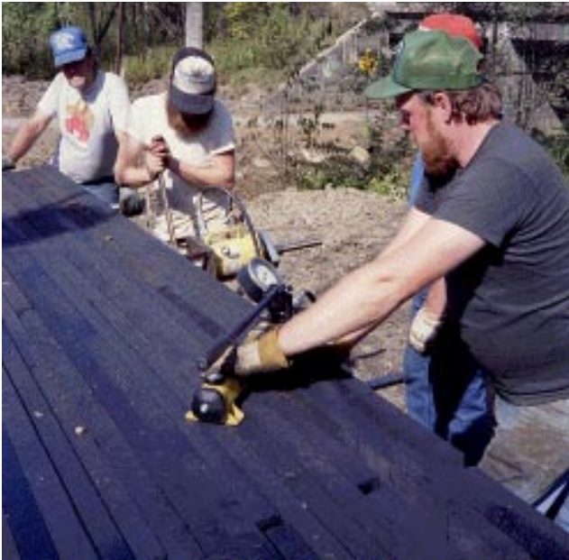
Figure 10—Stressing bars were tensioned with a single hydraulic jack.
