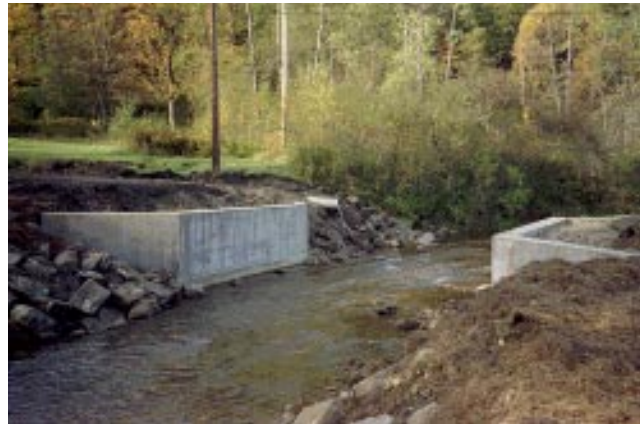
Figure 6—Completed concrete abutments and wingwalls for the Hoffman Run bridge.
