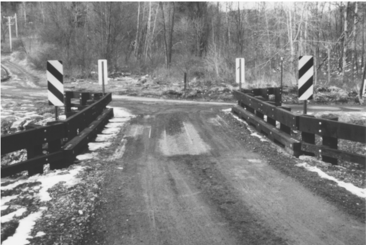
Figure 12—Completed Hoffman Run bridge: (top) side view; (bottom) end view.
