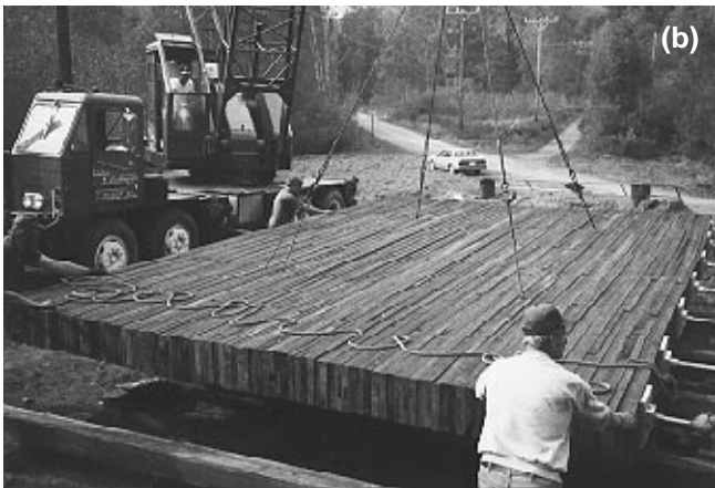
Figure 11—Completed deck placed on abutments: (a) bar tensioning completed, (b) deck lifted from temporary abutments by small crane, (c) deck positioned over Hoffman Run, (d) superstructure placed on abutments.
