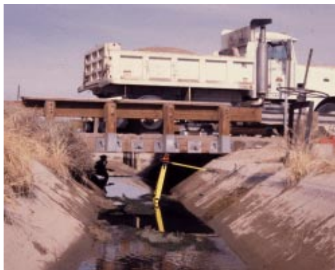
Figure 14—Transverse load positions 3 (top) and 5 (bottom) used for load test 2.
