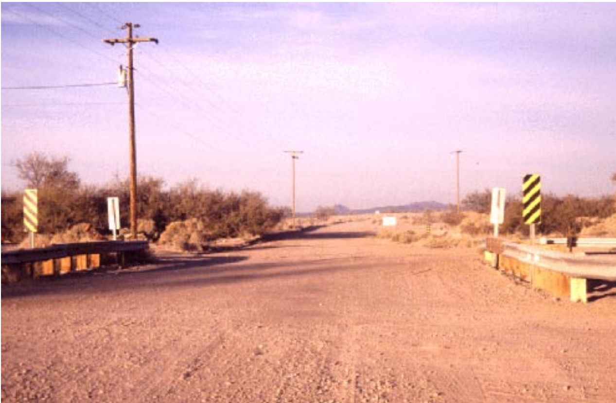
Figure 8—Completed Mohawk Canal bridge: side view (top), end view (bottom).
