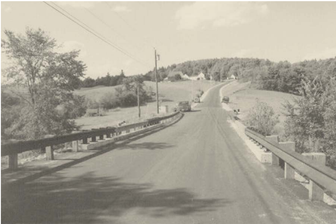
Figure 14—Completed Gray bridge.
