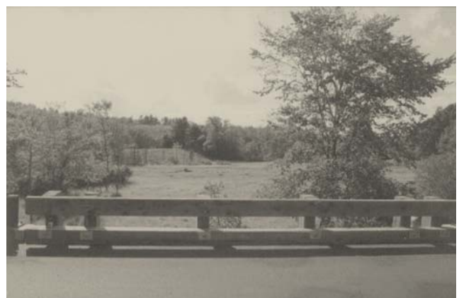
Figure 13—Gray bridge following installation of the post and rail system.
