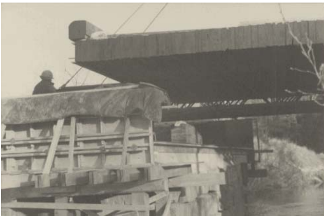
Figure 11—The deck was moved by crane over the span.
