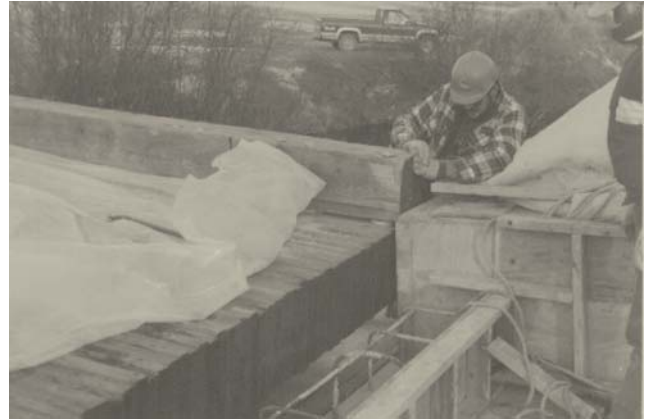
Figure 12—The deck was placed by crane onto the abutments.
