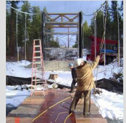
Towers, Cables, and Hangers
