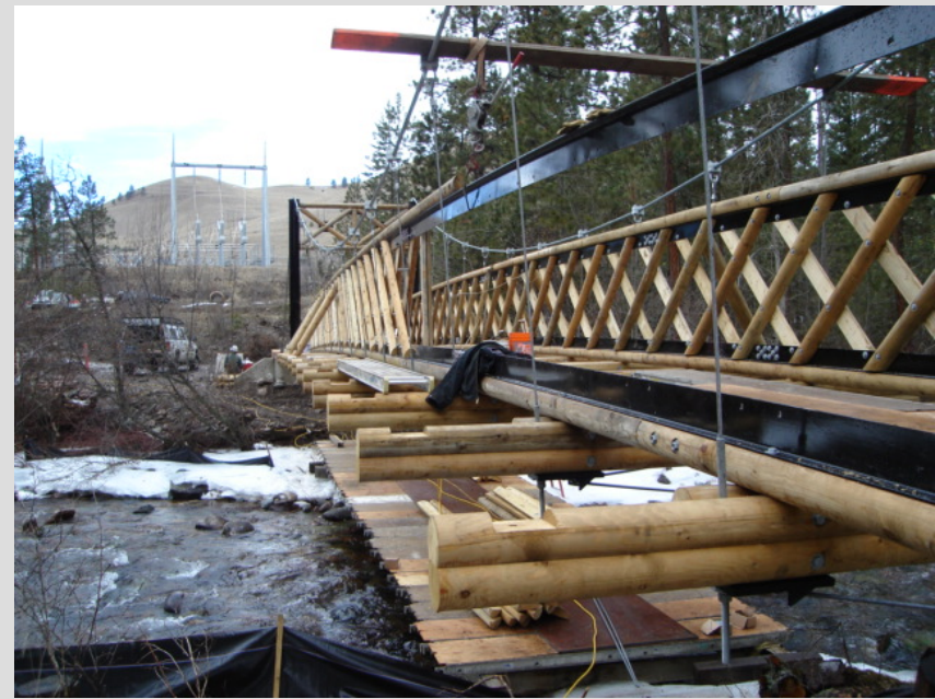
Lattice Stiffening Truss
