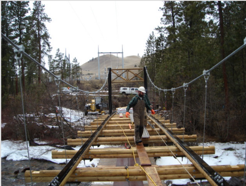
Transverse Floor Beams
