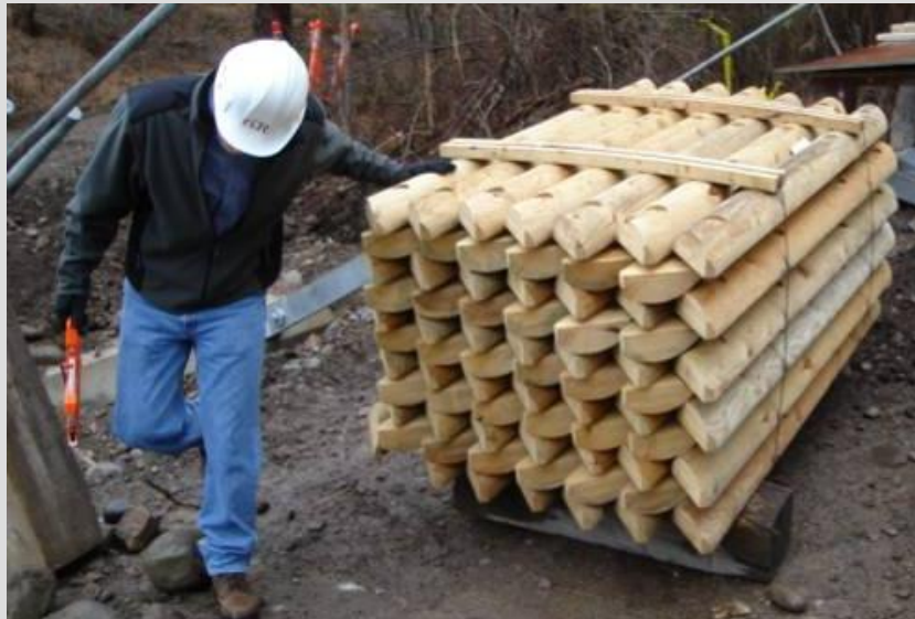
Lattice Truss Diagonals
