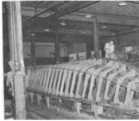
Figure 68.— Construction of V-bottom boat with frames joined at keel, chine, and deck with glued and bolted plywood gussets.
