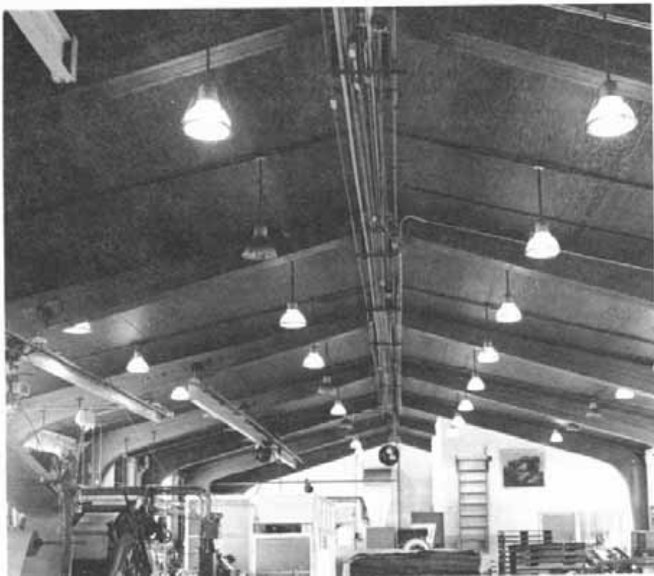
Figure 16.— Building erected in 1935 with casein glued-laminated arches. It is currently used for packaging research at the Forest Products Laboratory. Arches are in excellent condition.
