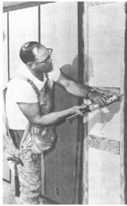
Figure 75.— Application of mastic adhesive to studs for bonding wall panels.
