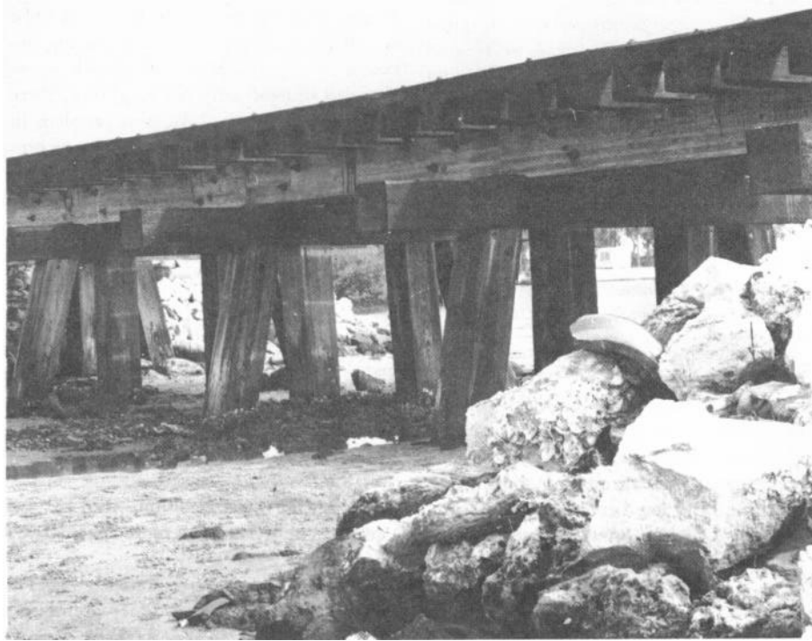
Figure 100.—Laminated southern pine stringers in 60-foot, open-deck trestle on Atlantic Coastline Railroad south of Palmetto, Fla. Lumber used in stringers was treated with fluor-chrome-arsenate-phenol (Wolman salt) before gluing. The stringers on the opposite side of the trestle were glued from creosote-treated southern pine.
