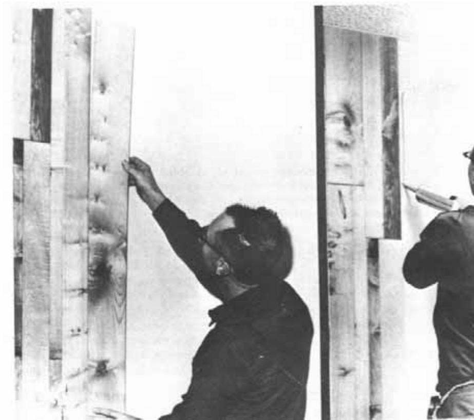
Figure 76.— Application of press-dried lumber paneling to plastered wall with mastic-type adhesive. left: Fitting panel to the adjacent one. Right: Applying adhesive to wall with caulking gun.
