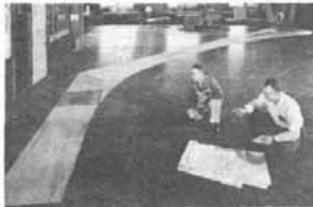
Figure 47.— Laying out template for an arch on mold-loft floor.
