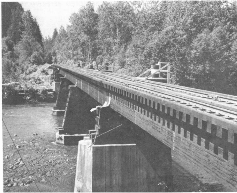
Figure 99. — Bridge on logging railroad near Longview, Wash., built with laminated stringers pressure treated with creosote-oil mixture before erection.
