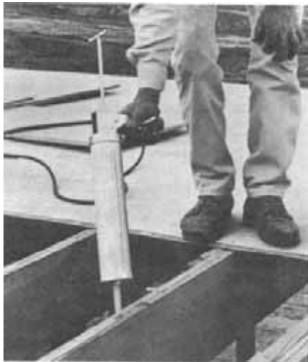
Figure 74.— Application of mastic adhesive for bonding plywood to joists. The plywood is also nailed, which furnishes gluing pressure.
