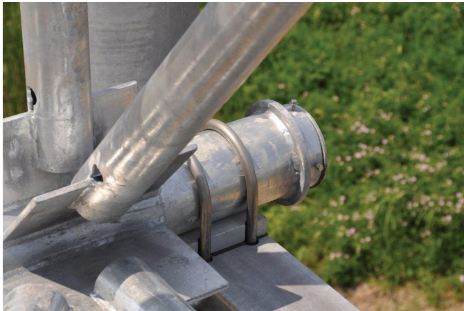
Type-A U-bolt connection
