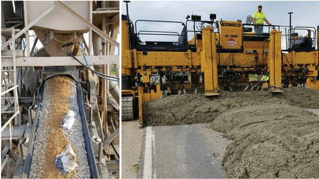
*Mitchell County test section construction showing addition of fibers at the batch plant and overlay paving*
