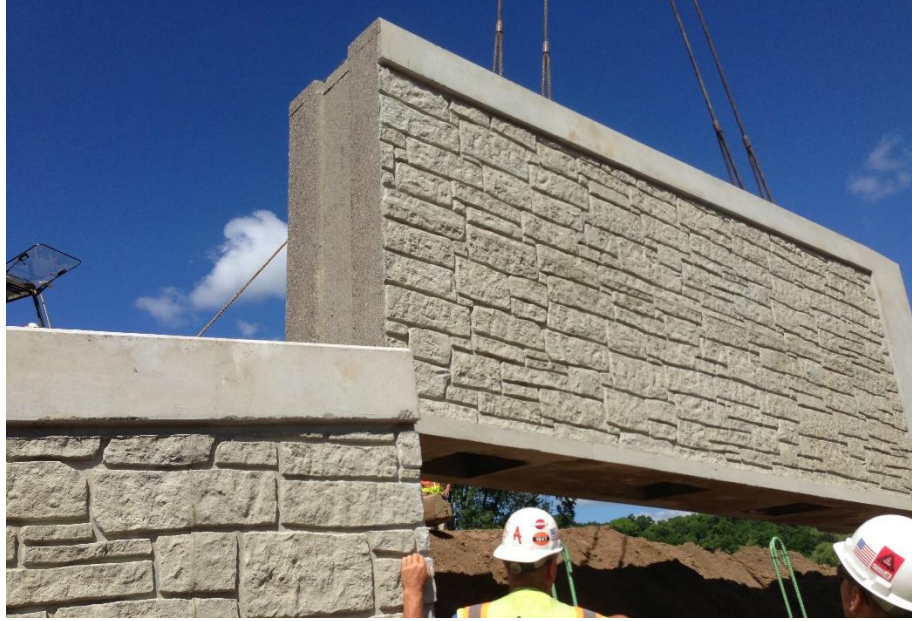
Figure 10. Precast abutment setting over piles with projecting, hooked, reinforcing steel bars
