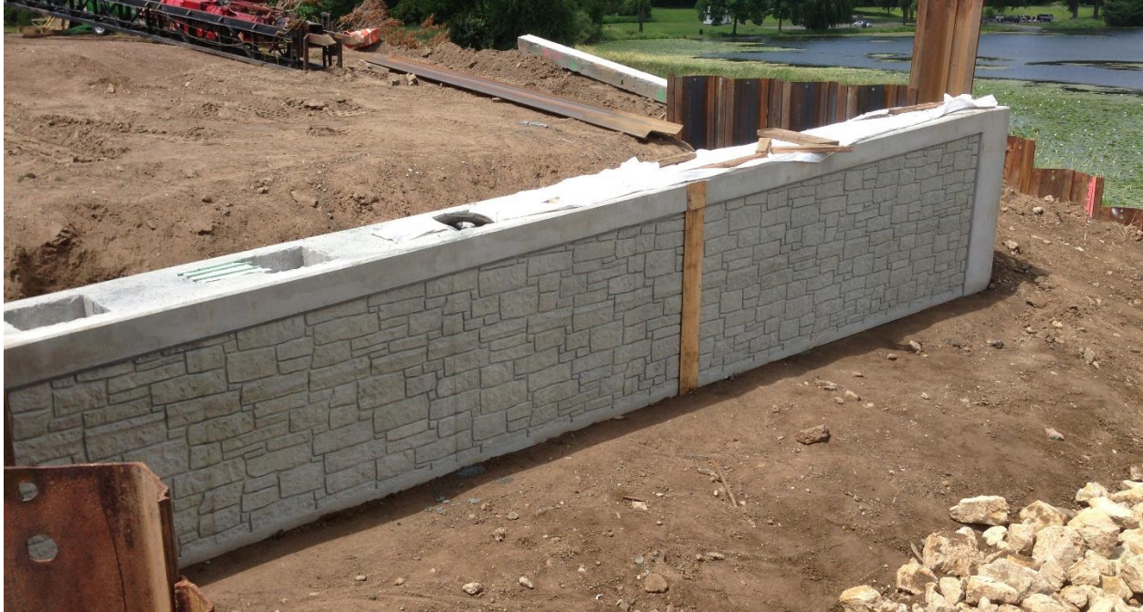
Figure 15. Precast abutment set showing pile grout pockets with wingwalls that consisted of a permanent sheetpile wall with a CIP facing and top coping
