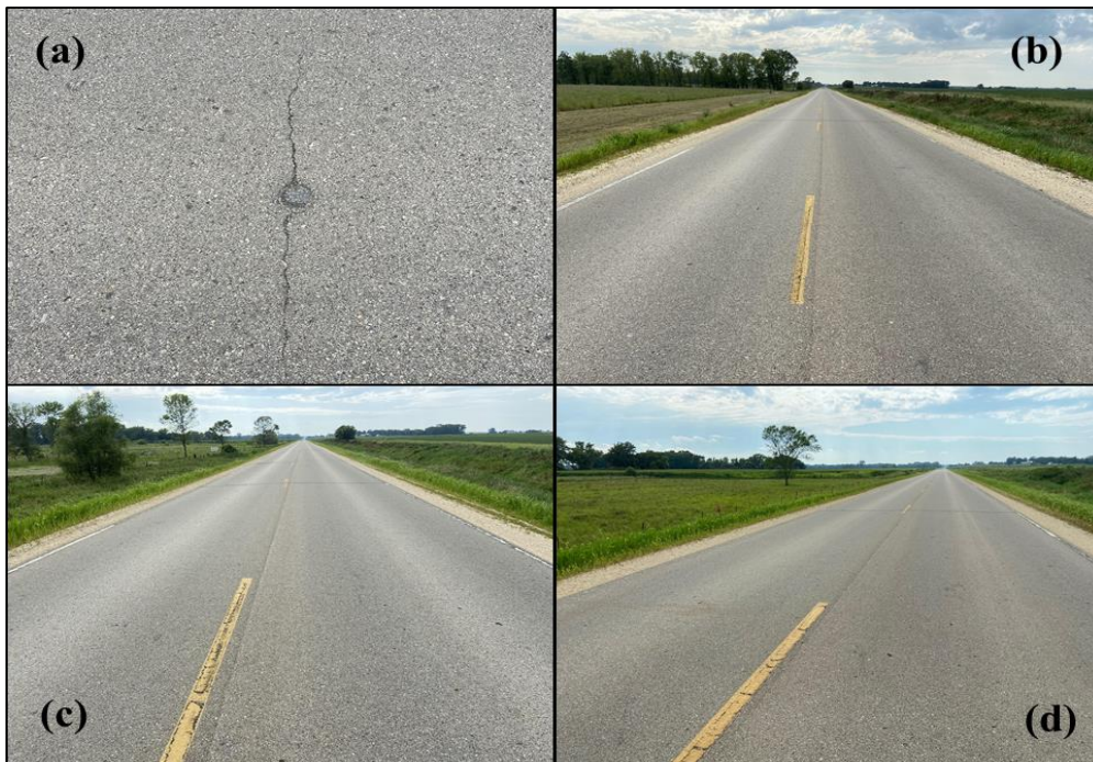
Figure 22. Field survey on August 9, 2020: (a) control section, (b) treated section No. 1 (0.03 gal/yd 2 ), (c) treated section No. 2 (0.025 gal/yd 2 ), and (d) treated section No.3 (0.02 gal/yd 2 )
