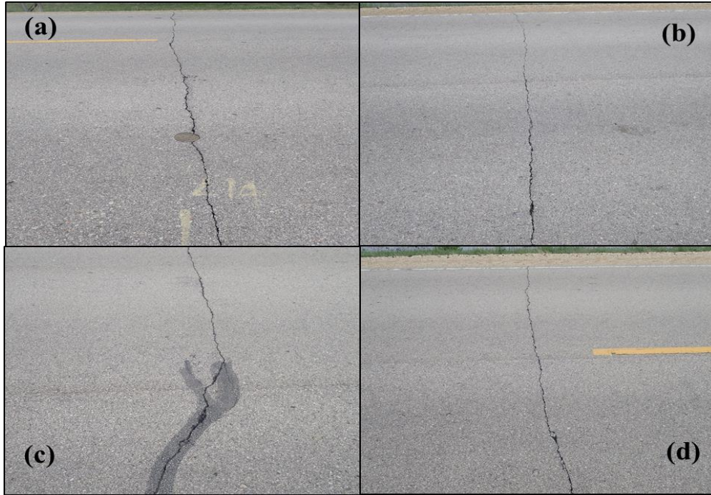
Figure 21. Field survey on May 11, 2019: (a) control section, (b) treated section No. 1 (0.03 gal/yd 2 ), (c) treated section No. 2 (0.025 gal/yd 2 ), and (d) treated section No.3 (0.02 gal/yd 2 )
