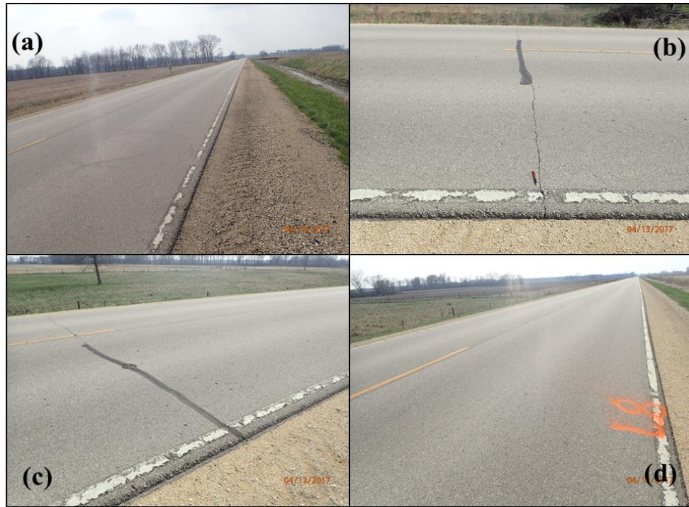
Figure 18. Field survey on April 13, 2017: (a) control section, (b) treated section No. 1 (0.03 gal/yd 2 ), (c) treated section No. 2 (0.025 gal/yd 2 ), and (d) treated section No.3 (0.02 gal/yd 2 )
