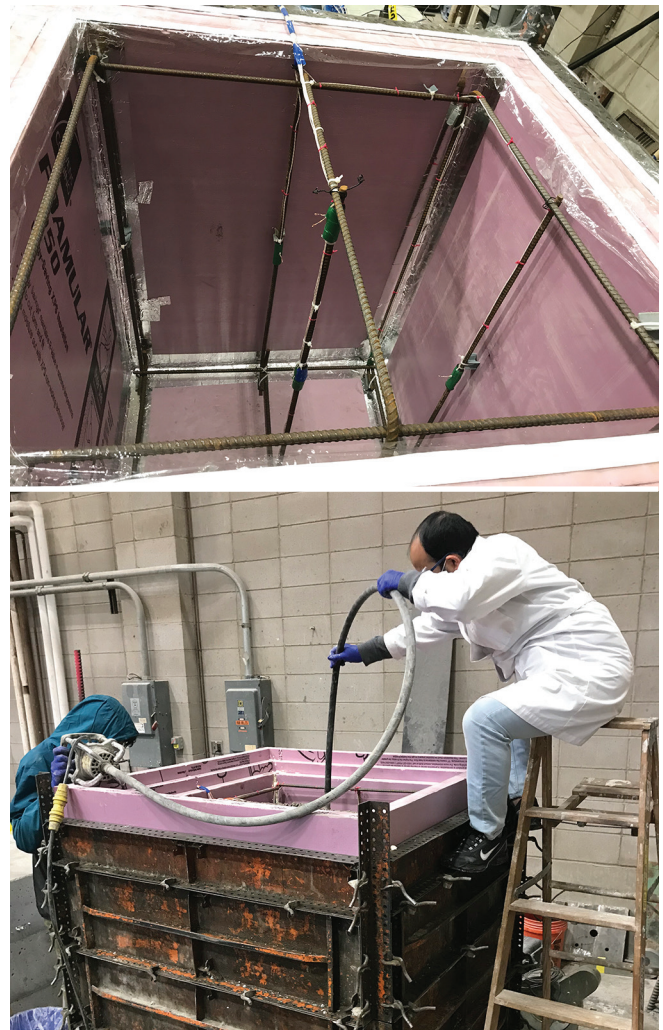
Large concrete block casting
