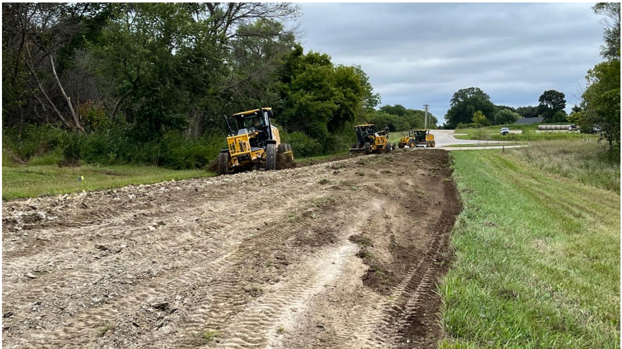
Figure 37. Incorporation of material from both ditches to build up road elevation
