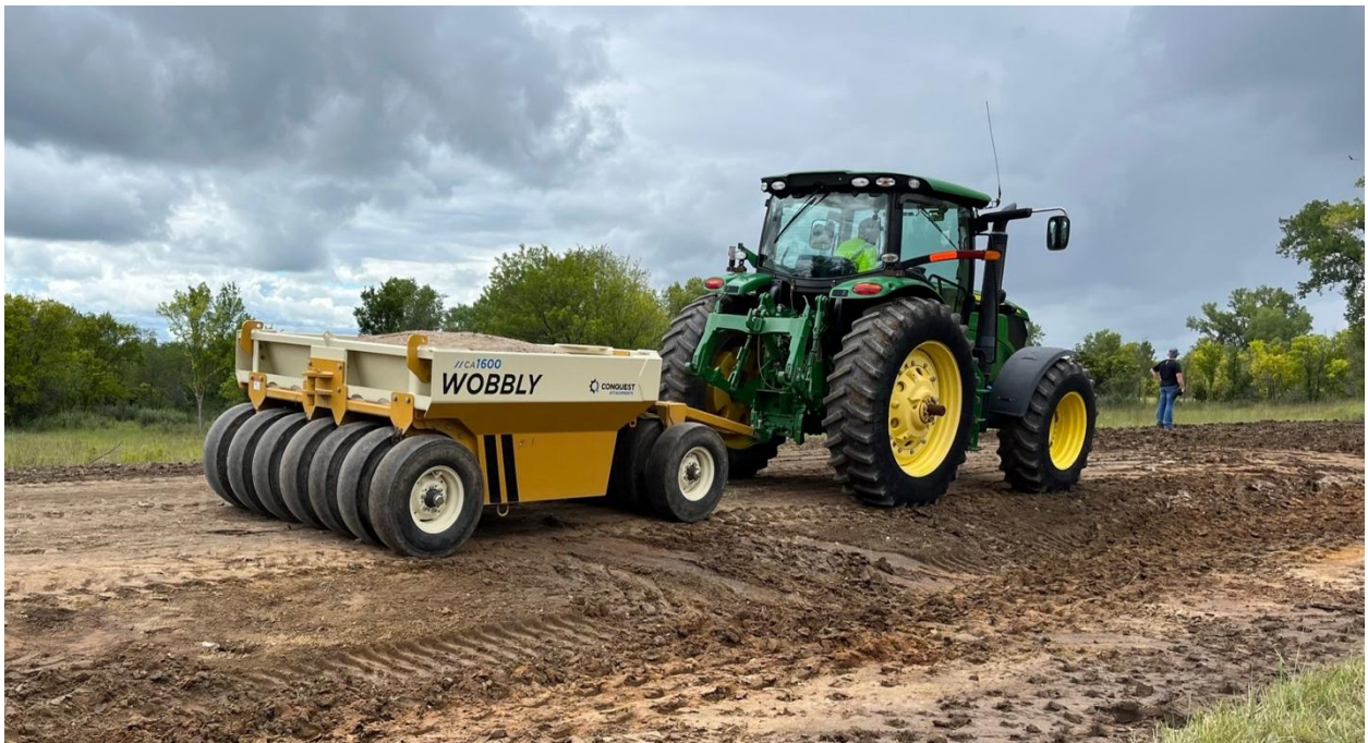
Figure 39. Smooth-tired compactor used for test section construction
