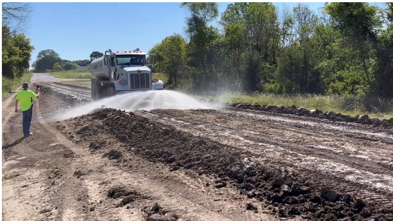
Figure 47. Spraying liquid stabilizer on Section 1
