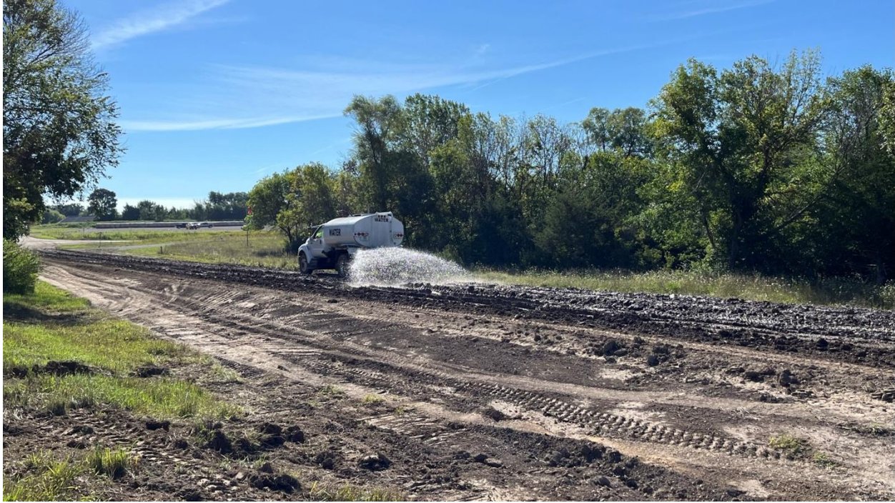
Figure 45. Spraying water on surfaces of Sections 1 and 2 on Day 3 prior to spraying stabilizer
