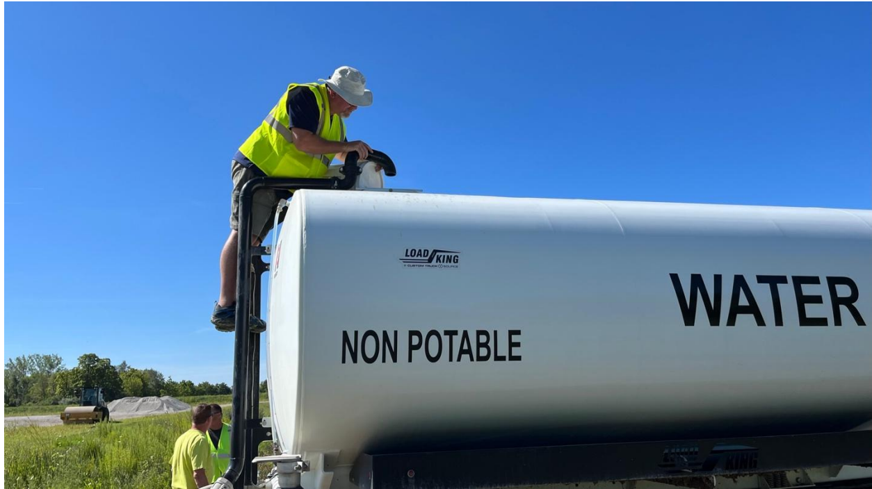
Figure 46. Adding liquid stabilizer to nearly full 2,200 gal water truck
