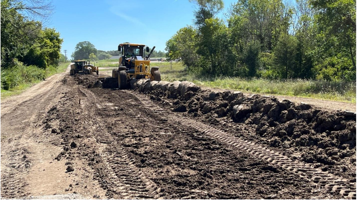
Figure 50. Mixing stabilizer into top 6 in. of subgrade in Sections 1 and 2
