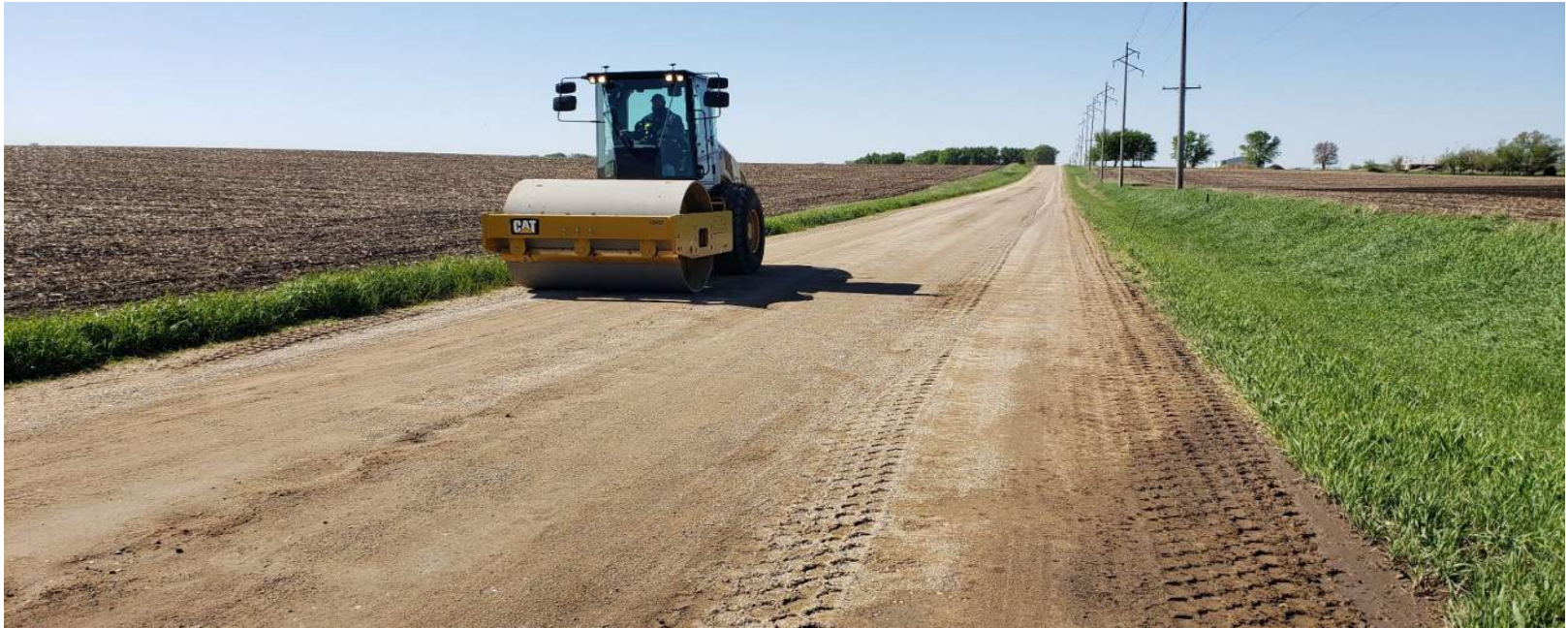
Figure 1. Picture of the COMP-Score RT enabled roller mapping (Picture taken on 05/27/22 at 10:04 am)
