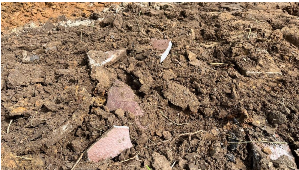
Figure 35. Example of construction debris encountered in existing roadbed materials
