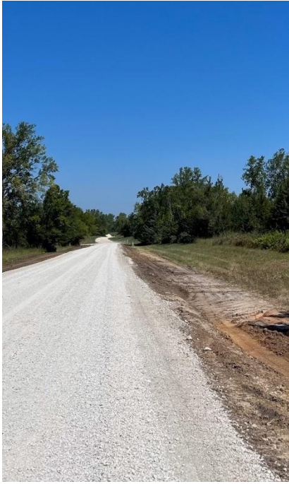
End of construction, Summer 2023
