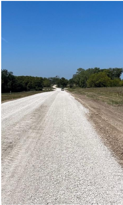
End of construction, Summer 2023
