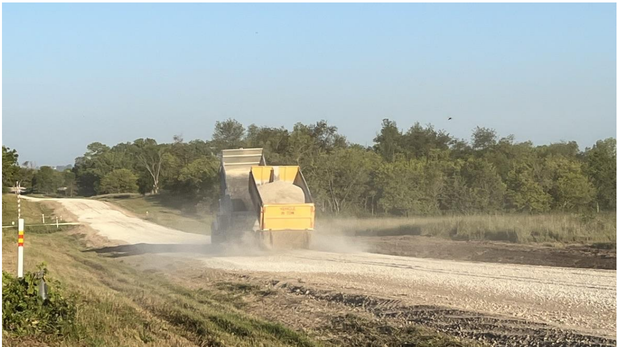
Figure 54. Start of spreading of surfacing aggregate on Sections 1 and 2 on Day 4 (August 17, 2023)
