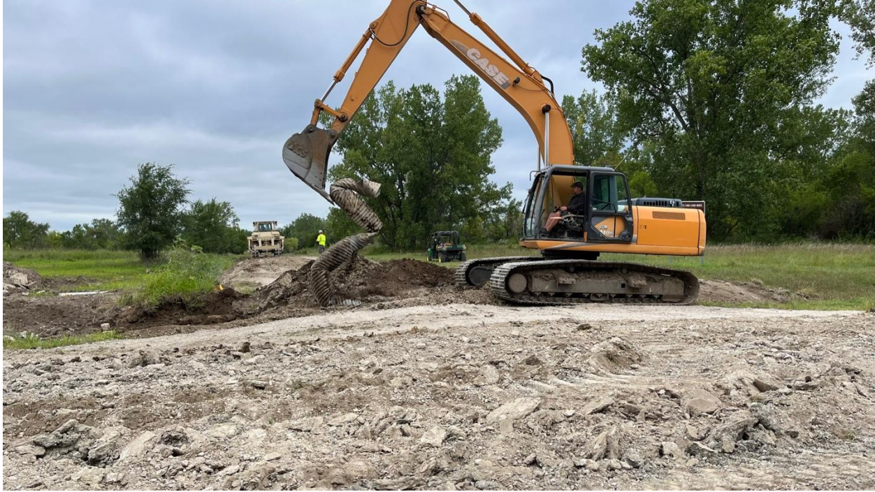
Figure 41. Removal of old corrugated culvert pipe for replacement
