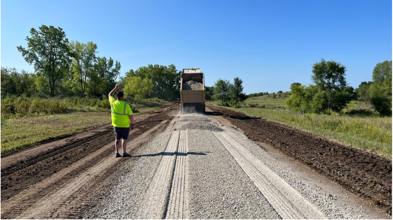
Figure 44. Spreading Class A roadstone on surface of Section 4 on Day 2 (August 15, 2023)
