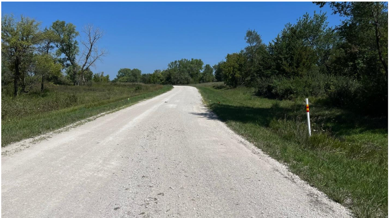
Figure 60. Surface of the untouched control Section 5 at end of construction
