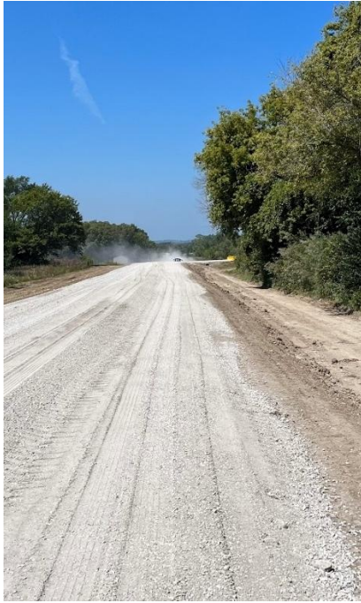
End of construction, Summer 2023
