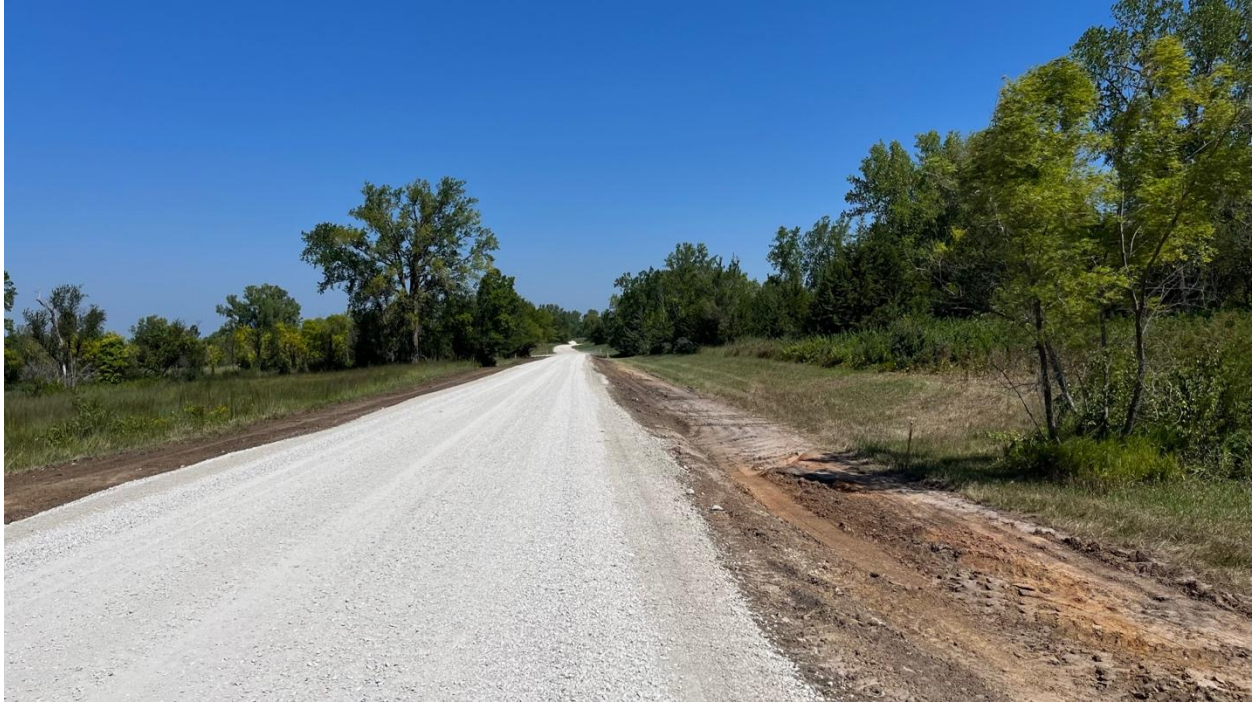
Figure 59. Surface of Section 4 at end of construction
