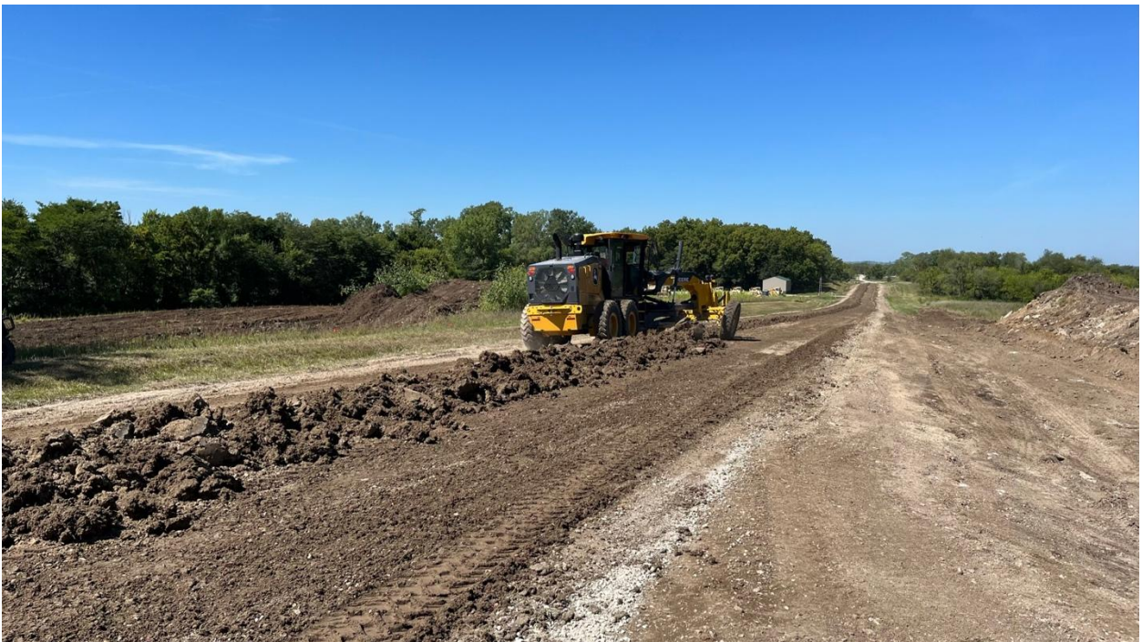
Figure 51. Mixing stabilizer into top 6 in. of subgrade in Sections 1 and 2
