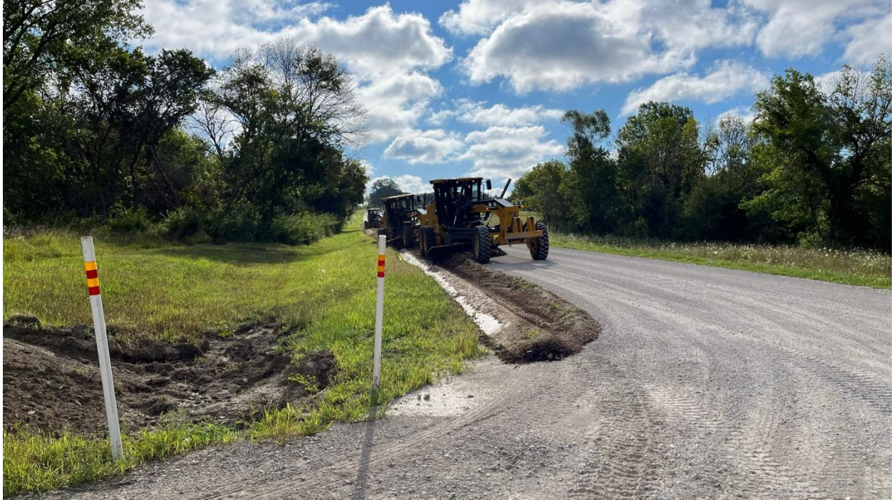
Figure 36. Initial excavation of ditch material in Section 1
