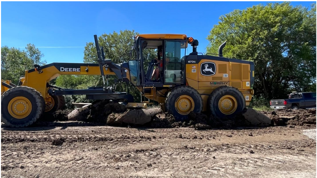
Figure 49. Mixing stabilizer into top 6 in. of subgrade in Sections 1 and 2
