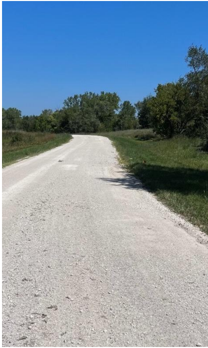
End of construction, Summer 2023
