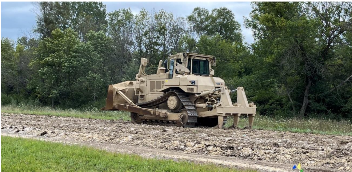
Figure 34. Ripping existing roadway materials
