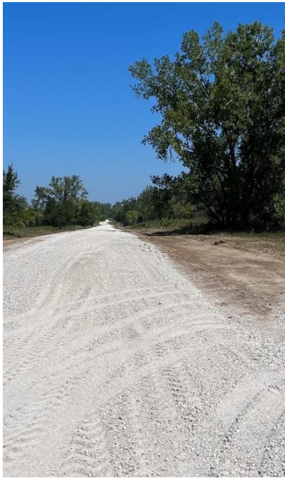
End of construction, Summer 2023
