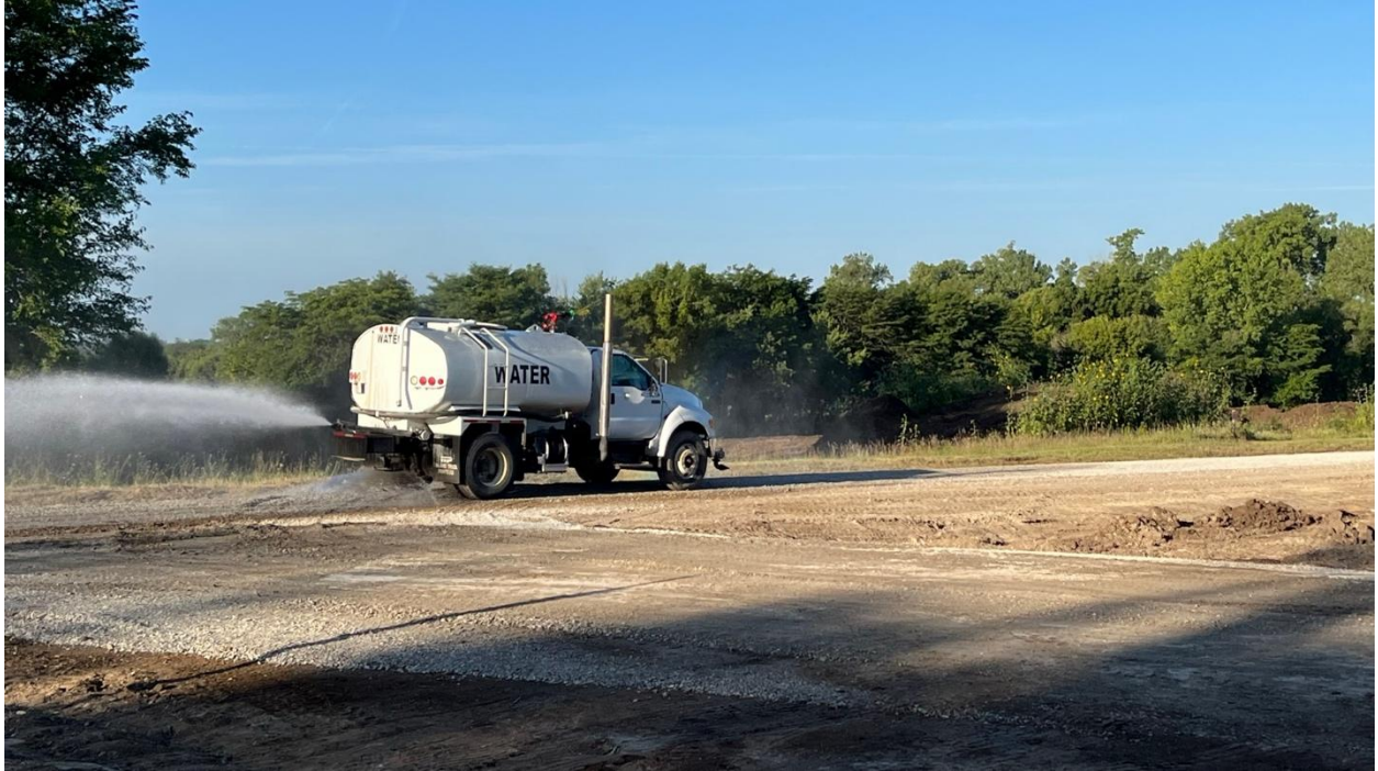
Figure 55. Additional water being sprayed for compaction of Class A roadstone surface
