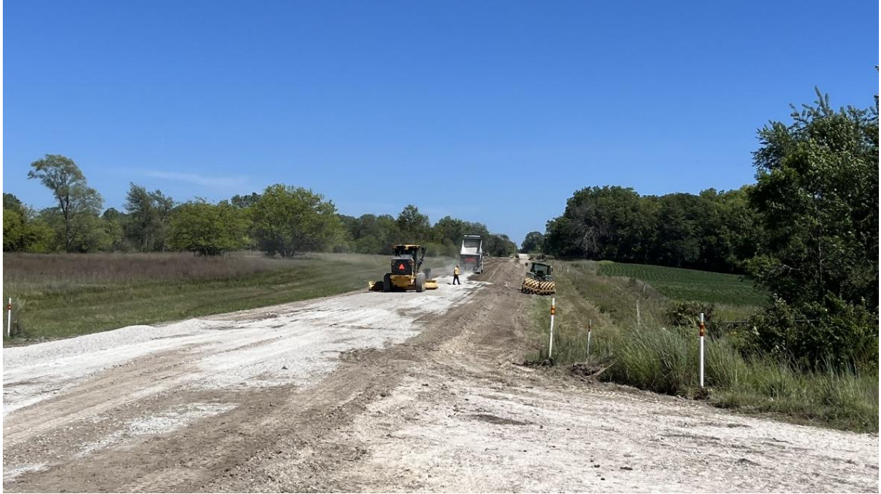
Figure 53. Spreading of light roadstone cover to leave on road overnight
