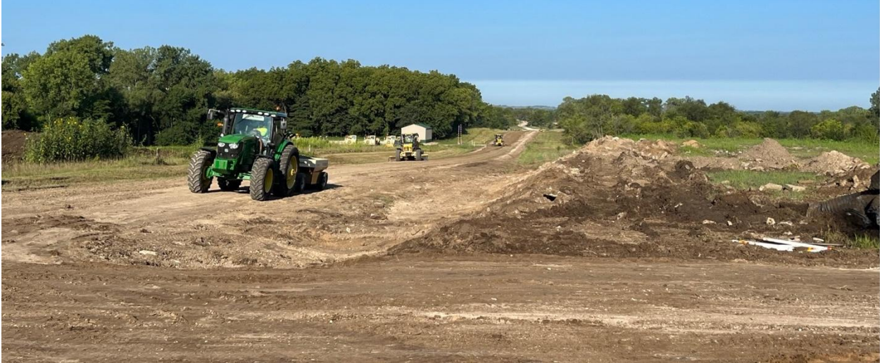
Figure 42. Continued shaping and compaction of reconstructed road profile on Day 2
