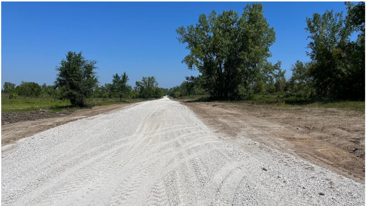
Figure 58. Surface of Section 3 at end of construction
