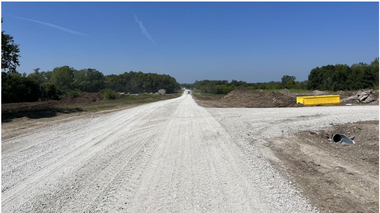
Figure 56. Surface of Section 1 at end of construction
