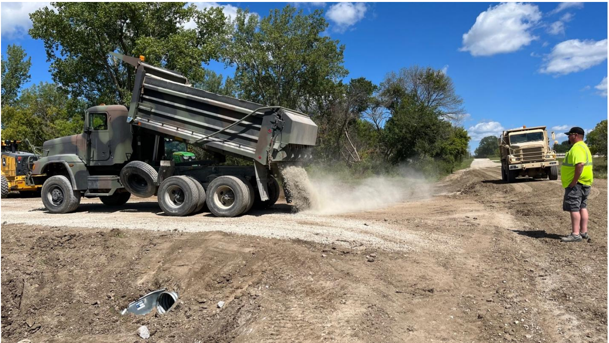
Figure 43. Spreading Class A roadstone on surface of Section 3 on Day 2 (August 15, 2023)
