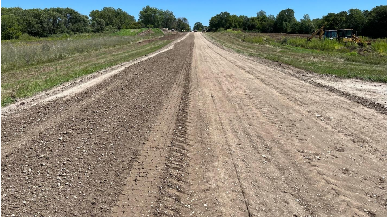
Figure 52. Perma-Zyme treated subgrade in Section 1 before (left) and after (right) first compaction pass of smooth-tired roller
