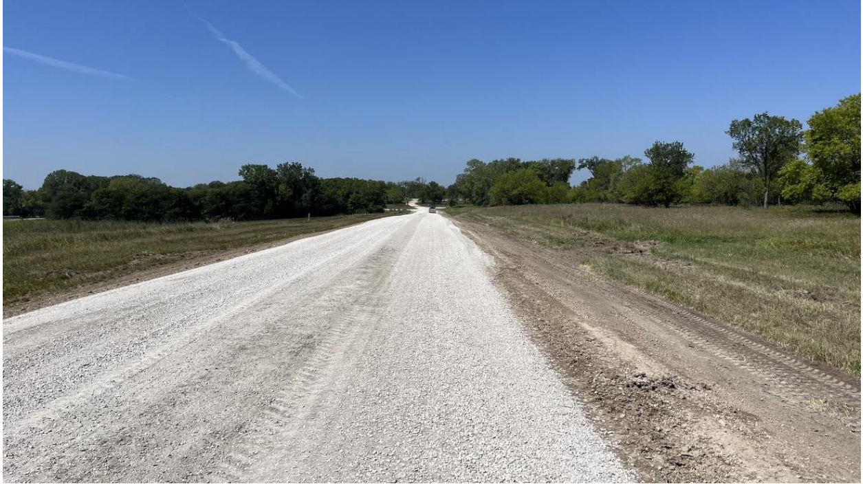
Figure 57. Surface of Section 2 at end of construction
