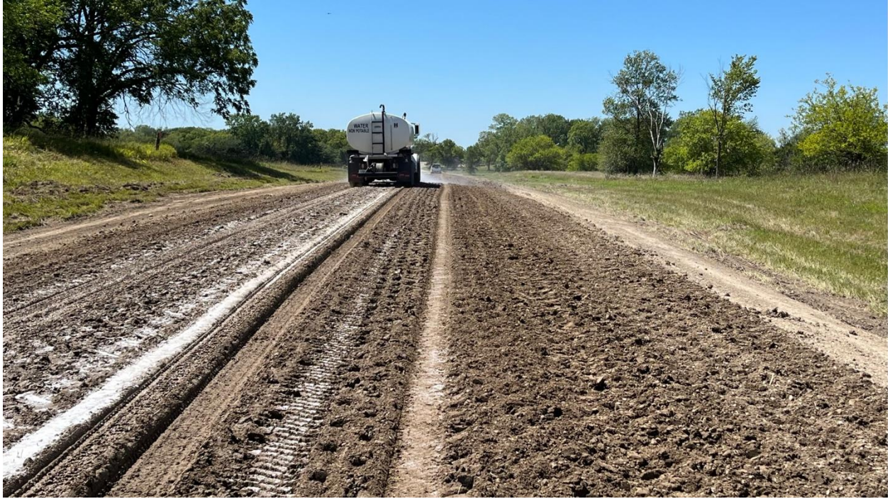
Figure 48. Surface of Section 2 during spraying of stabilizer
