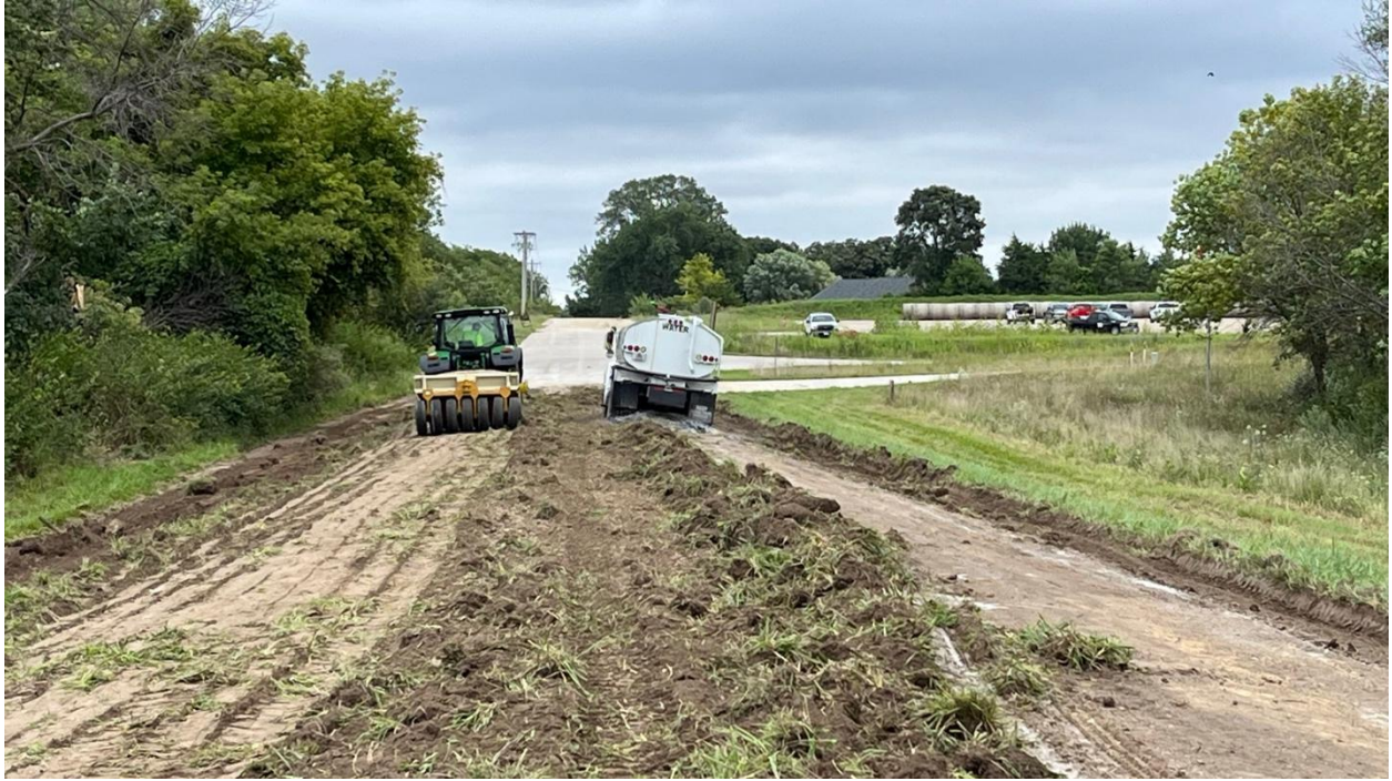
Figure 38. Application of water and compaction during reconstruction of roadway profile
